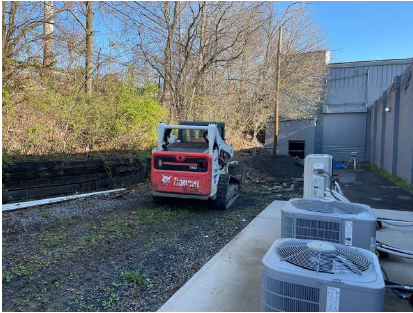
Bobcat loading the soils from stockpile
