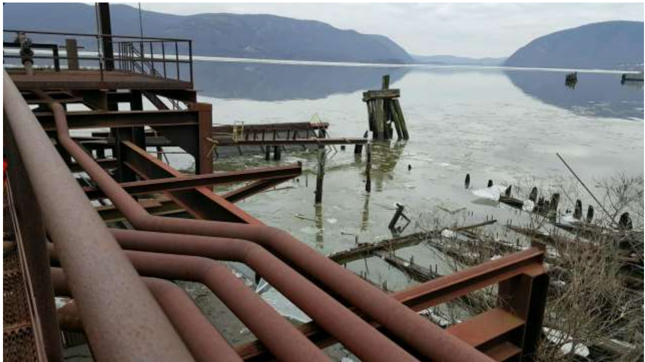
Photograph 2: Remaining onsite piping at the location of the former fuel dock.
