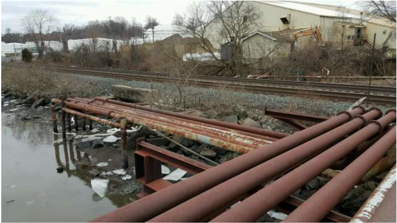
Photograph 3: Remaining onsite piping at the location of the former fuel dock.
