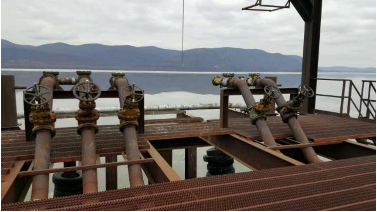
Photograph 4: Remaining onsite piping at the location of the former fuel dock.
