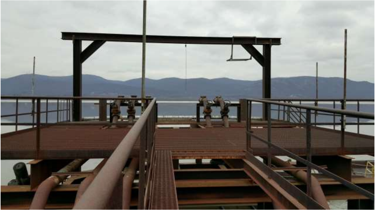
Photograph 6: Remaining onsite piping at the location of the former fuel dock.
