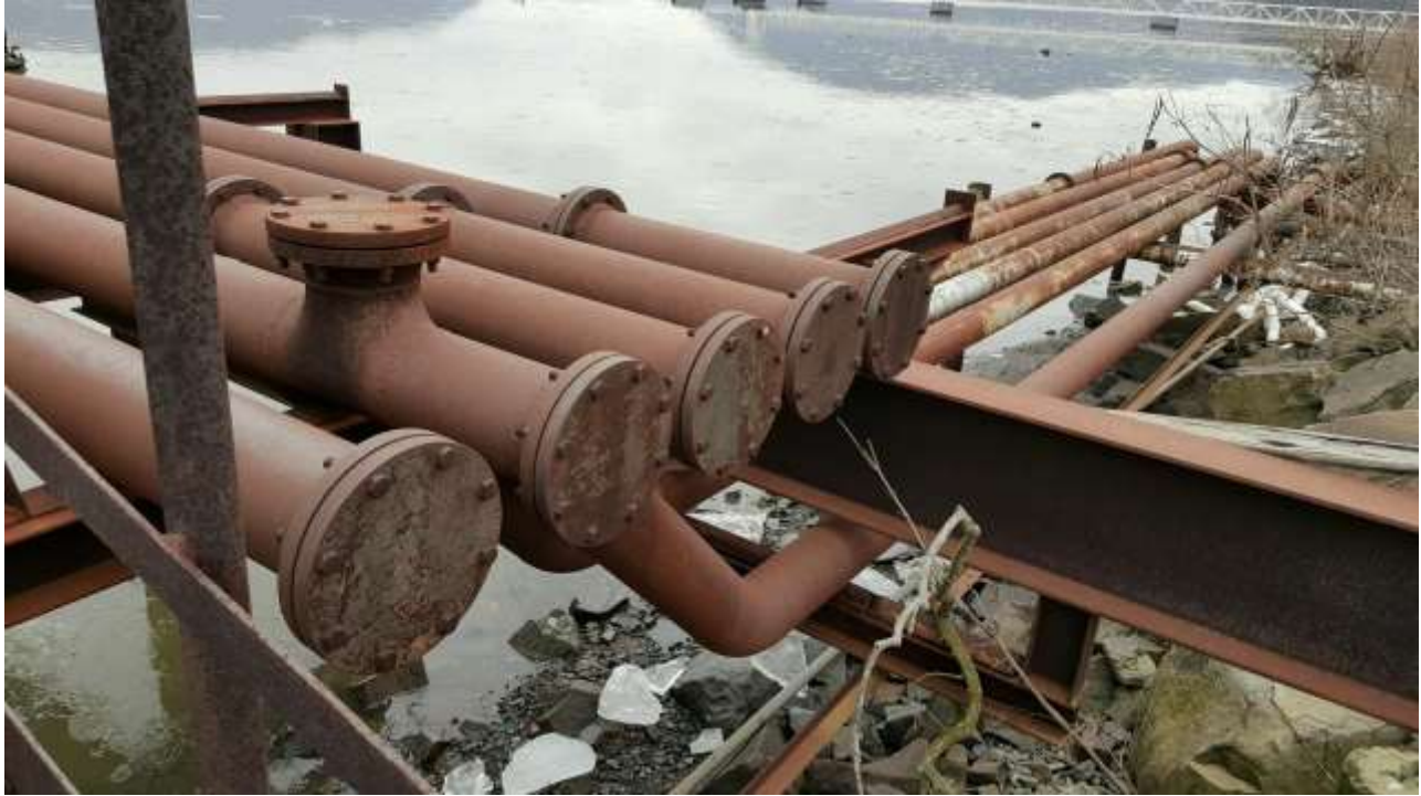
Photograph 5: Remaining onsite piping at the location of the former fuel dock.
