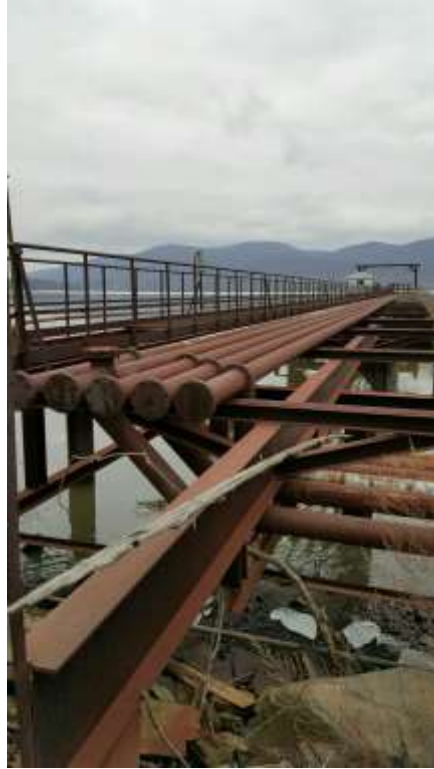
Photograph 7: Remaining onsite piping at the location of the former fuel dock.
