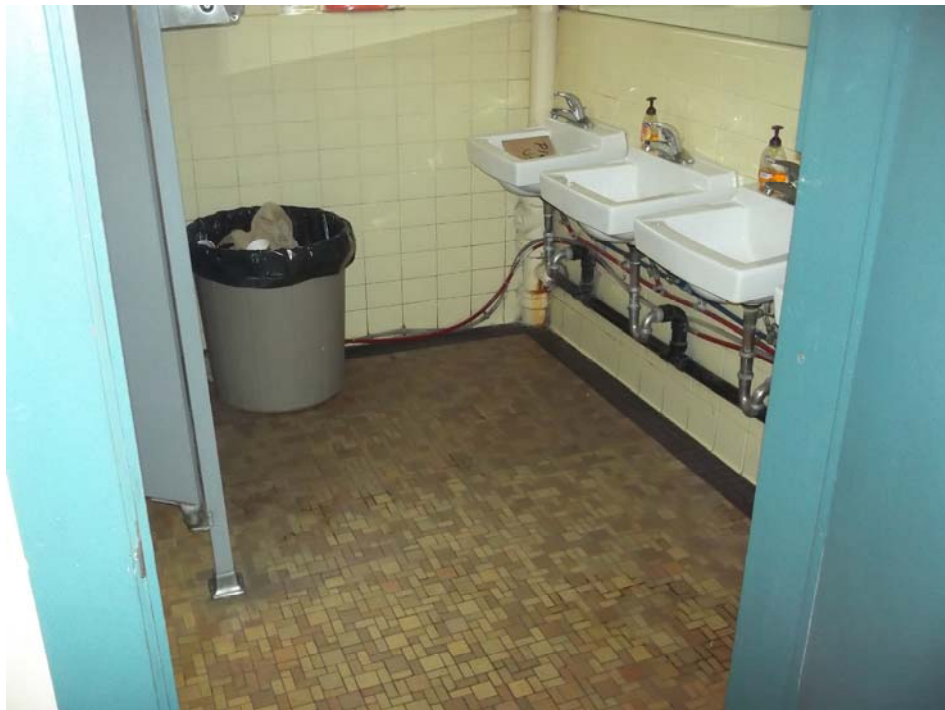
View of men's restroom.
