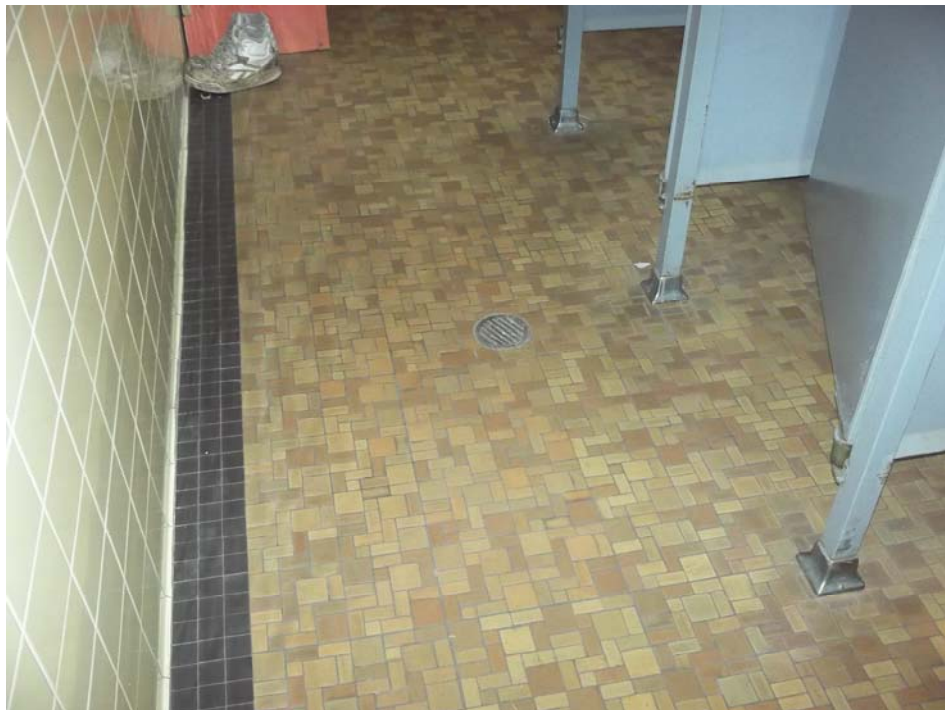
View of floor drain in men's restroom.
