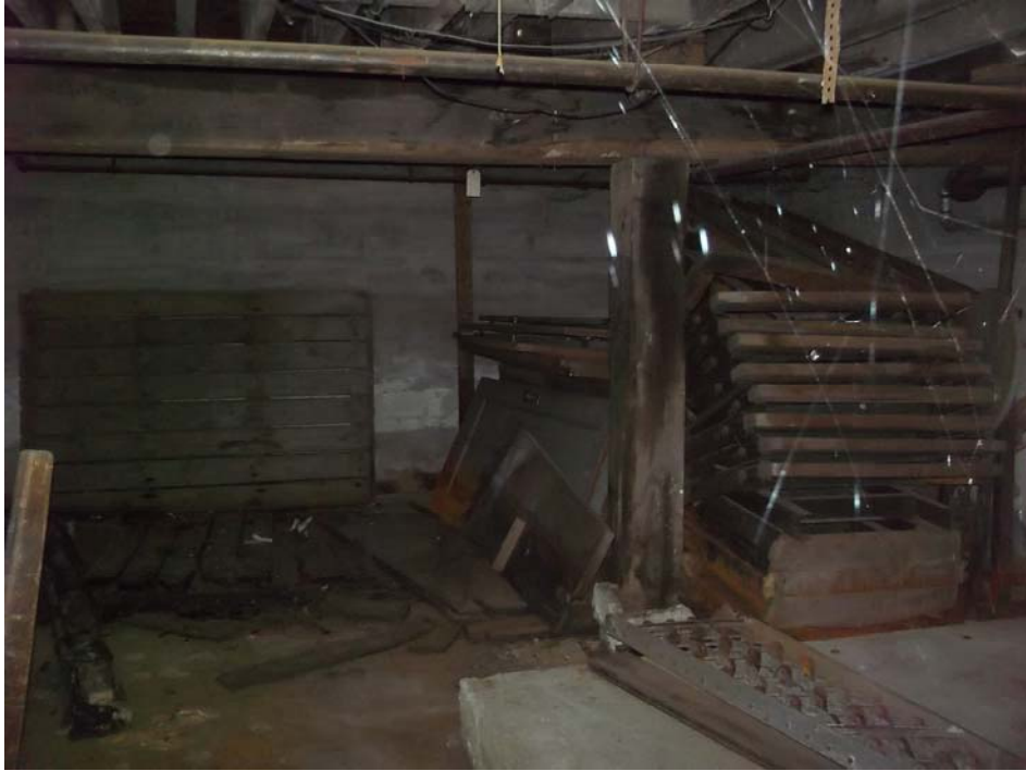
View of storage in basement area.
