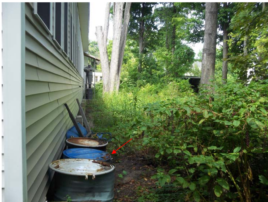
View of north side of subject building – facing west. Note drums utilized to store aluminum shavings from on-site operations.
