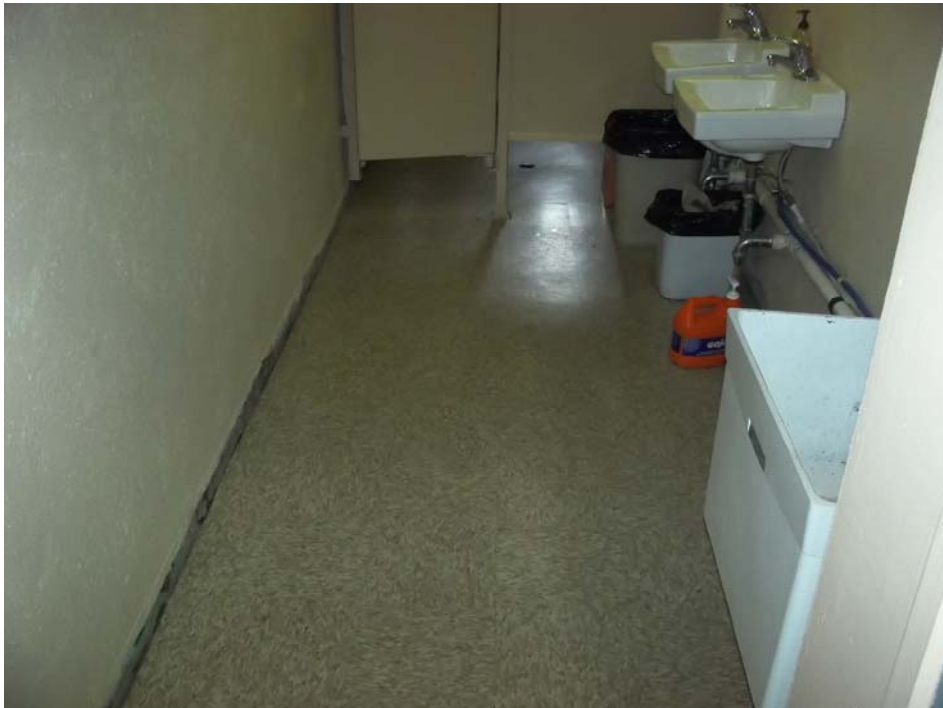
View of women's restroom.
