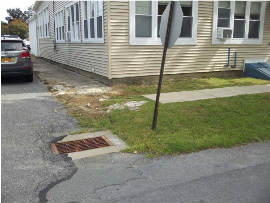
View of municipal storm water drain near southwest corner of subject property.
