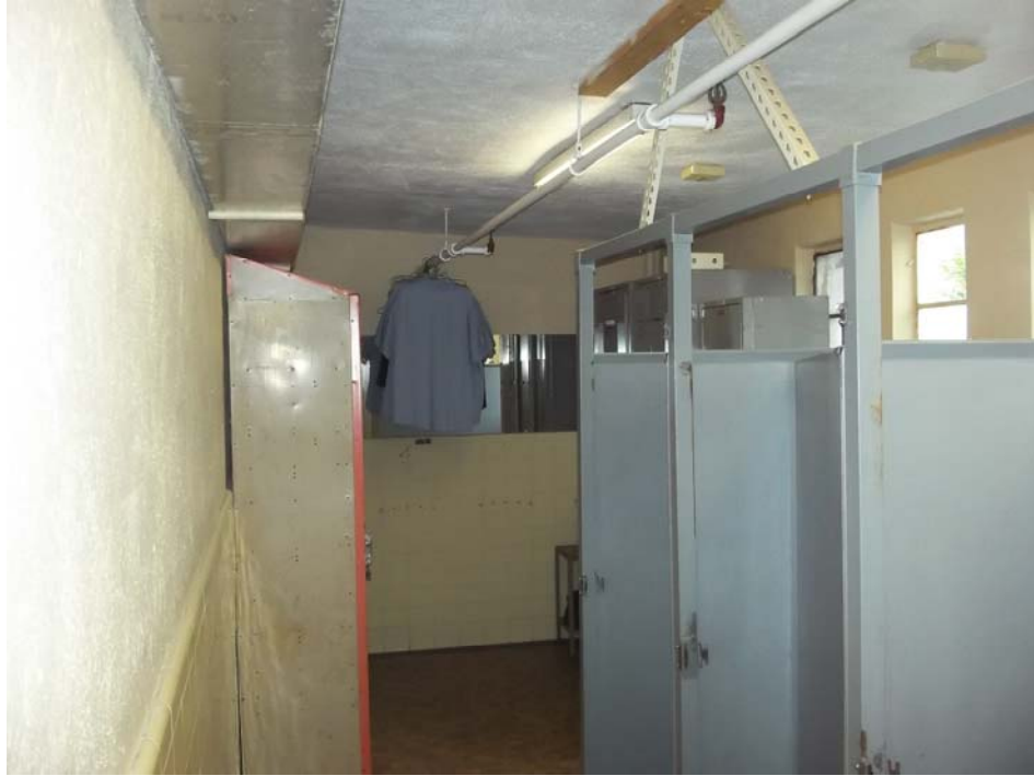
View of men's restroom.
