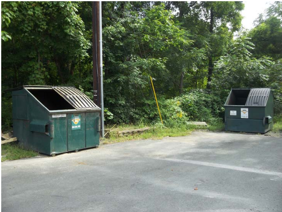
View of solid waste dumpsters to southeast of subject building.
