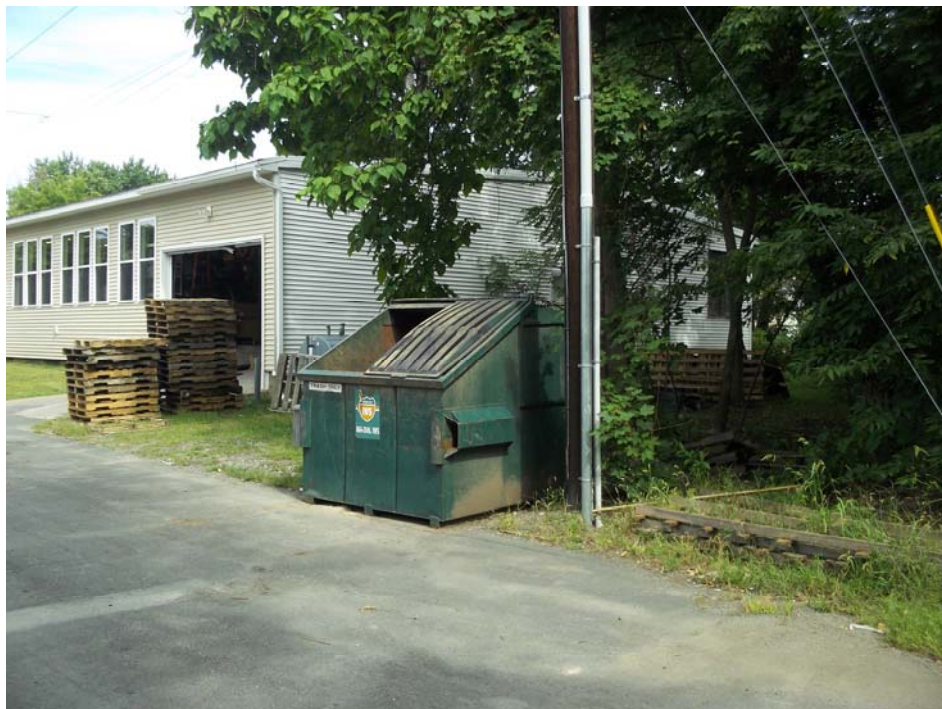
View of east side of subject building – facing west.
