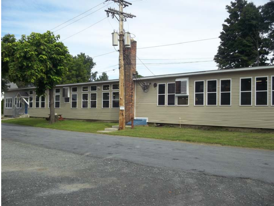
View of south side of subject building– facing north.
