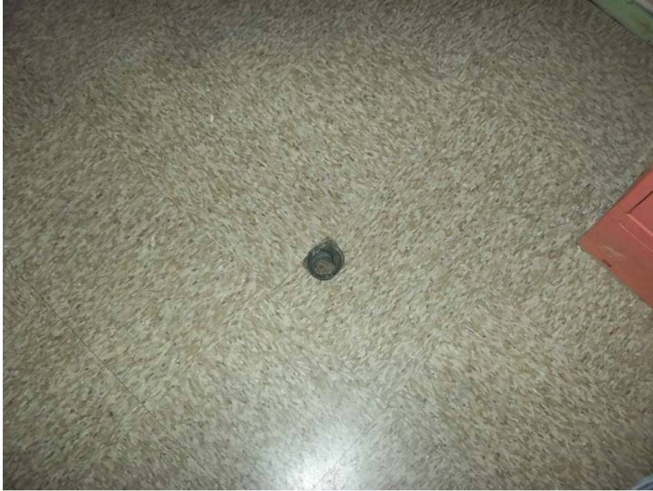
View of floor drain in women's restroom.
