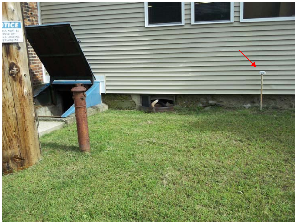
View of sprinkler system main. Note location of vent line reportedly associated with former 10,000-gallon UST, previously removed from site.
