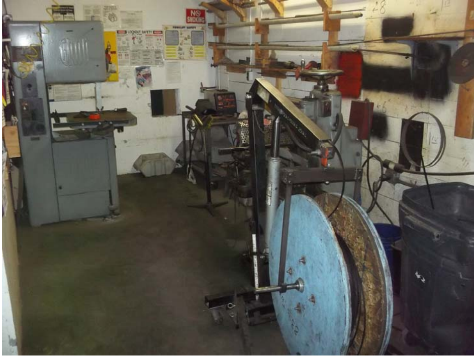
View of band saw and welder in shop area.
