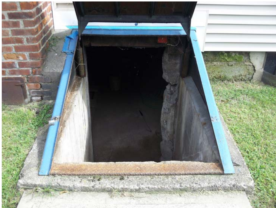
View of access to boiler room, located beneath shop area.
