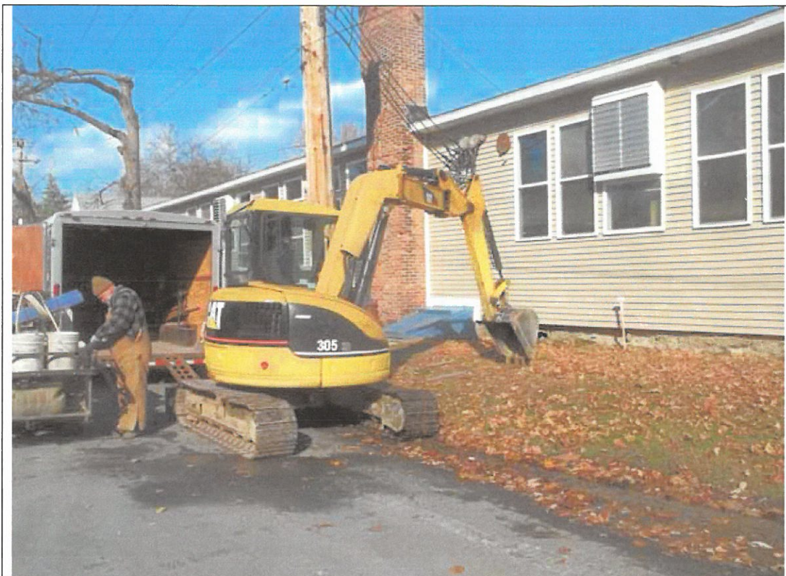
Mobile Media-Site Investigation, 175 Kelly Avenue, Pine Bush, NY Installing Test Pits Near UST Vent With Excavator
