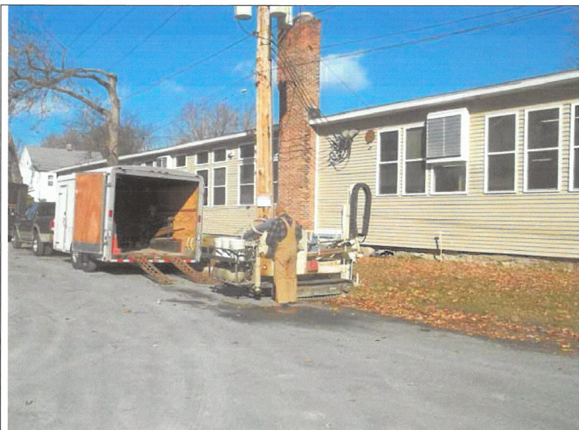
Mobile Media-Site Investigation, 175 Kelly Avenue, Pine Bush, NY Installing Soil Borings With Geoprobe
