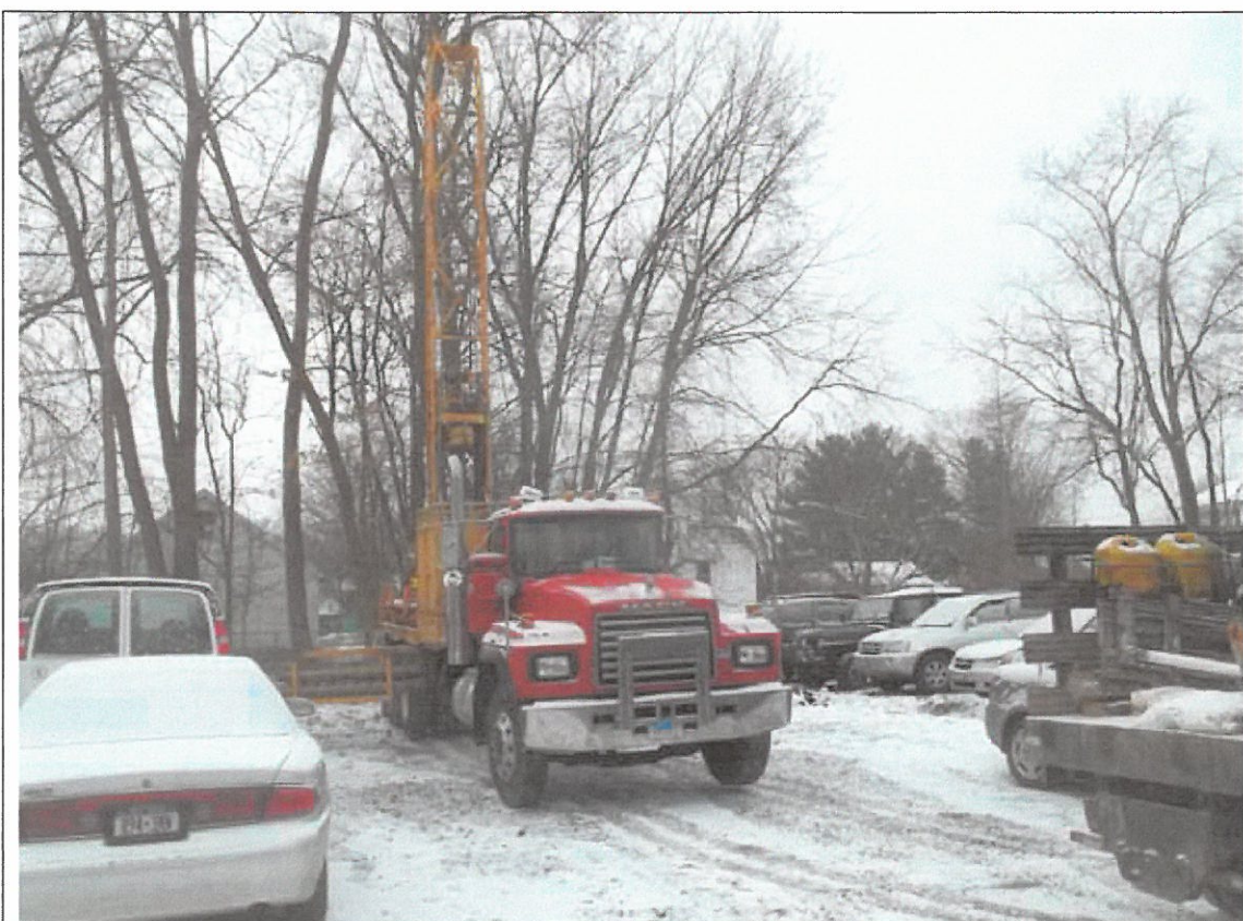
Mobile Media-Site Investigation, 175 Kelly Avenue, Pine Bush, NY Installing MW-3 With Truck Mounted Drill Rig
