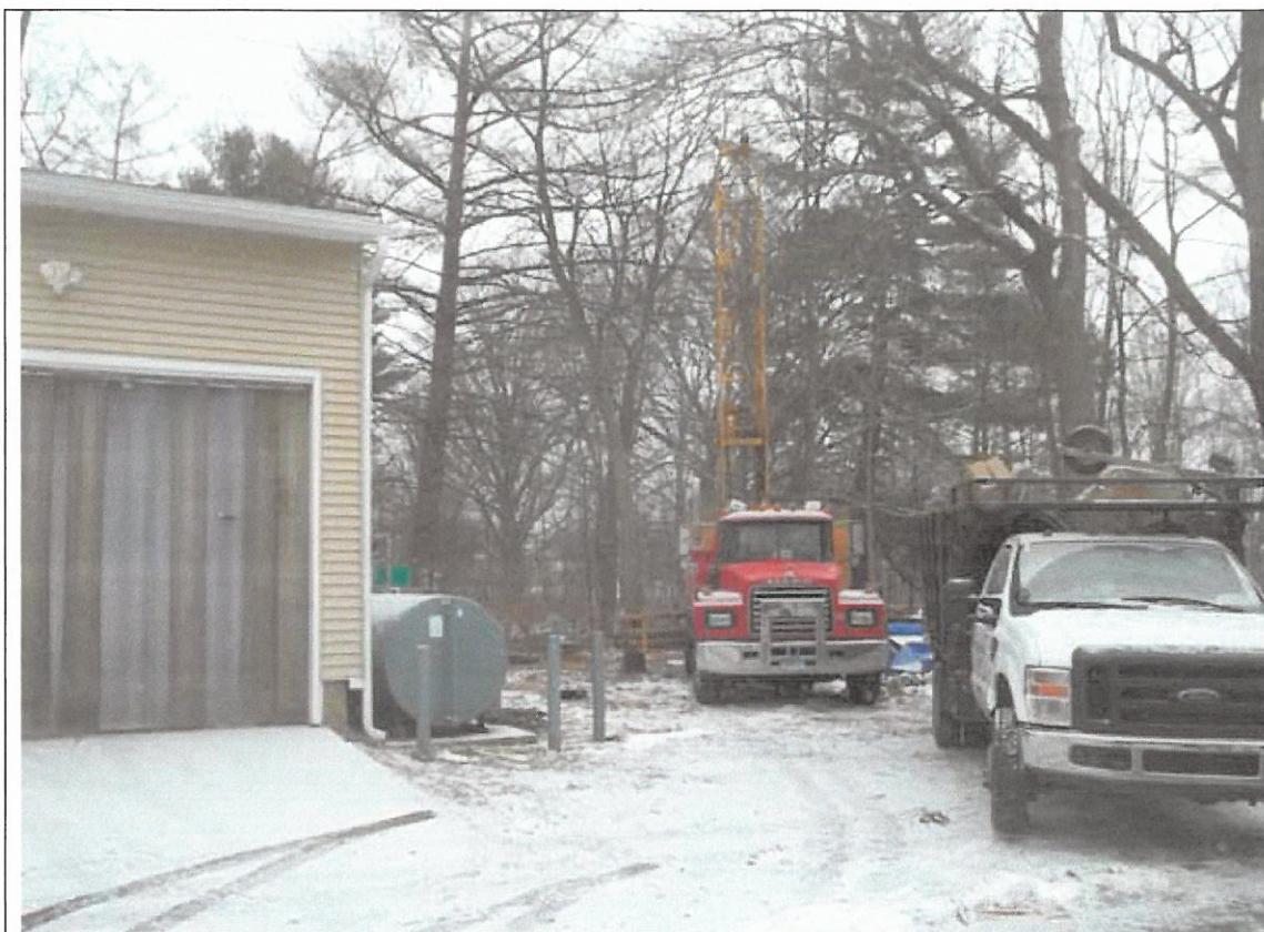
Mobile Media-Site Investigation, 175 Kelly Avenue, Pine Bush, NY Installing MW-2 With Truck Mounted Drill Rig
