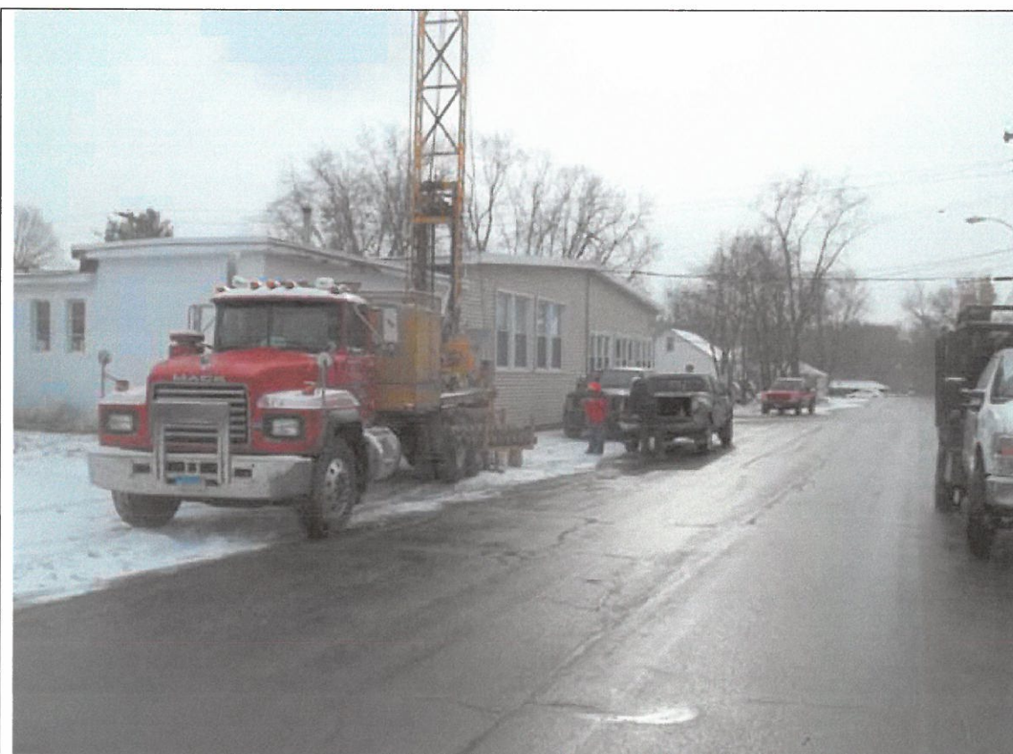
Mobile Media-Site Investigation, 175 Kelly Avenue, Pine Bush, NY Installing MW-4 With Truck Mounted Drill Rig
