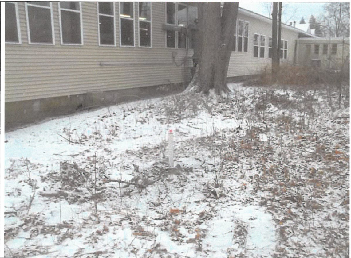
Mobile Media-Site Investigation, 175 Kelly Avenue, Pine Bush, NY Installing MW-1 With Truck Mounted Drill Rig
