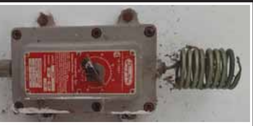
Fire-Safety Switch Former Degreaser Room
