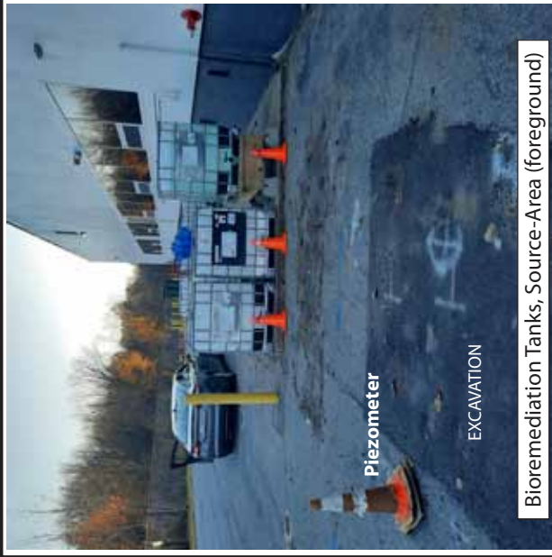
Bioremediation Tanks (Left); Source-Area Well (Cone/Right)
