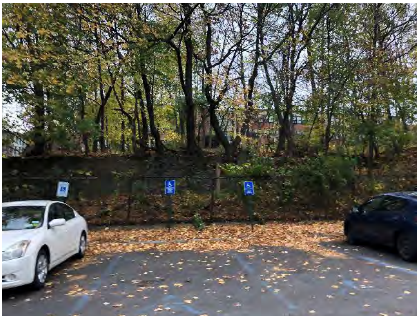
4. Retaining wall and foundation remains as viewed from the eastern adjoining property, facing west
