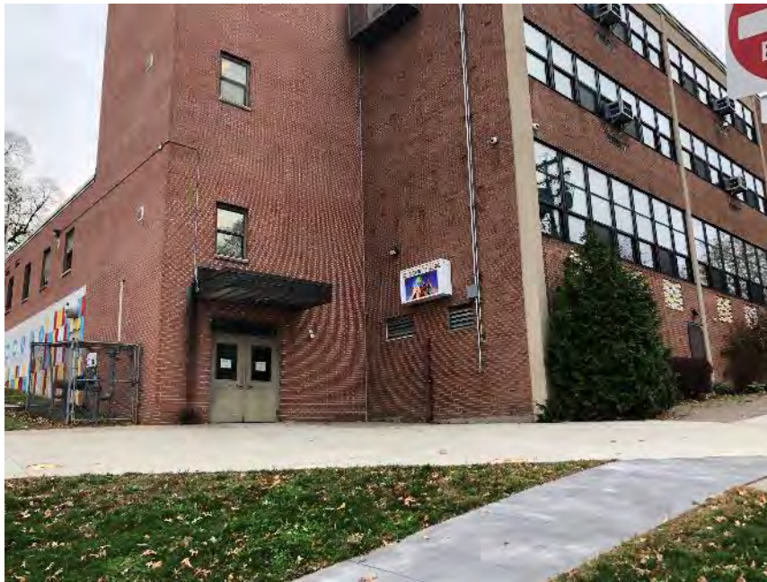
9. Western adjoining public school
