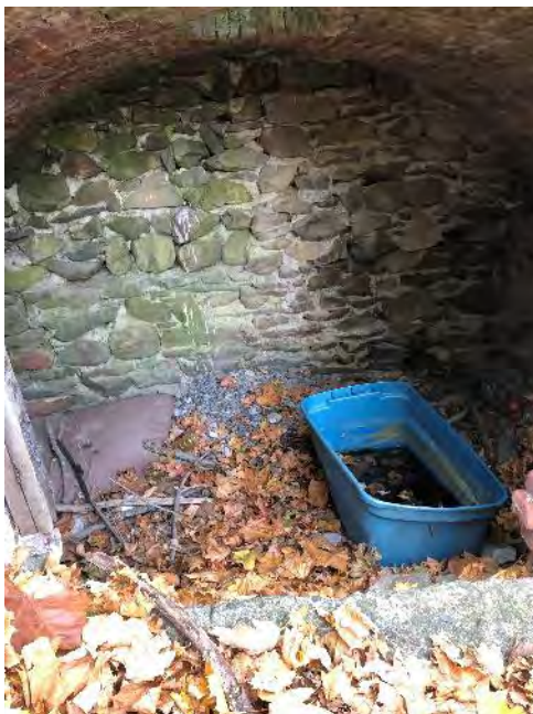
6. Trash located at cellar area
