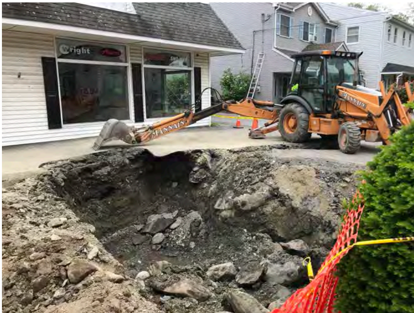
12. Looking southwest across excavation area.
