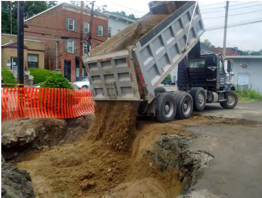
17. Delivery and placement of clean fill for excavation area
