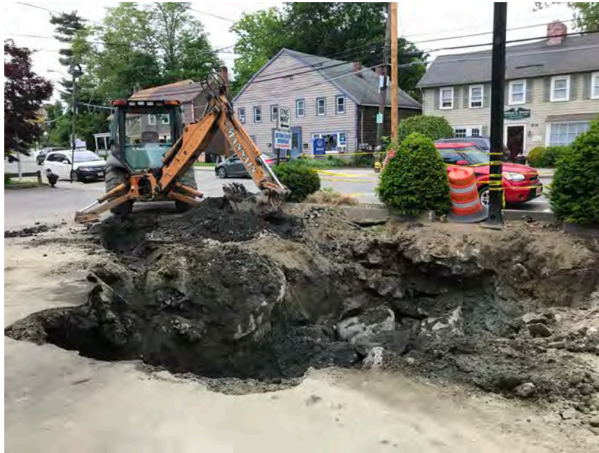
13. Looking northwest across excavation area
