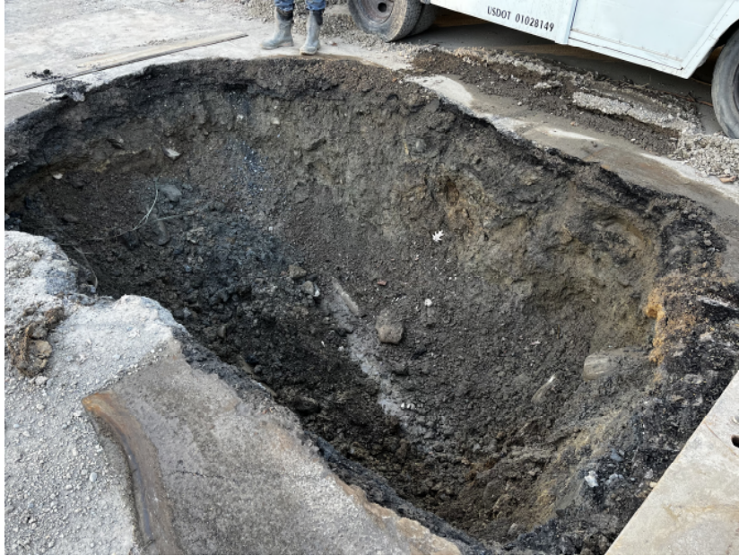
Photograph 1: View of 317 Main Street excavation.
