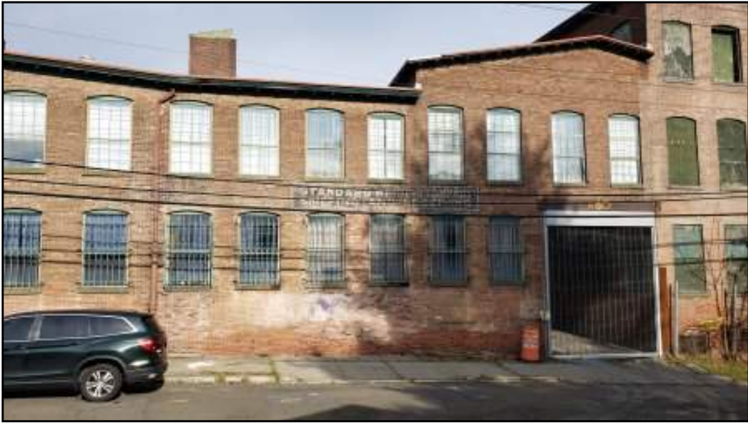
Adjoining property to the north.
