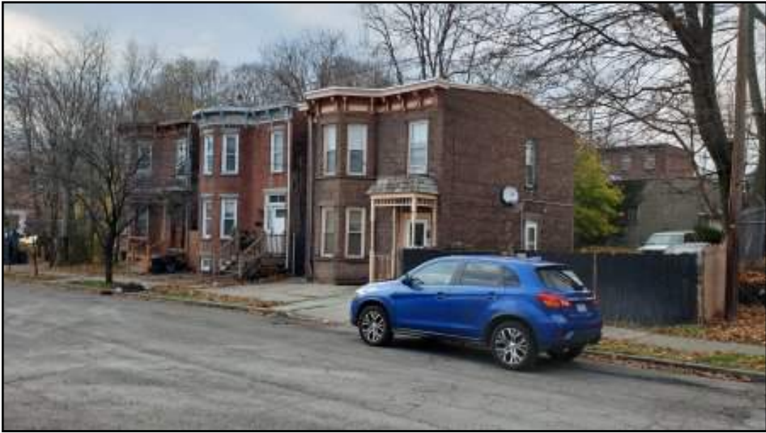
Adjoining property to the west.
