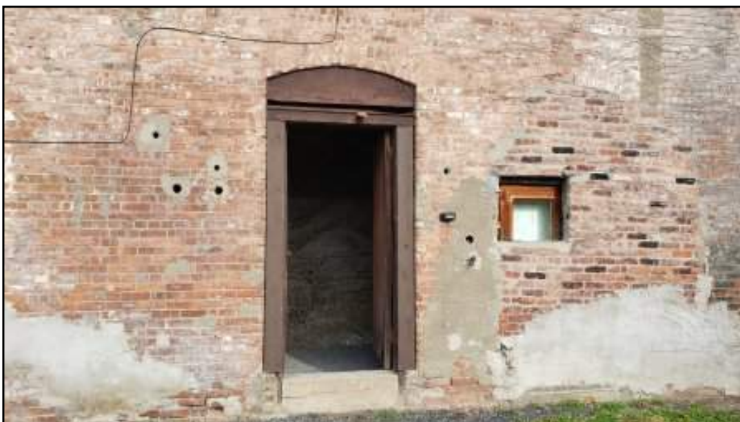
View of the entrance to the former tank room.
