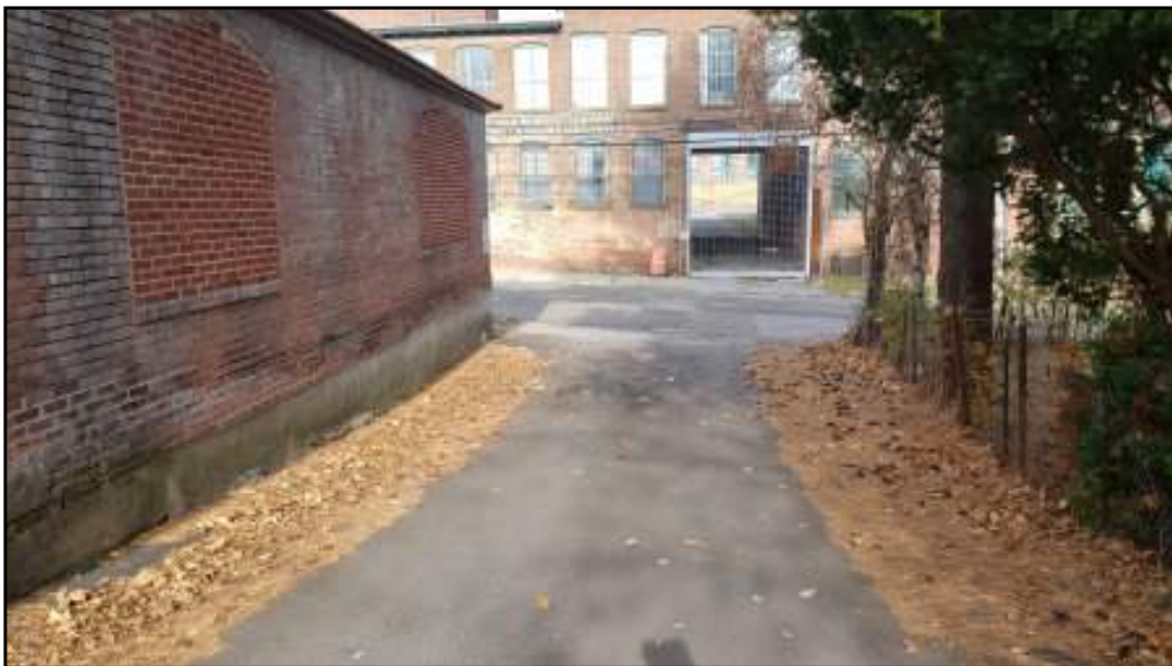
Facing north, view of the main entrance to the subject property.
