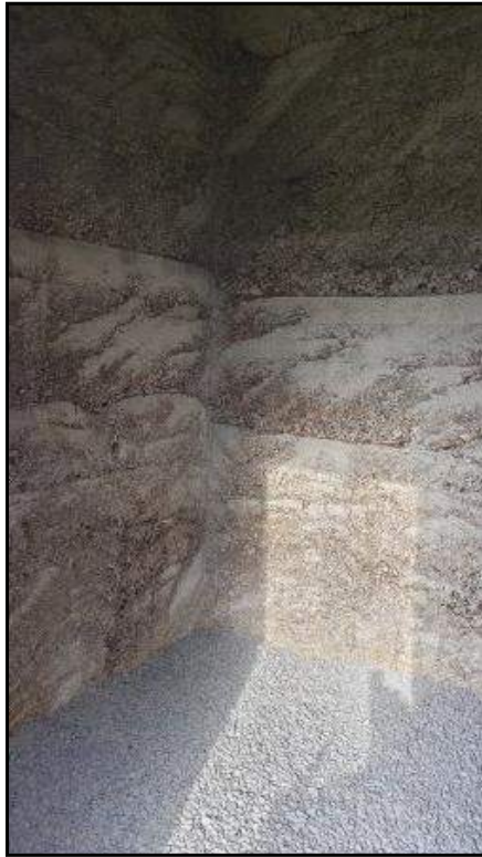
View of the interior of the former tank room.
