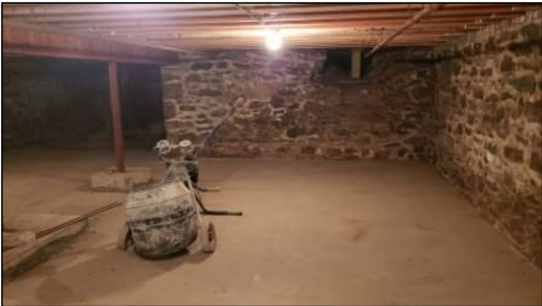
Typical interior of the basement in the on-site building.
