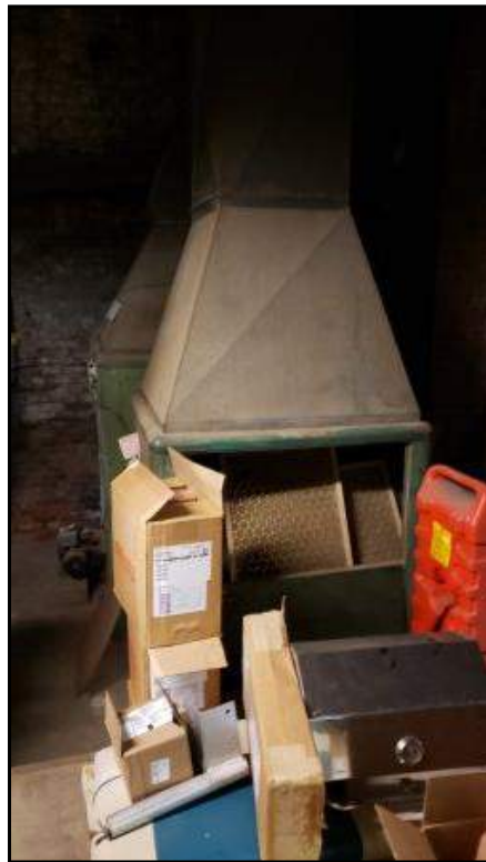
View of the interior of the decommissioned boiler room.
