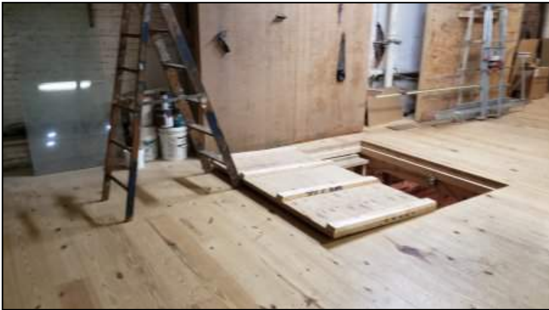
Entry-way to the basement of the on-site building.
