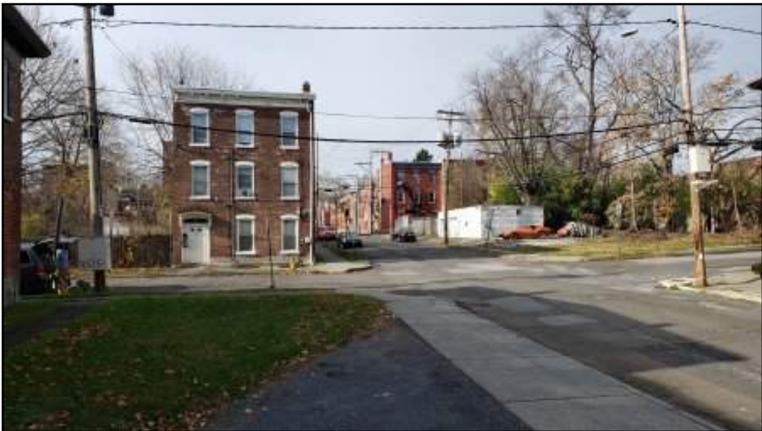
View of the northern exterior of the subject property.
