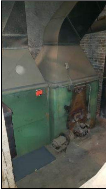
View of the interior of the decommissioned boiler room.
