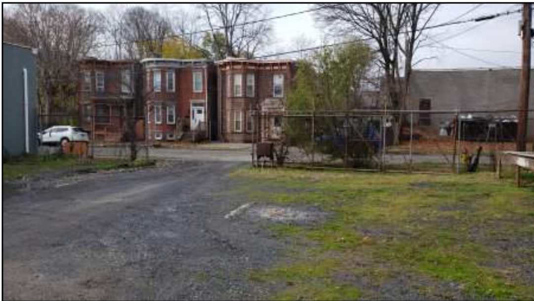
Facing west, view of the southern exterior of the subject property.
