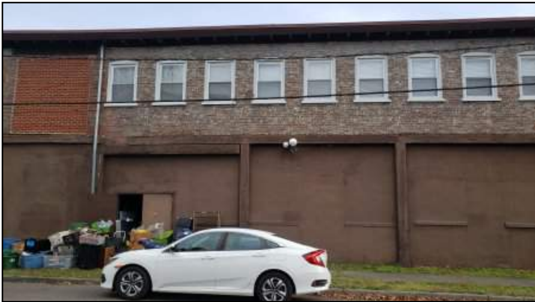
View of the western exterior of the on-site building from Johnes Street.
