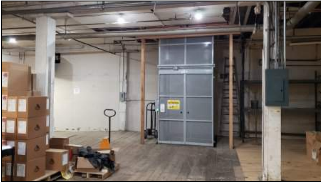
Typical interior of the first floor.
