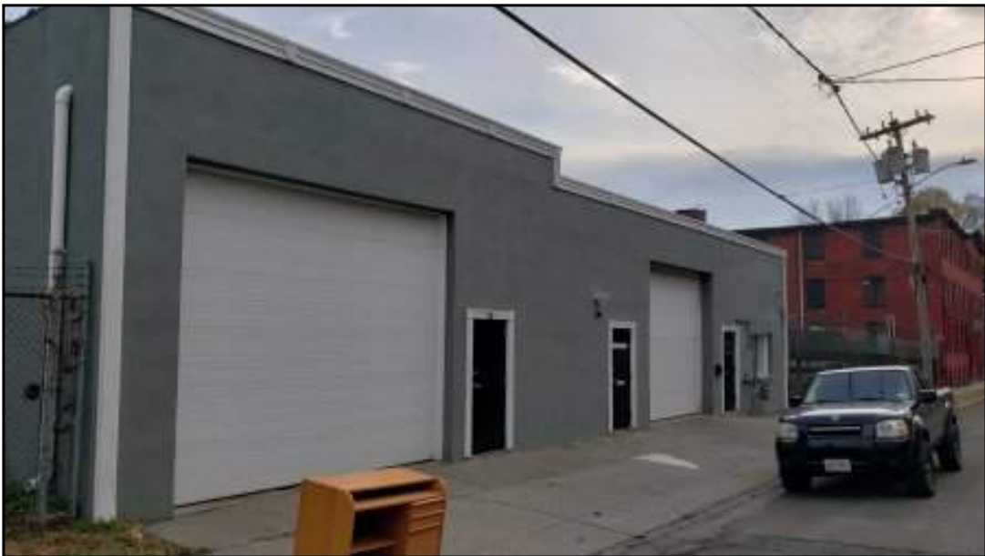
Adjoining property to the south.
