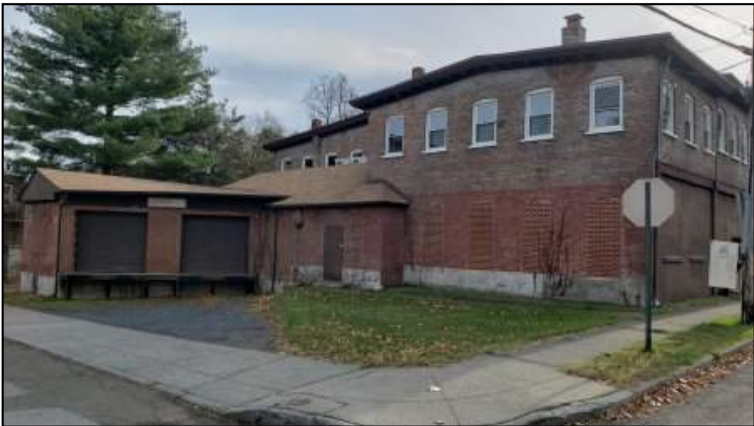
View of the on-site building on the subject property from South William Street.
