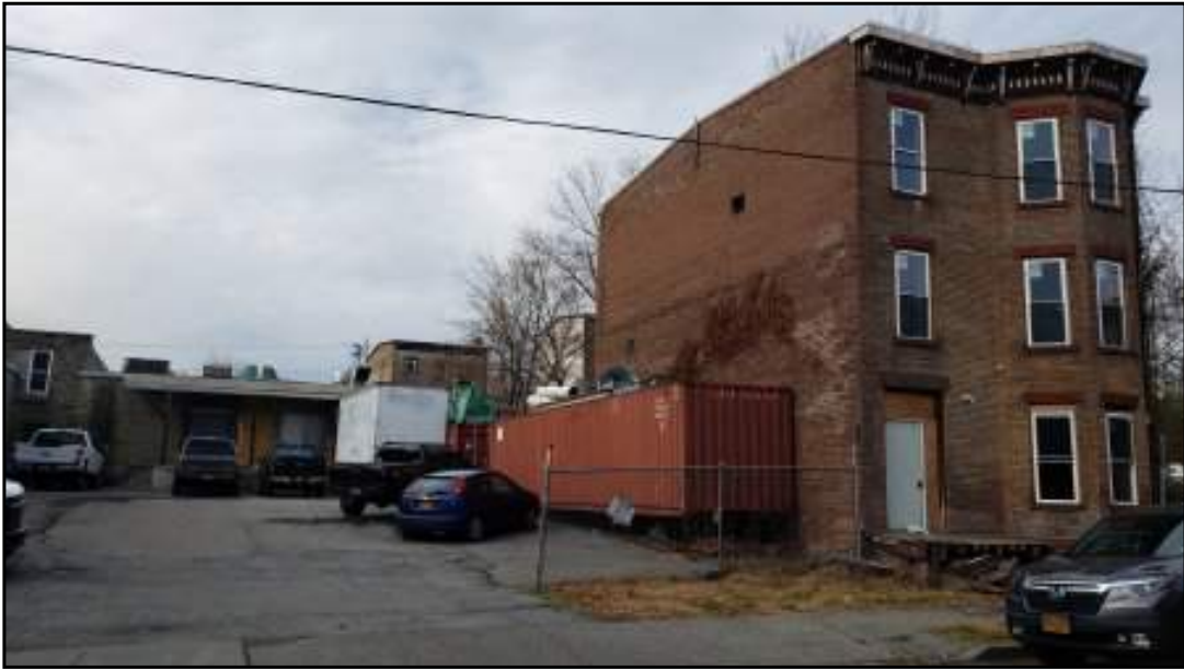
Adjoining property to the west.
