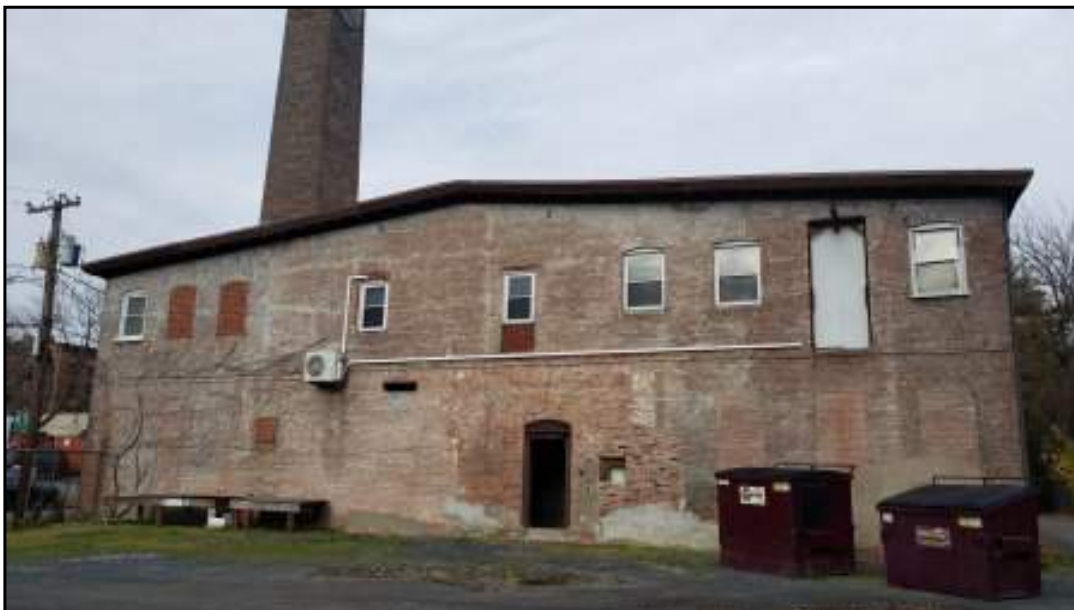
Facing north, view of the southern exterior of the on-site building.
