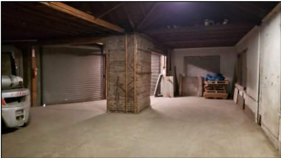
Facing north, view of the loading dock area on the first floor of the building.
