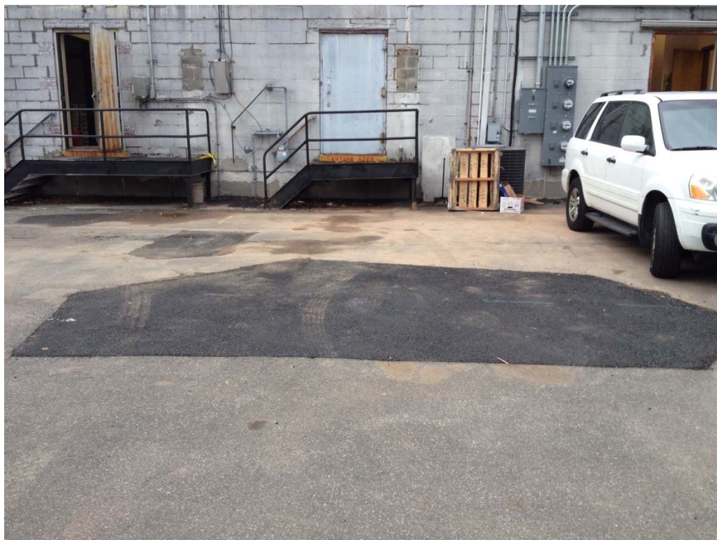
View to the west of the waterline and gas line repairs made to the east of building #2 in November 2014
