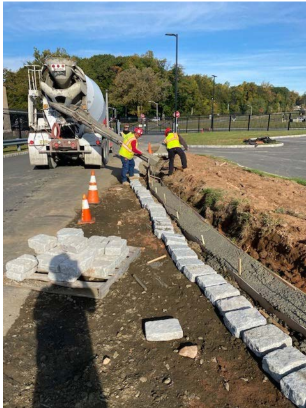
Photo 2: Pouring belgian block tie-in to existing curb-line at VVRC.
