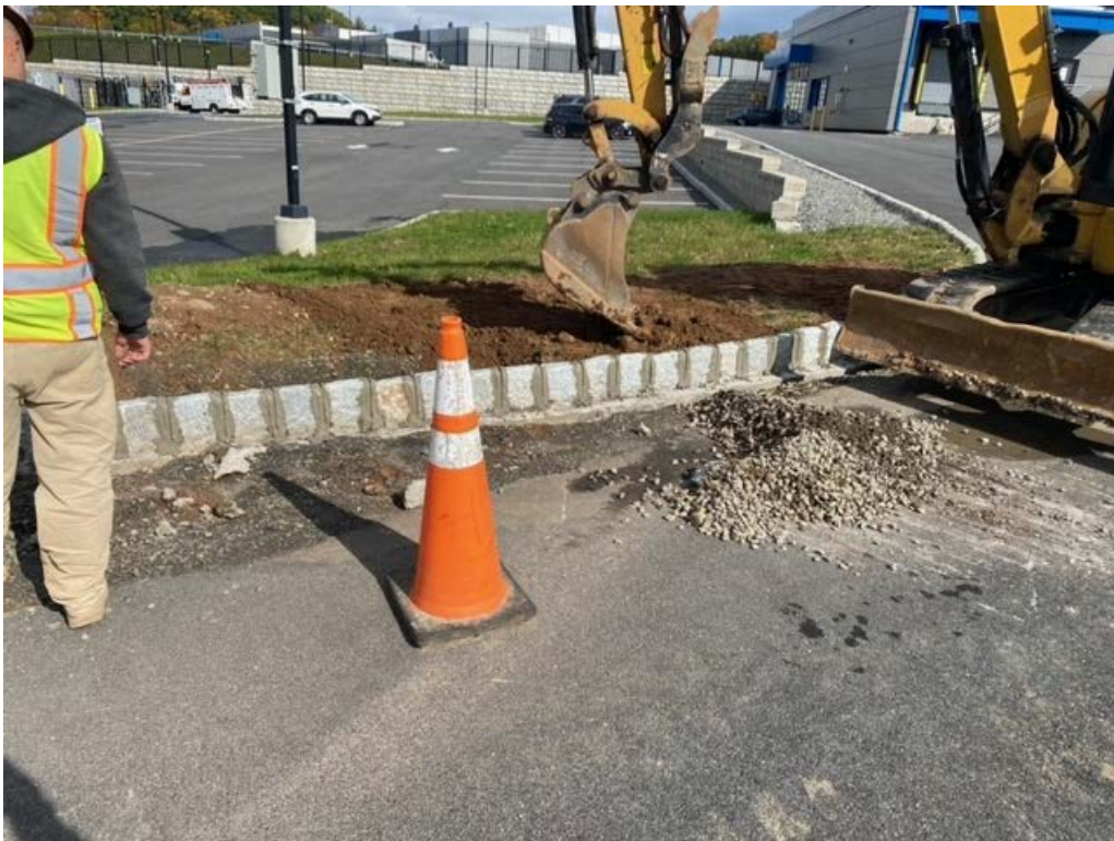
Photo 2: Applying mortar joints for VVRC curbing area.
