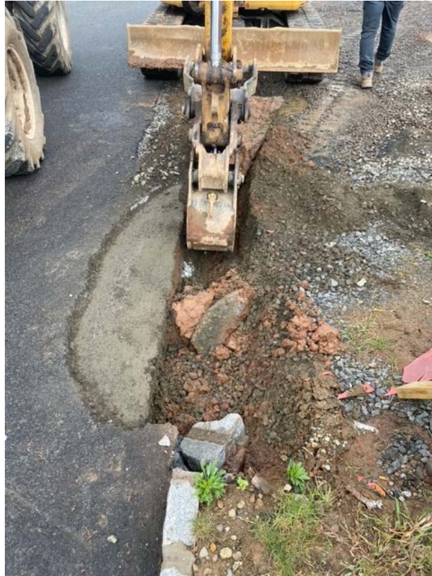
Photo 1: Excavating curb at Building G.
