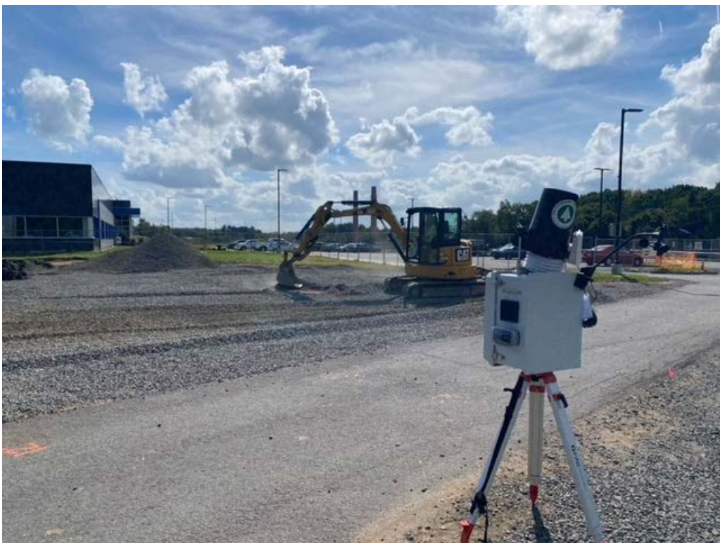
Photo 2: Removal of ¾" stone at Building G.
