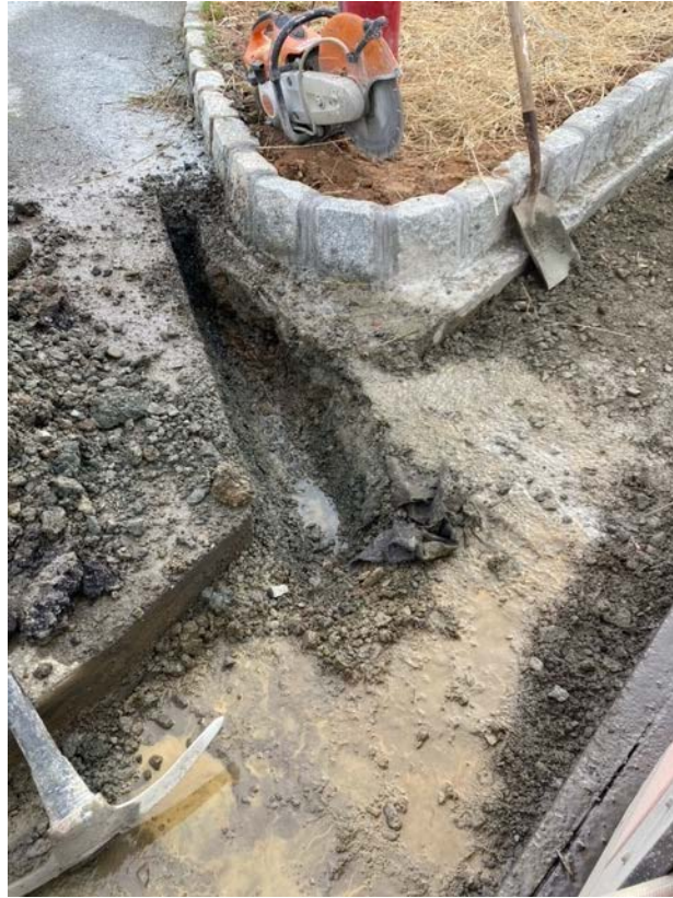
Photo 1: Expand drainage radius at far west portion of tie-in at VVRC.
