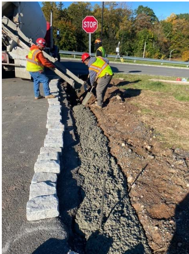
Photo 2: Pouring along sidewalk area in at Building G west.
