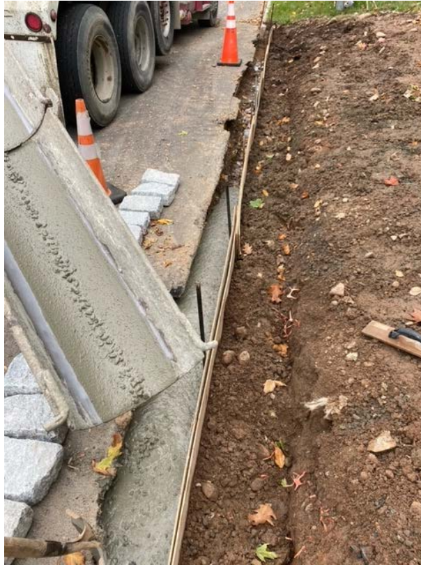
Photo 1: Concrete pouring at Building G.
