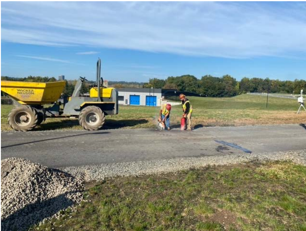
Photo 2: Demolition saw with water to cut asphalt.
