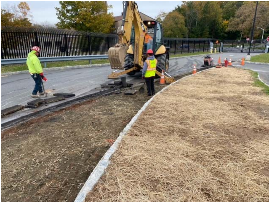
Photo 2: Wet saw cut asphalt at VVRC.
