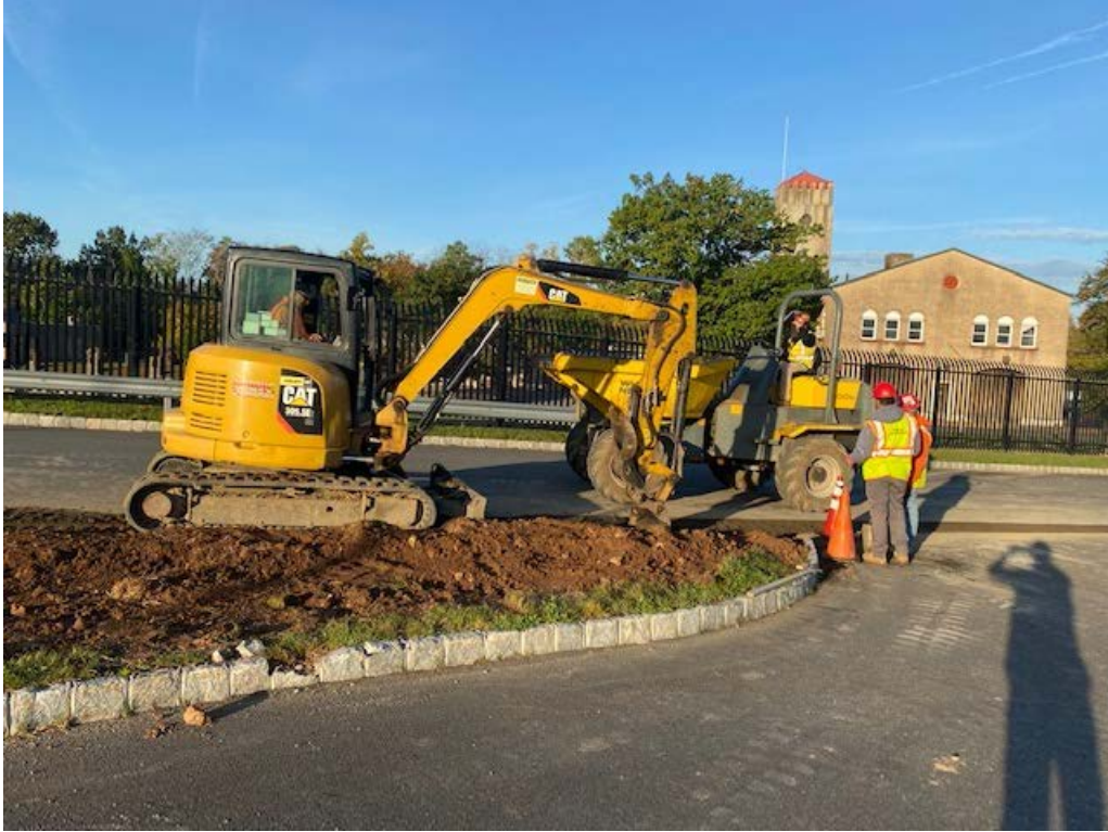
Photo 1: Placing forms at curb-line to be cemented.
