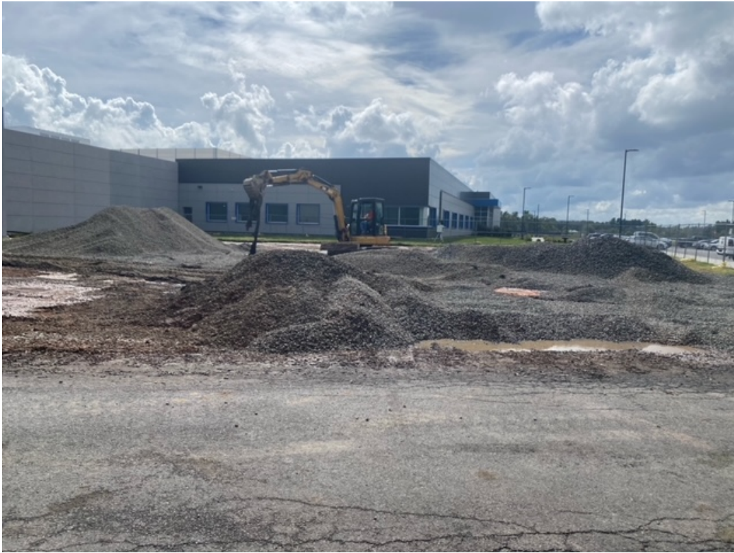
Photo 1: Removal of 3/4" stone at Building G.
