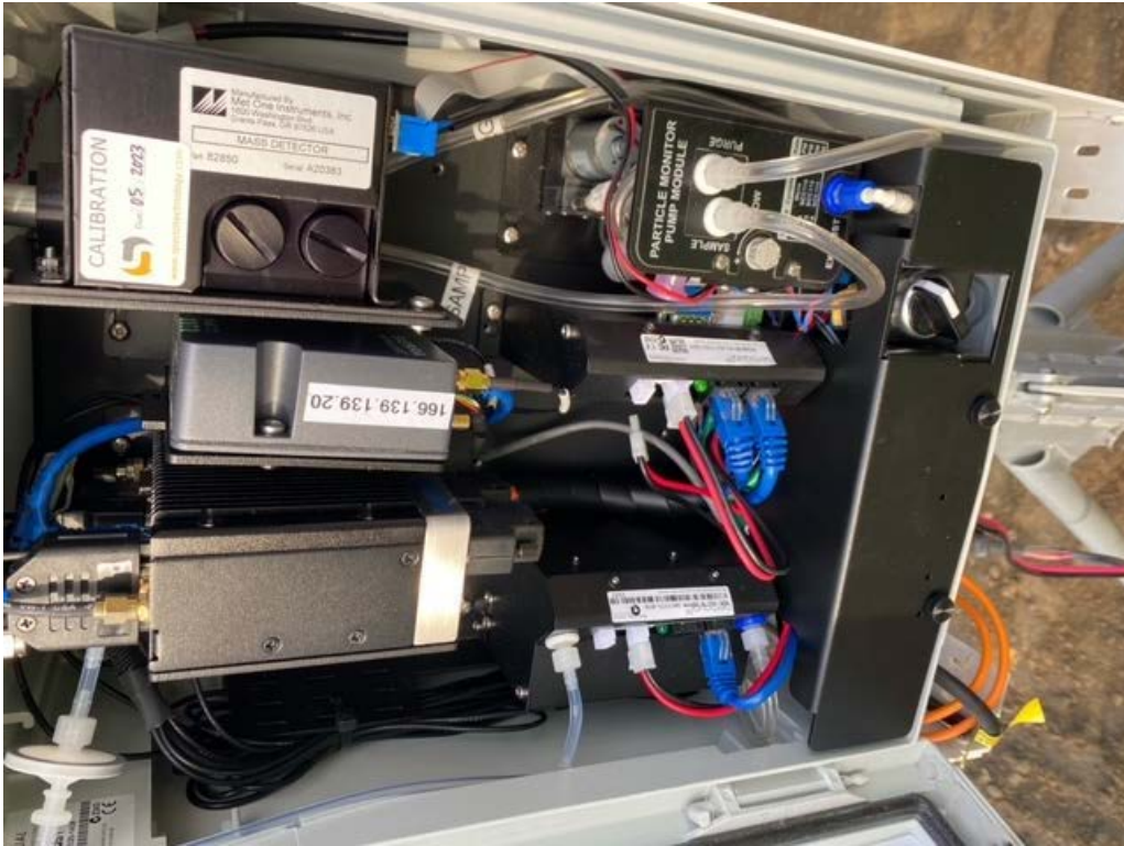
Photo 1: Troubleshooting CAMP Station 1.
