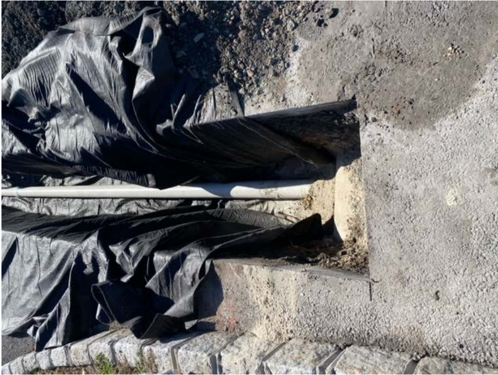
Photo 1: Excavating along VVRC roadway and tying into existing drain.
