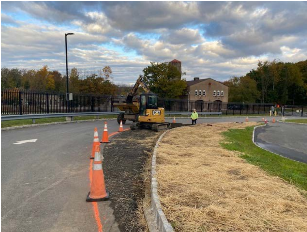
Photo 2: Milling, excavating, and cutting asphalt for tie-in at VVRC area.
