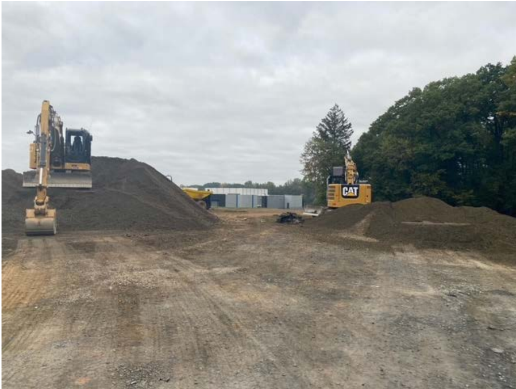
Photo 1: Removal of DGA from trailer yard.
