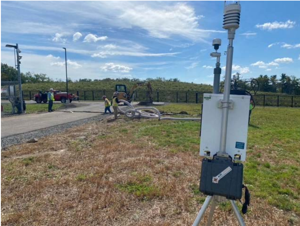
Photo 1: CAMP monitoring at drainage trench installation.
