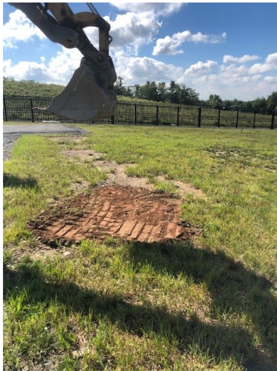
Photo 2: Waste class sampling test pit at substation.
