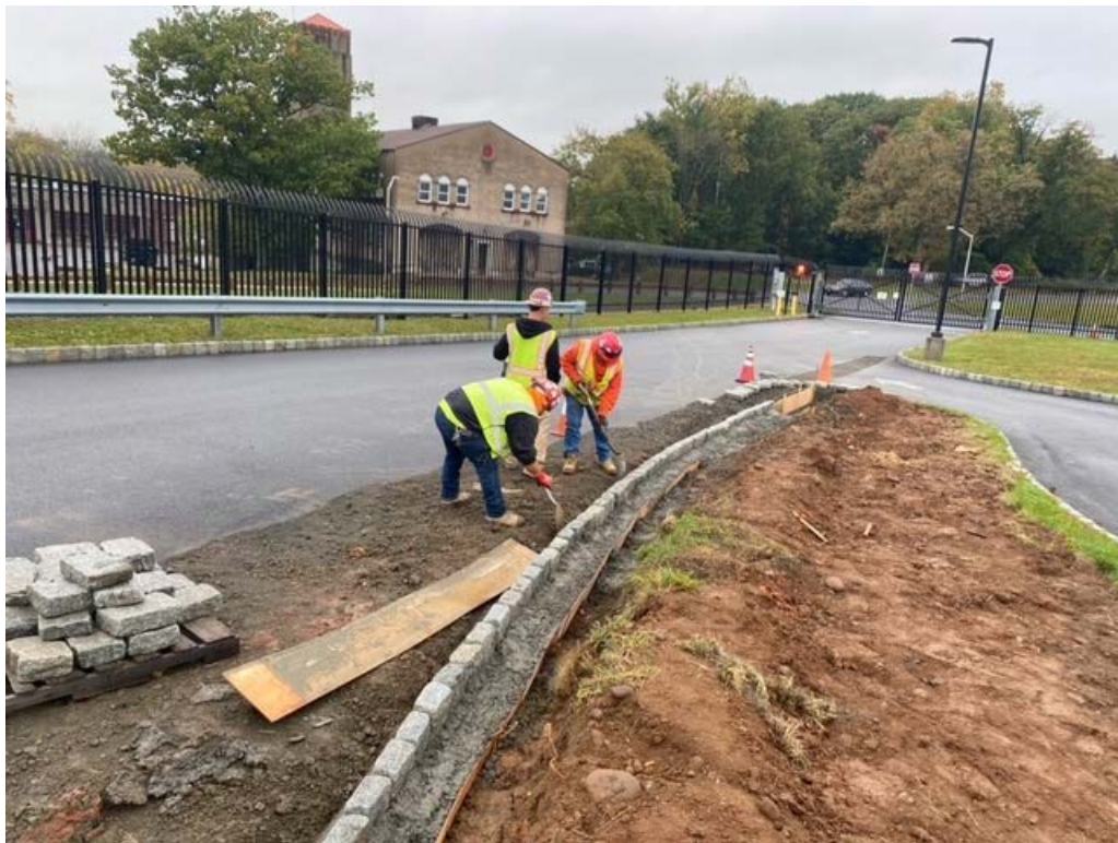
Photo 2: Removing forms from VVRC curb pour.
