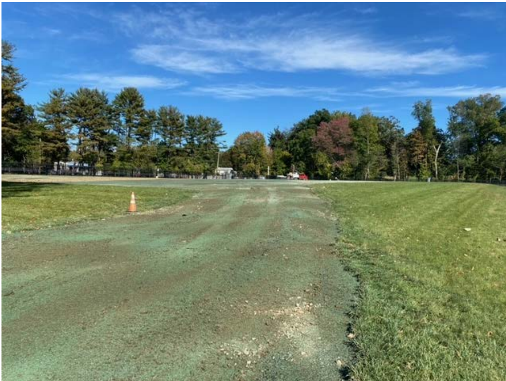
Photo 2: Hydroseeding former northern trailer area.
