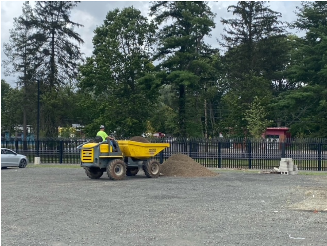
Photo 2: Begin staging at northern former trailer yard area.
