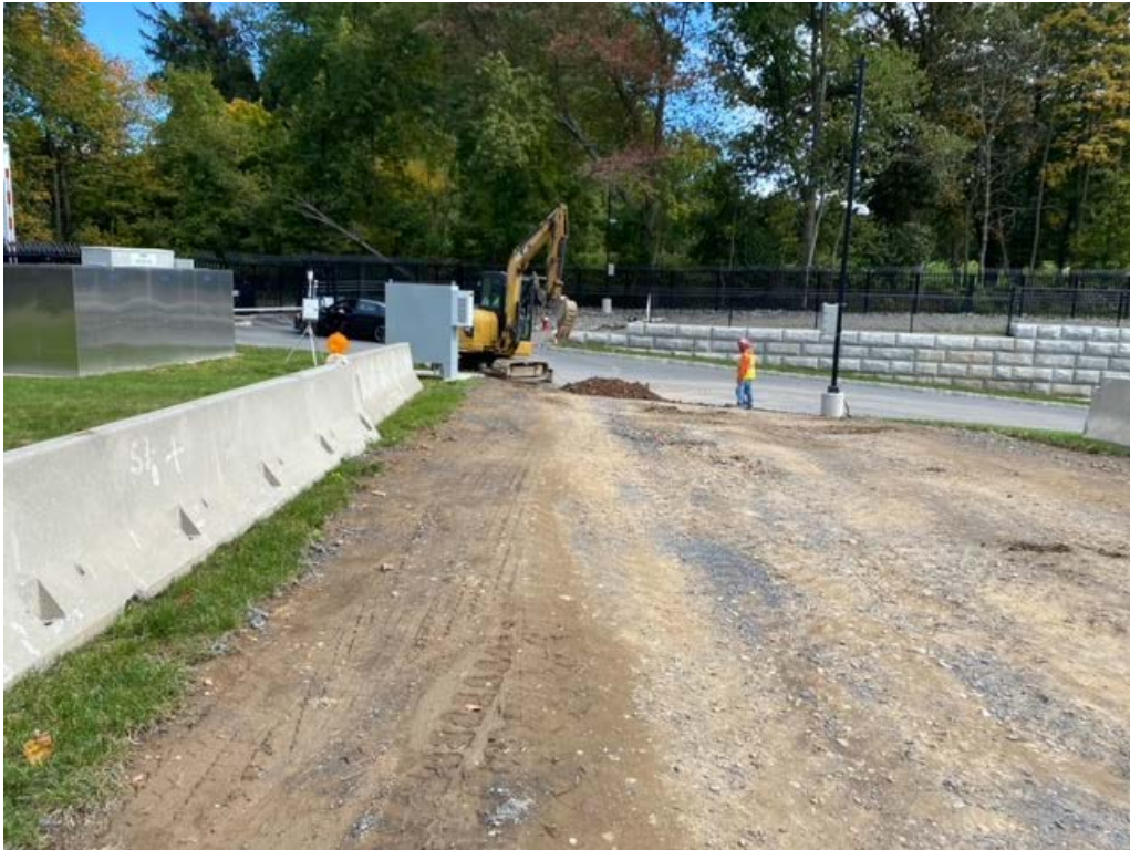
Photo 2: Northeast ramp excavation.
