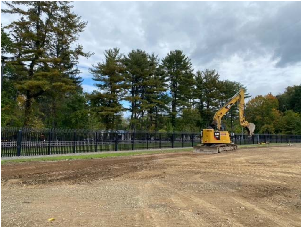
Photo 1: Grading former trailer yard.
