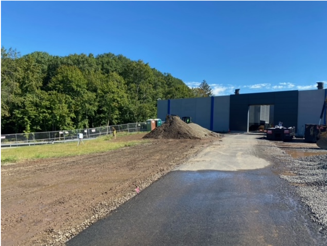
Photo 1: Completing removal of ¾" stone at Building G.
