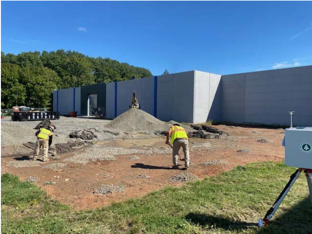
Photo 1: Removal of ¾" stone at Building G.
