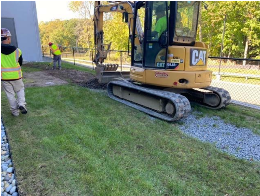
Photo 2: Scrape minimal stone from former Building G walkway.
