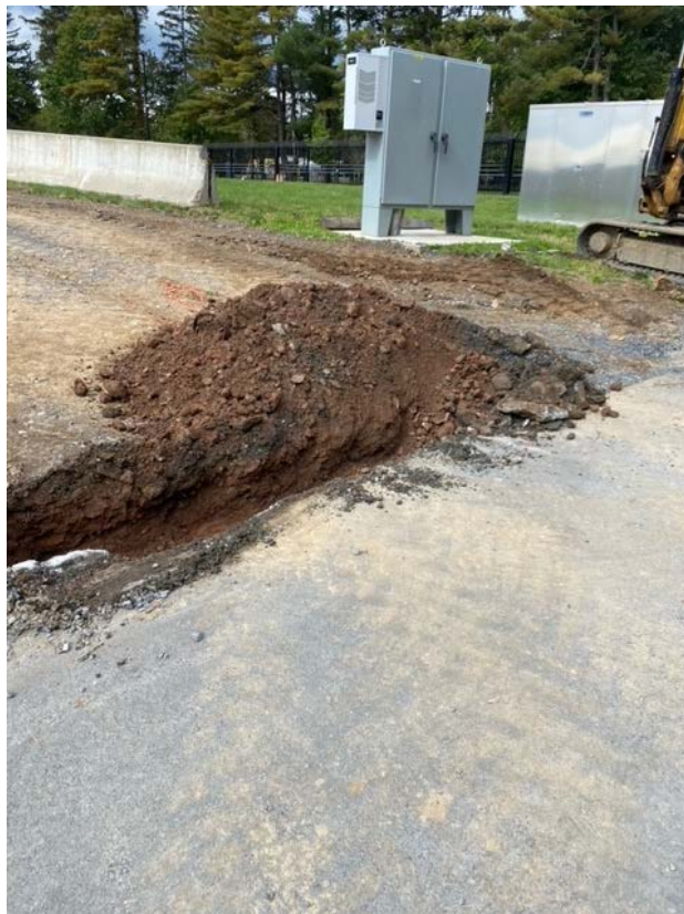
Photo 2: Excavating berms at VVRC parking area.
