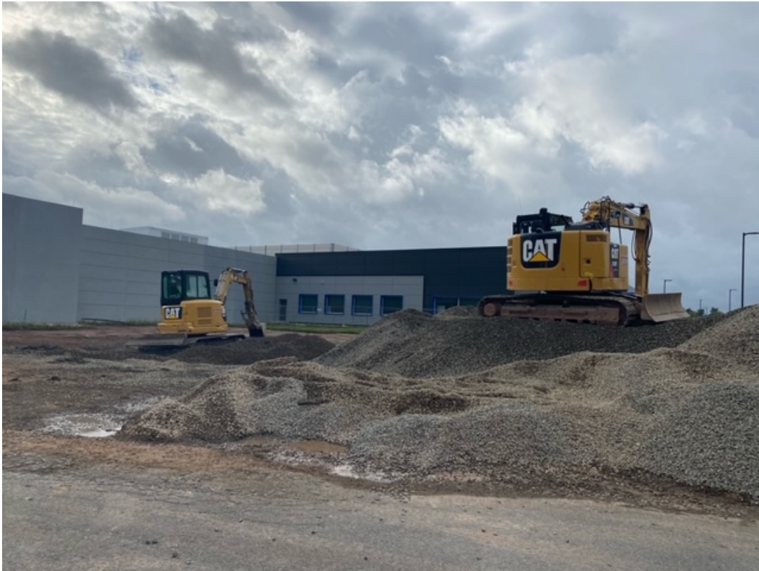
Photo 1: Removal of 3/4" stone at Building G.
