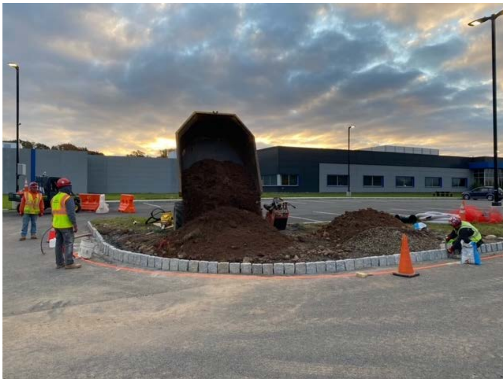
Photo 2: Backfilling curb area at Building G.
