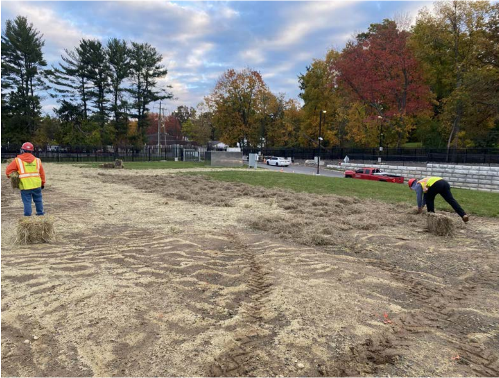
Photo 1: Continues with hay installation in northern former trailer yard.
