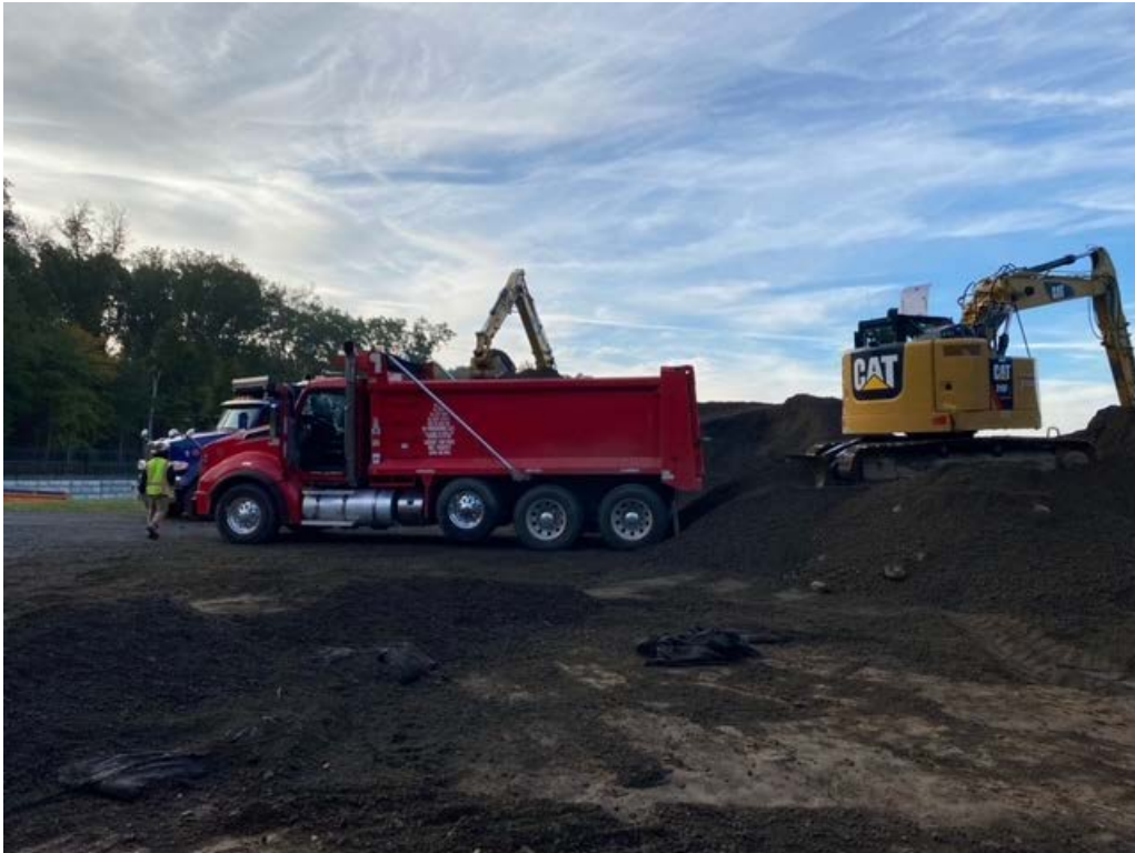
Photo 2: Spread additional stone throughout the substation area.
