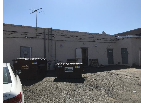
#2: VIEW OF BACK (NORTH SIDE) OF PROJECT BUILDING
