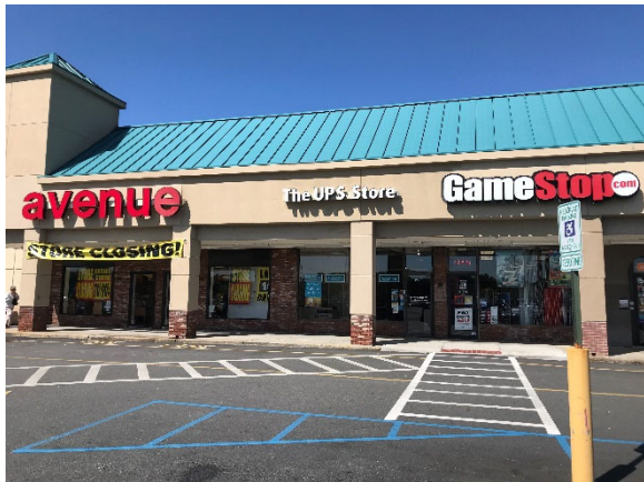
#1: VIEW OF FRONT (SOUTH SIDE) OF PROJECT BUILDING
