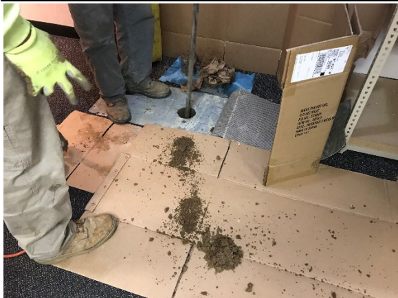
#3: VIEW OF INTERIOR SOIL BORING SB-1 AND SOIL REMOVED FROM LOCATION
