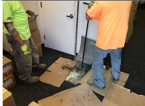
#4: VIEW OF SOIL BORING SB-2
