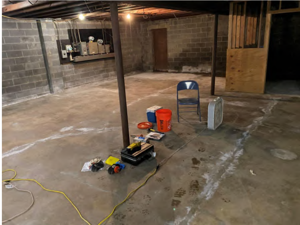
Photograph 13 – Concrete chip sample collection work area.
