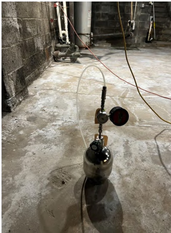
Photograph 11 – Sub-slab soil vapor sample collection.
