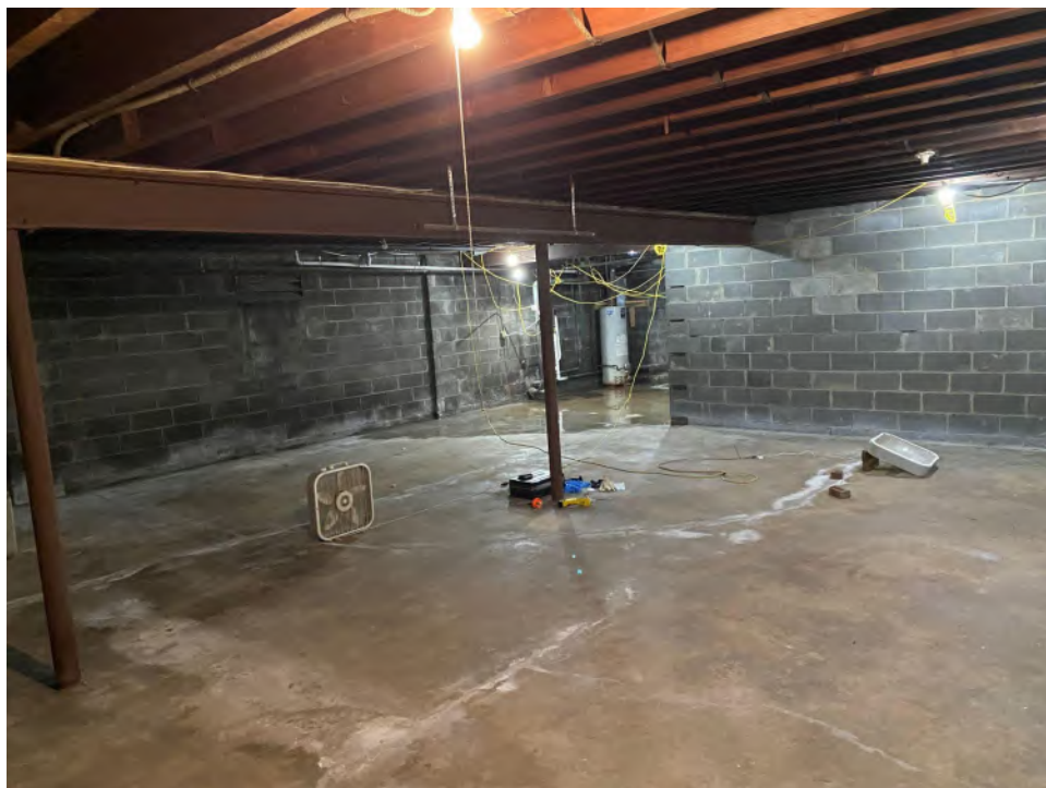
Photograph 14 – Concrete chip sample collection work area.
