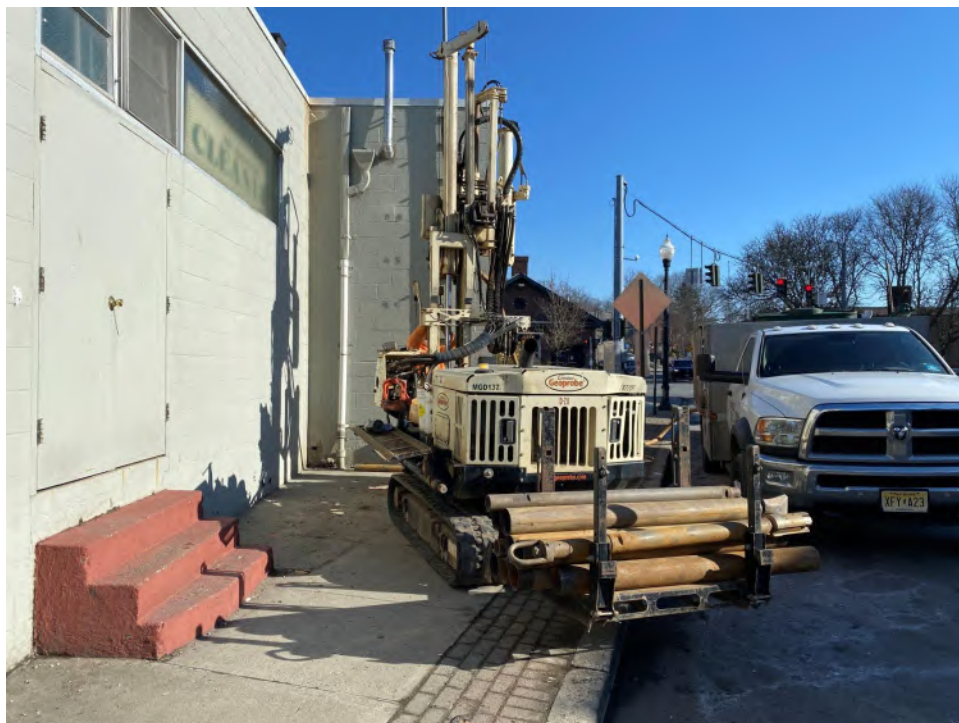
Photograph 4 – MGD137 Geoprobe, seen here installing monitoring well MW-2 (along Chestnut Street).
