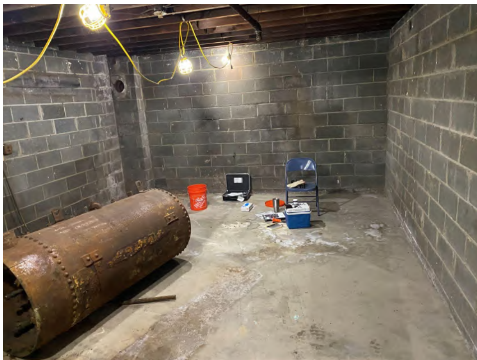
Photograph 12 – Concrete chip sample collection work area.
