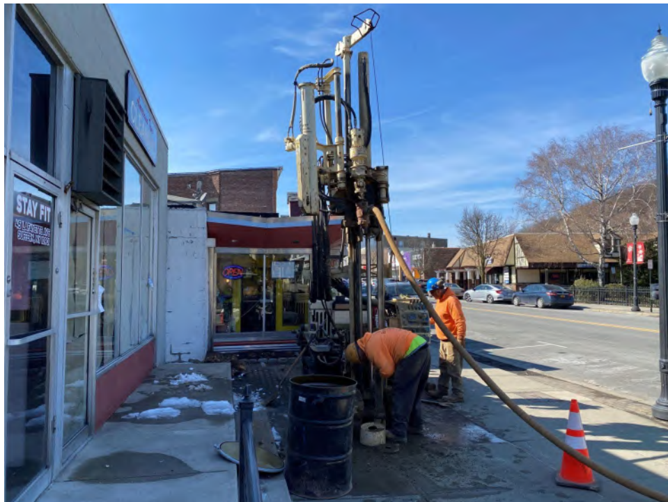
Photograph 6 – Installation of monitoring well MW-1 (along Lafayette Avenue).
