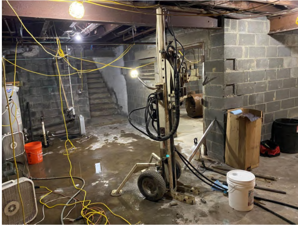
Photograph 3 – Drill unit used to advance basement soil borings.
