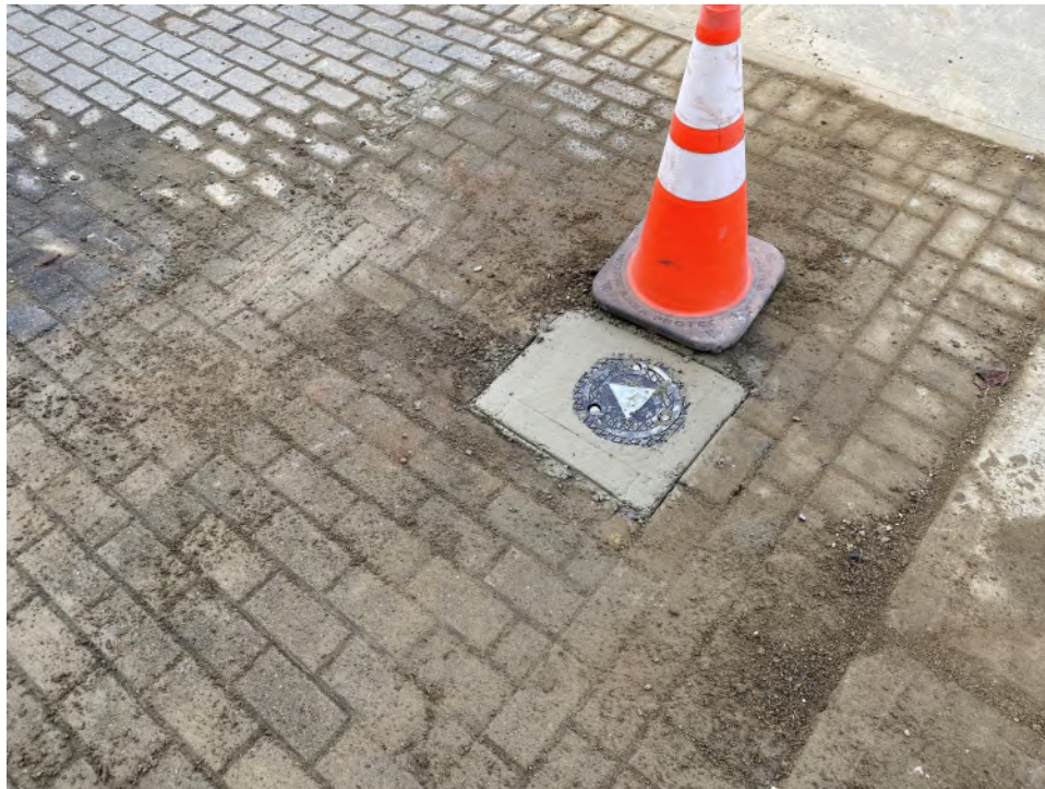
Photograph 7 – Monitoring well MW-1.
