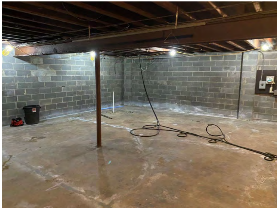
Photograph 2 – Basement work area during January 13, 2022 soil boring investigation.
