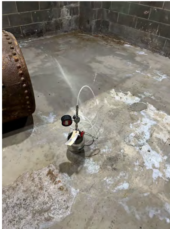
Photograph 10 – Sub-slab vapor sample collection.
