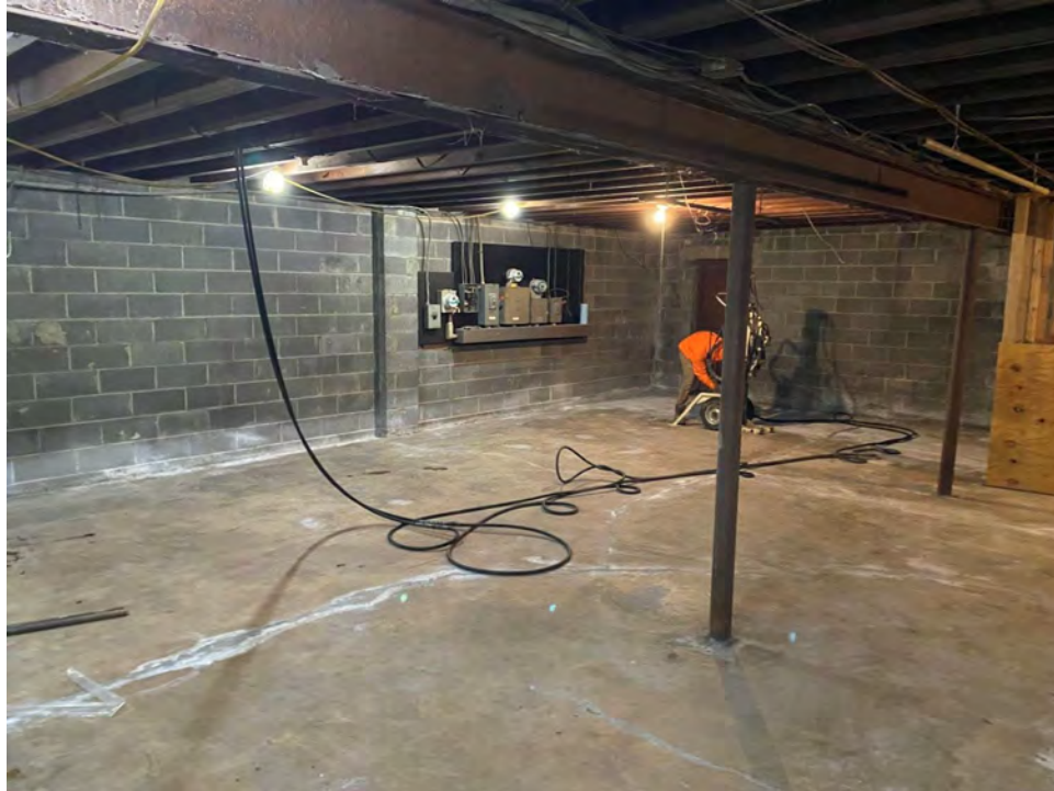
Photograph 1 – Basement work area during January 13, 2022 soil boring investigation.
