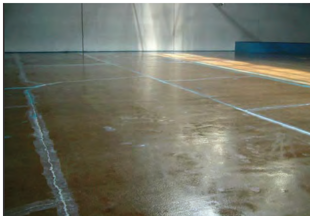
Completed surface preparation consisting of shot blasting, Retro-Coat Caulk, to fill joints and cracks and a 6 mil application of Retro-Coat Primer
