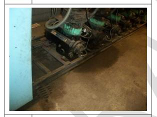
Note a floor drain in the vicinity of staining beneath the refrigeration equipment;
