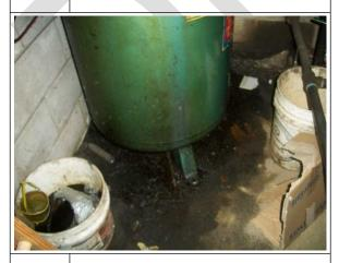
7. Staining beneath the compressor in the dry cleaning unit.
