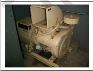
Note de minimis staining beneath one of two natural gas fired emergency generators in the Stop & Shop unit.
