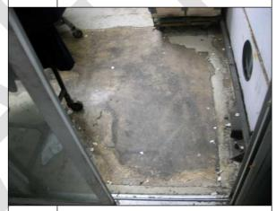
View of the floor in the dry cleaning room; note exposed concrete floor where the epoxy sealant has come off.
