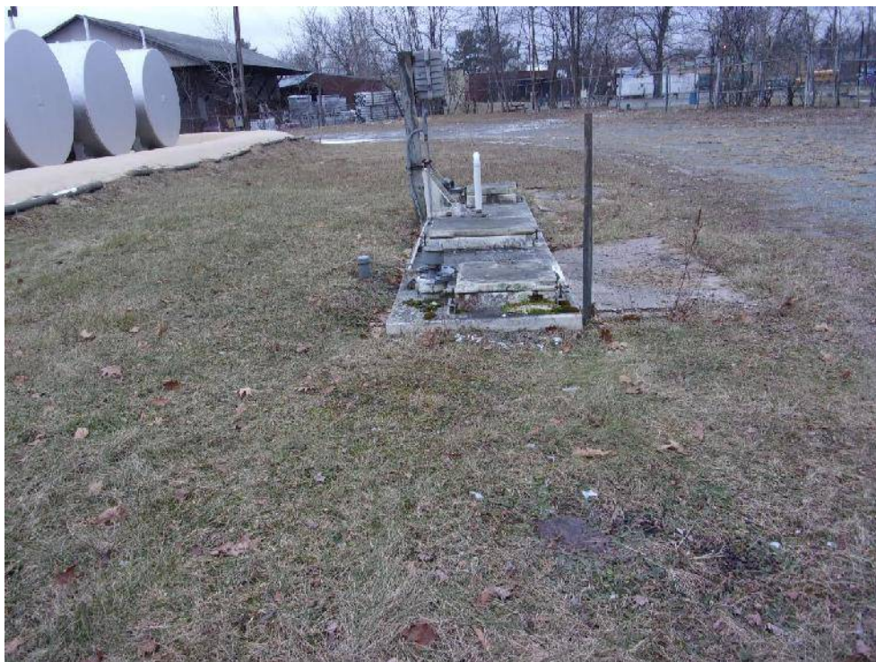
Photo A9 – Oil-water separator at the South Fallsburg terminal
