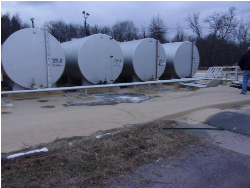
Photo A6 – Tanks 5 through 8, which are 20,000-gallon diesel and fuel oil ASTs
