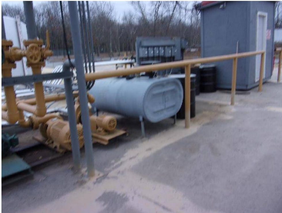
Photo A3 – 275 gallon fuel oil AST at the South Fallsburg loading rack
