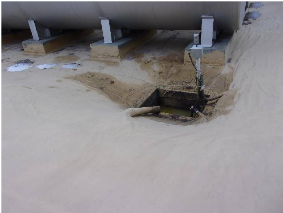
Photo A8 – Sump inside secondary containment for the 20,000-gallon ASTs
