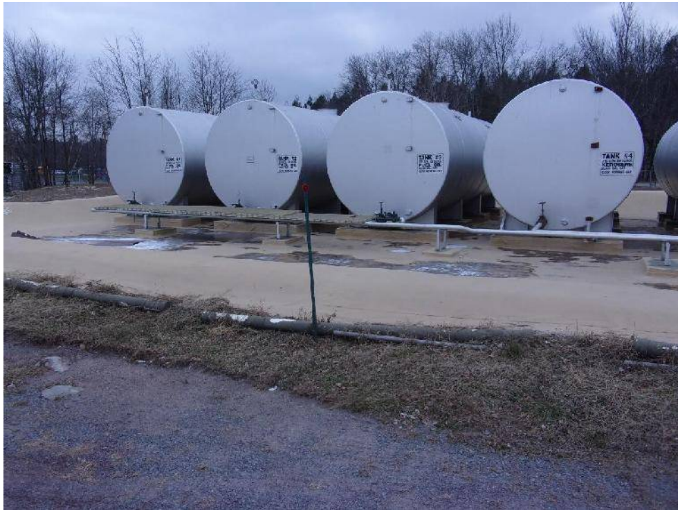
Photo A5 – Tanks 1 through 4, which are 20,000-gallon fuel oil and kerosene ASTs
