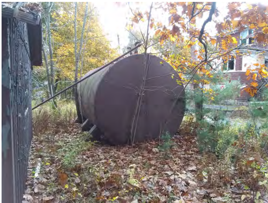
2. Large AST north of main building
