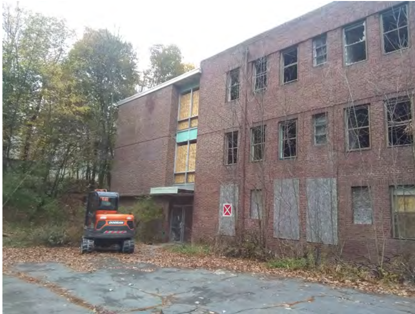
1. Location of TP-1, main building (former hospital) and excavator
