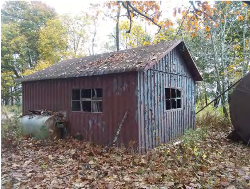
3. 275-gallon AST in vicinity of large AST
