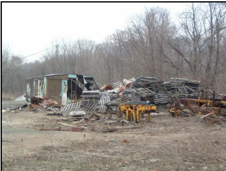
An abandoned, gutted trailer on the southern side of the Island with a construction debris pile adjacent. Large metal equipment has also been deposited here.
