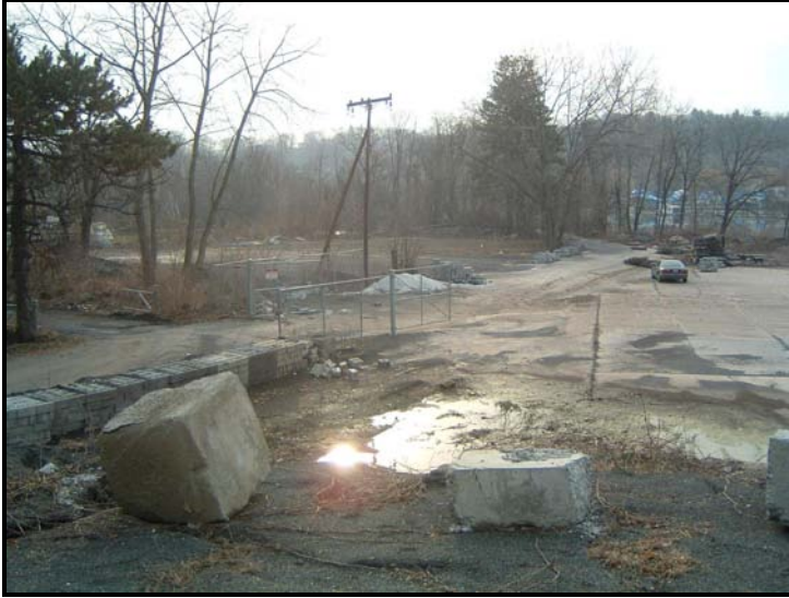
A view from Abeel Street of the gated site entrance, small parcel used for storage, and entrance to the Island.
