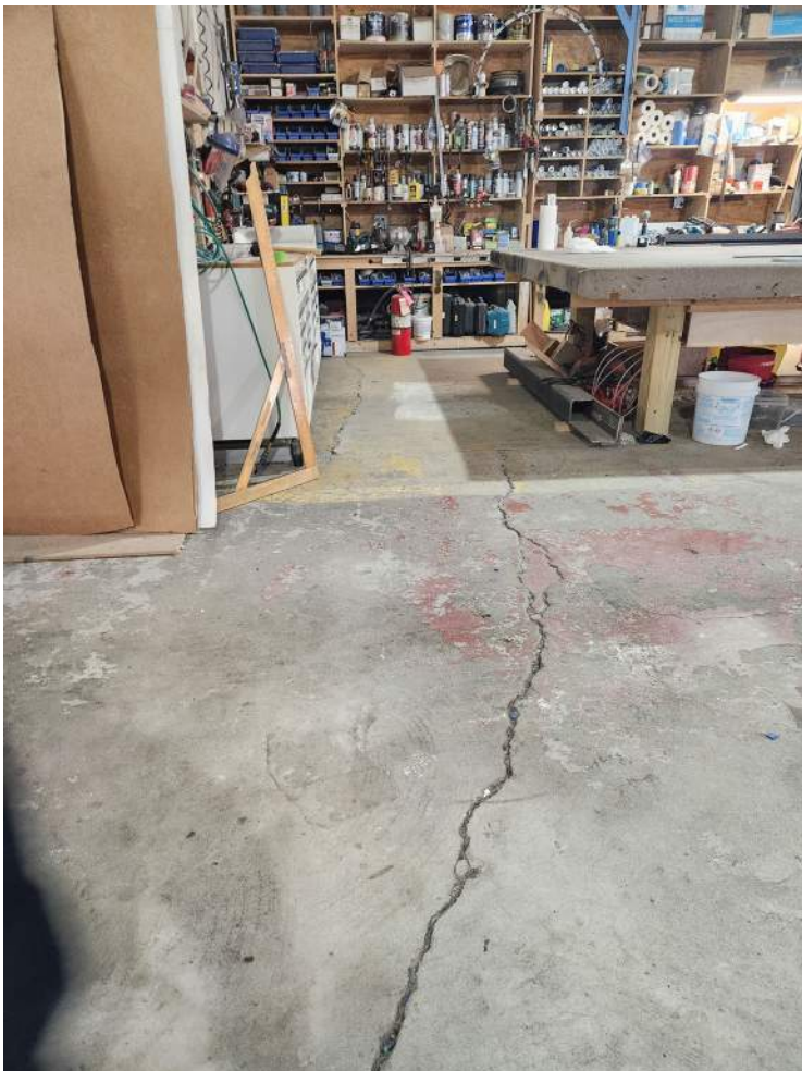
Cracks in the floor slab identified at 61 Water Street in the Mirage Glass Manufacturer.
