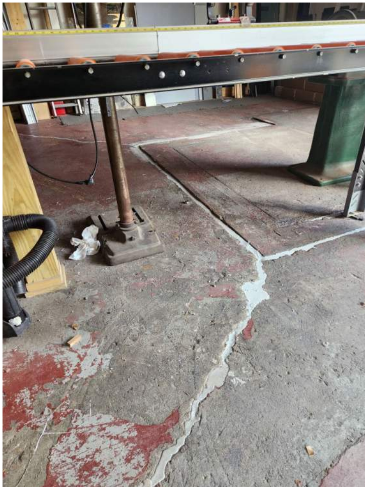
03 - Northeastern Portion of 61 Water St.
