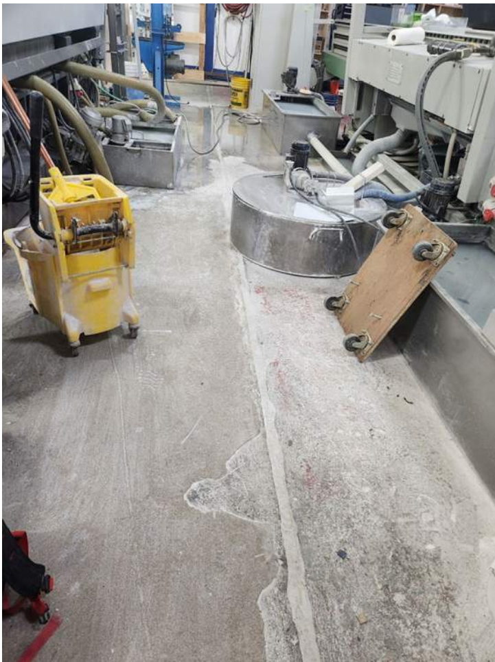
07 - Southwestern Portion of 61 Water St.
