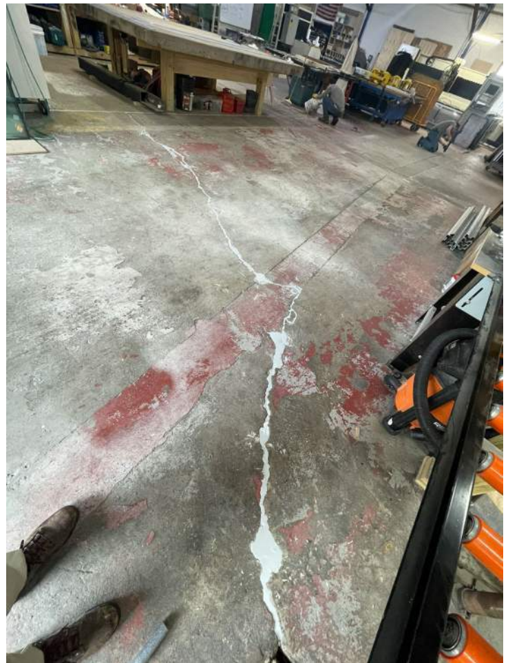
04 - Northeastern Portion of 61 Water St.
