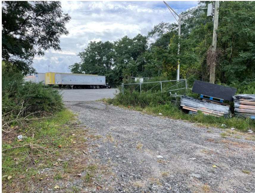
Photo 1 Site entrance from Stew Leonard Drive.
