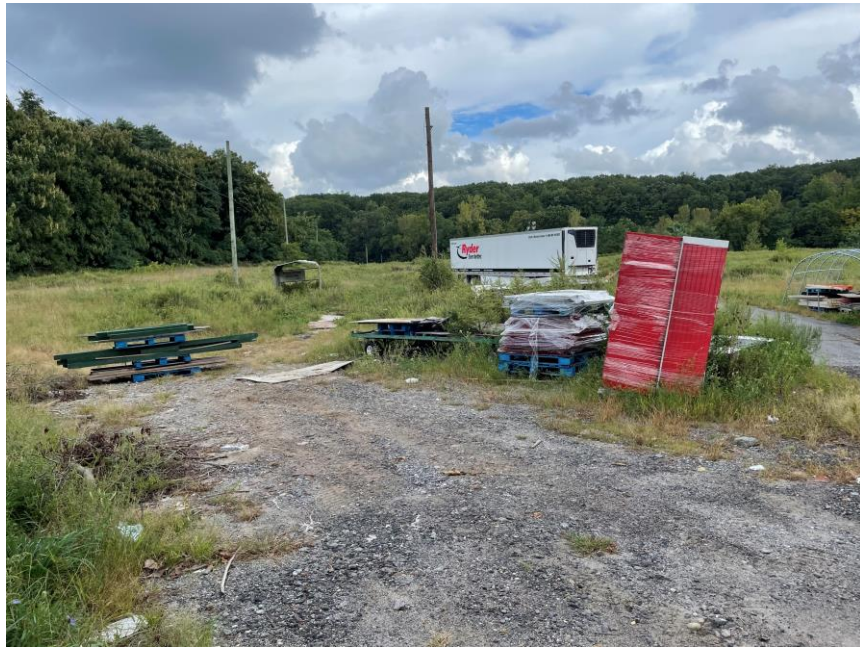
Photo 7 Typical material staging from adjacent business.
