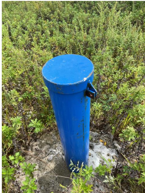
Photo 6 Piezometer installed by others during geotechnical investigation. Needs cover to be locked.
