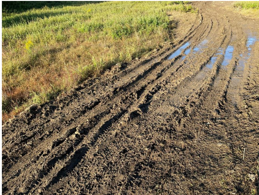
Photo 11 Typical disturbance resulting from geotechnical investigation activities. Areas will be regraded and reseeded once work is completed.
