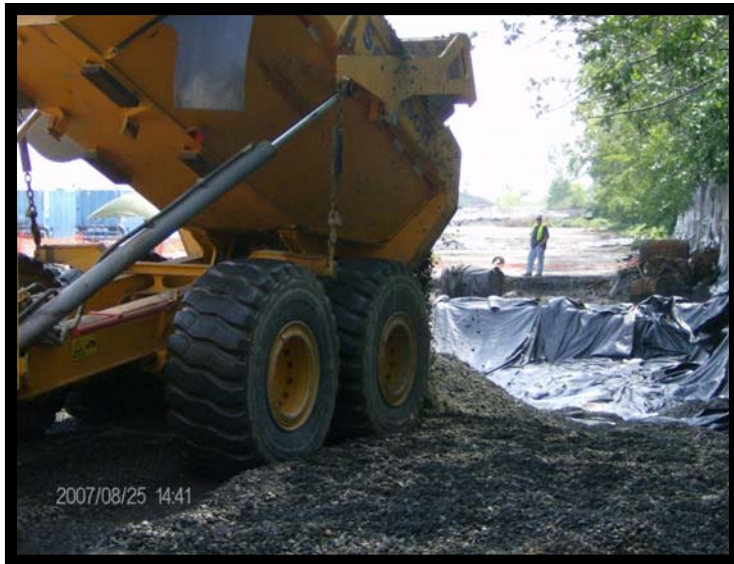
Placement of Backfill in PAOC 29
