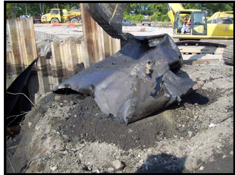
Second Additional UST Encountered in Former UST Area
