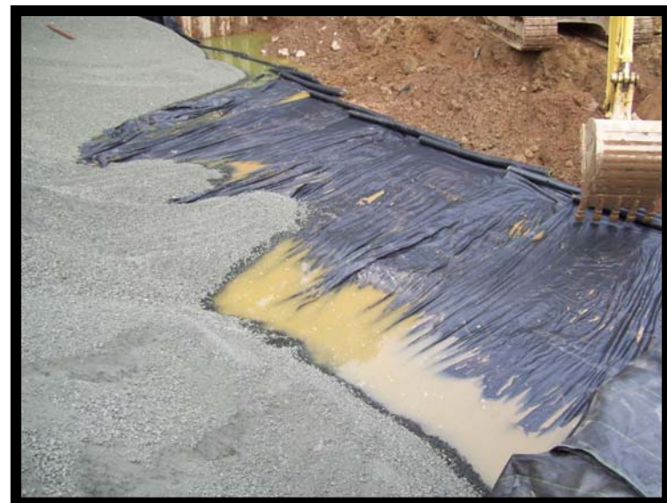
Placement of Demarcation Barrier in PAOC 47
