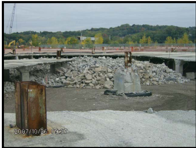
PAOC 7 Post-Restoration, Containing Consolidated Concrete Rubble
