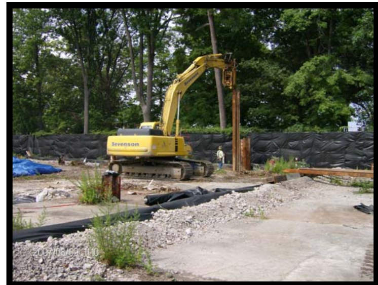
Installation of Excavation Support in PAOC 47
