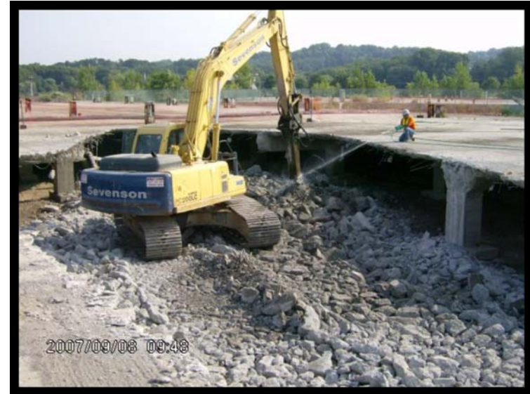
Concrete Demolition, PAOC 7
