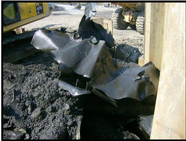
First Additional UST Encountered in Former UST Area
