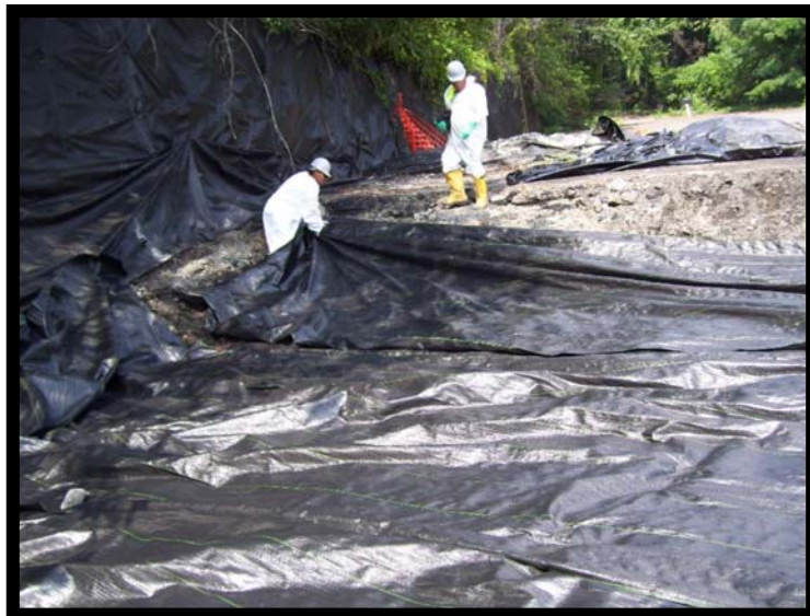
Placement of Demarcation Barrier in PAOC 29
