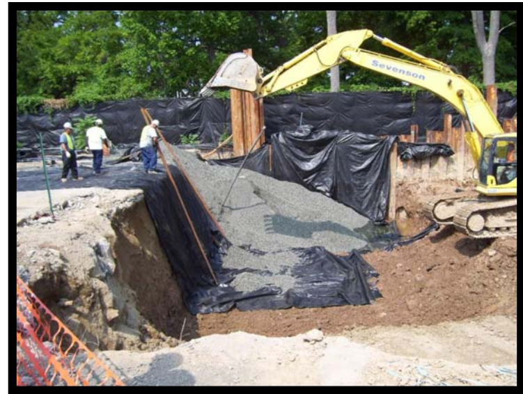
Placement of Backfill in PAOC 47
