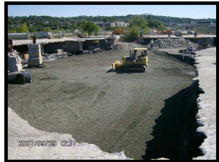
Placement of PAOC 7 Backfill
