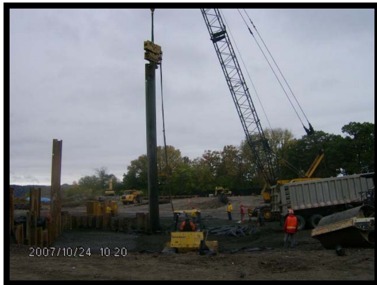
Removal of Sheet Pile from Former UST Area
