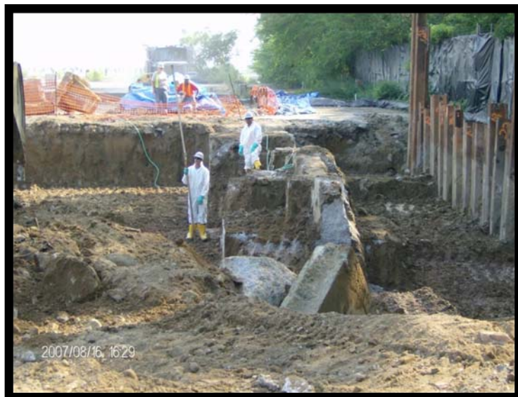
Concrete Structures Encountered During Excavation of PAOC 47
