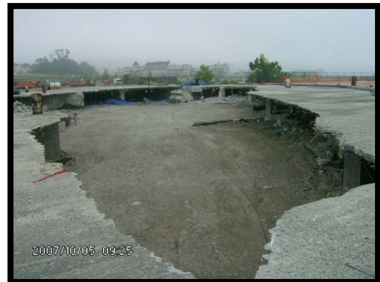
PAOC 7 Following Backfill Placement
