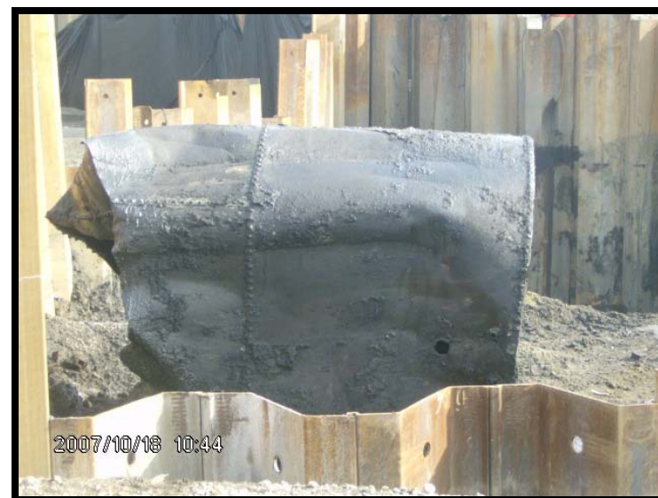
Removed Remnant of 10,000 Gal UST
