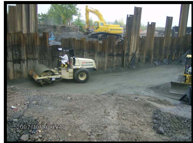
Compaction of Backfill in Former UST Area
