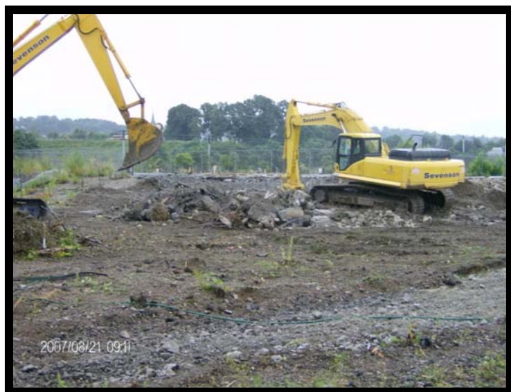
Removal of Concrete Foundation in Former UST Area
