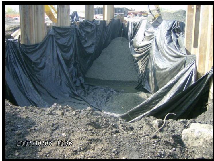
Placement of Demarcation Barrier in Former UST Area
