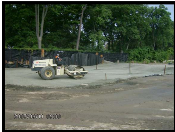
Compaction of Backfill in PAOC 47
