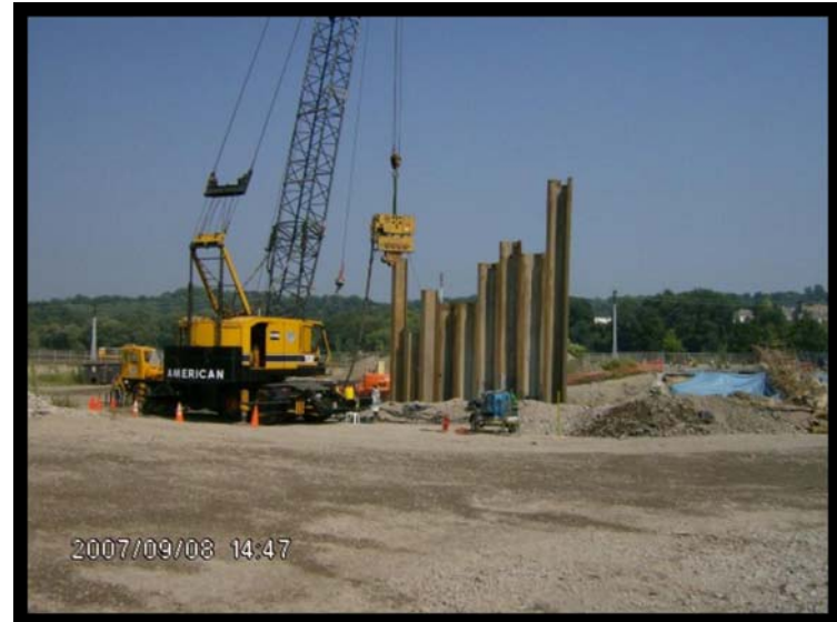
Installation of Excavation Support in the Former UST Area
