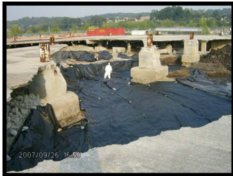
Placement of Demarcation Barrier, PAOC 7
