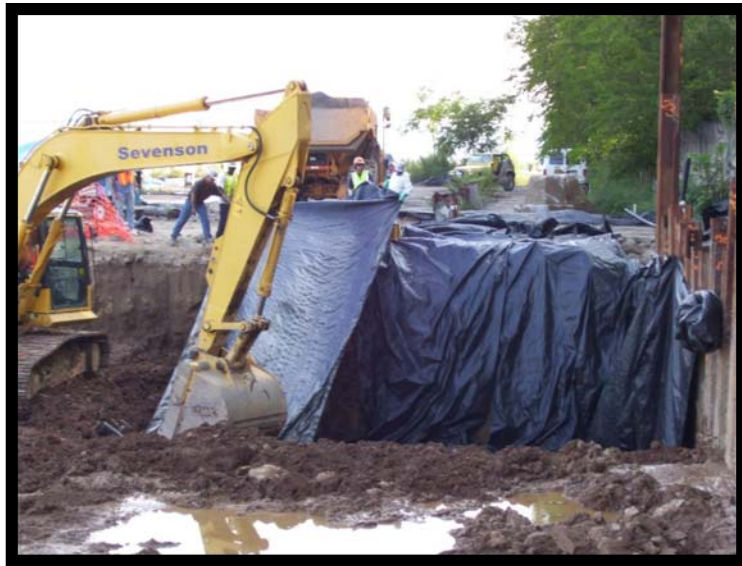
Placement of Demarcation Barrier in PAOC 47
