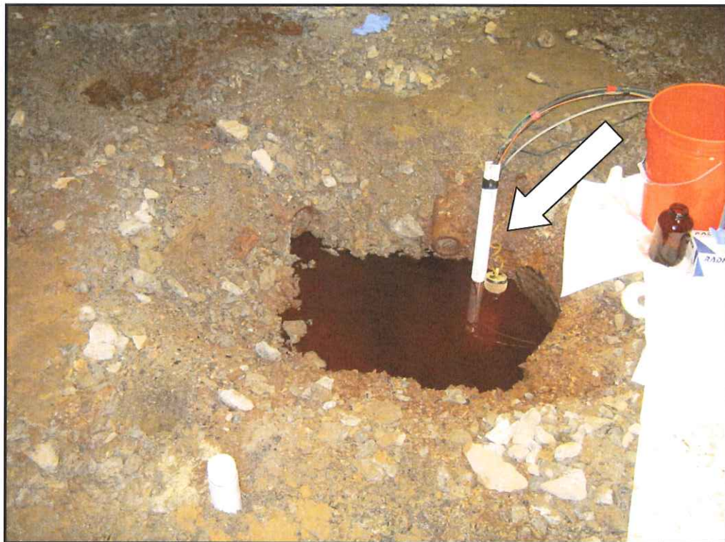
149 North Avenue – Petroleum Product within Sump (Note: Dewatering Point and Product Only Skimmer Pump)
