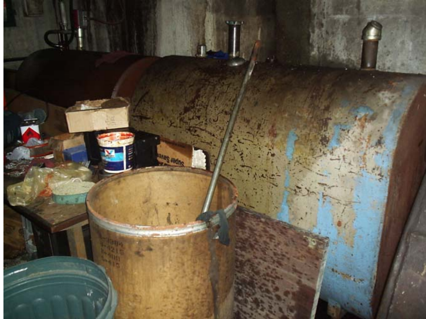
Photograph 9: Waste Antifreeze Tanks
