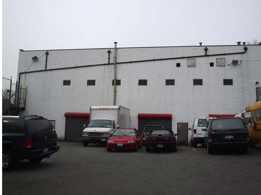
Photograph 3: East Side of the Building and Asphalt Yard
