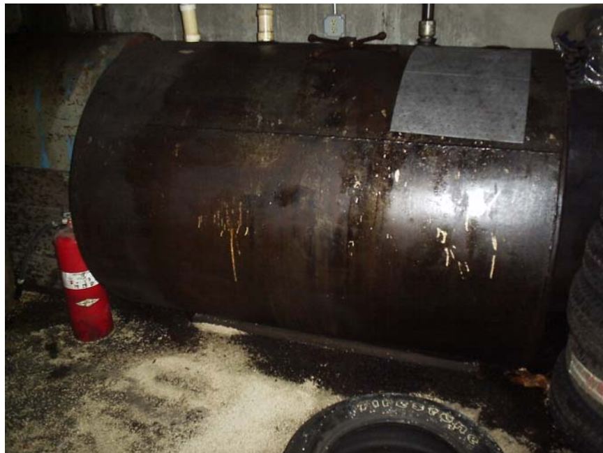
Photograph 10: Waste Oil Tank
