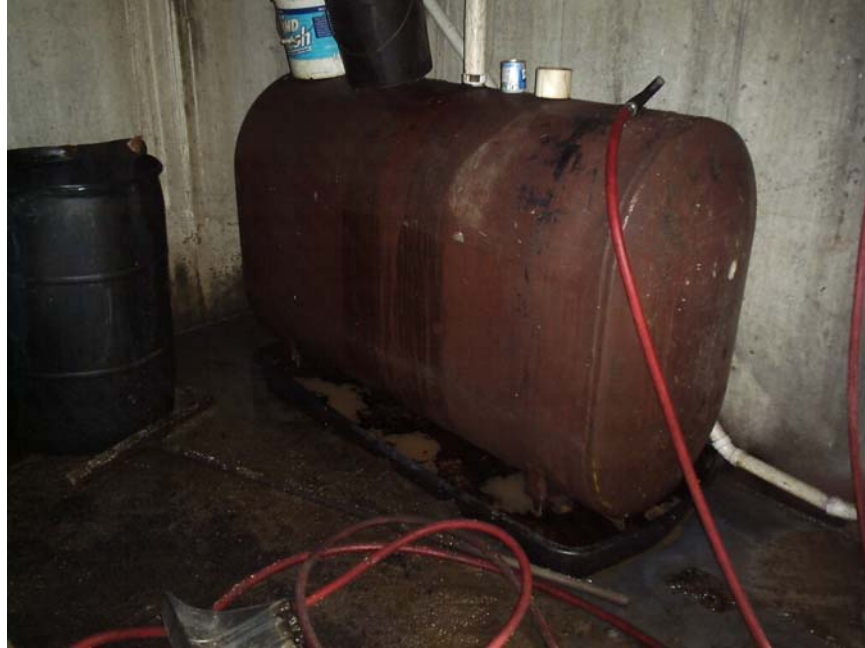
Photograph 11: Waste Water Tank
