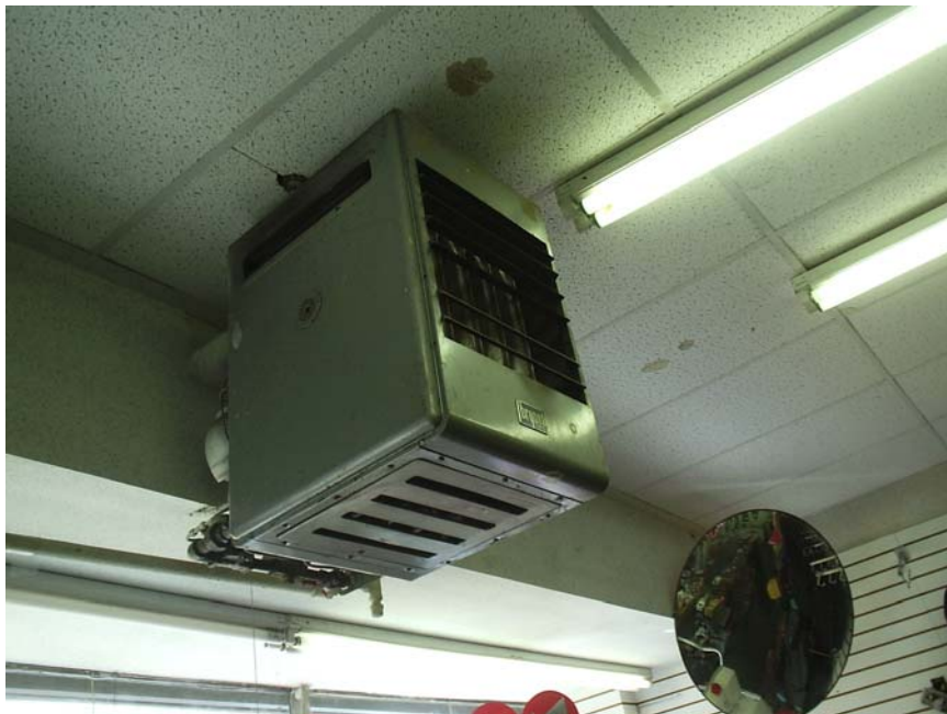
Photograph 6: Overhead Natural Gas Fired Heating Equipment
