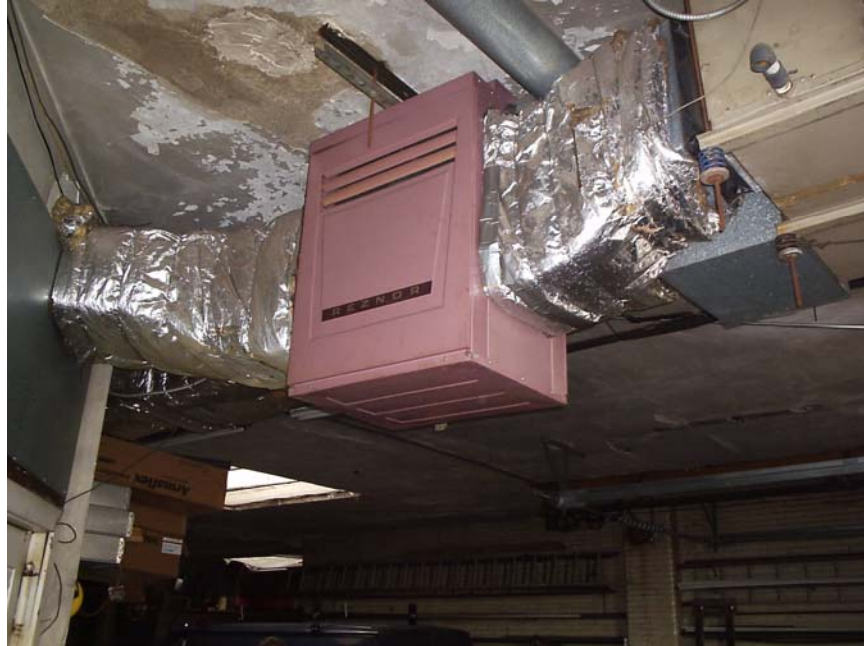
Photograph 7: Overhead Natural Gas Fired Heating Equipment
