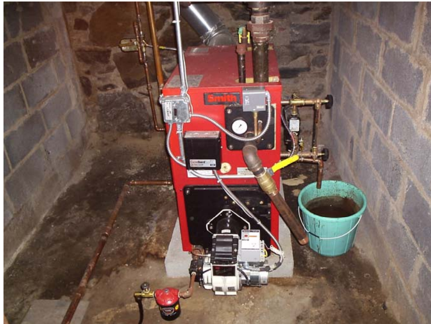
Photograph 4: Fuel Oil Fired Heating Equipment, 131 New Main Street
