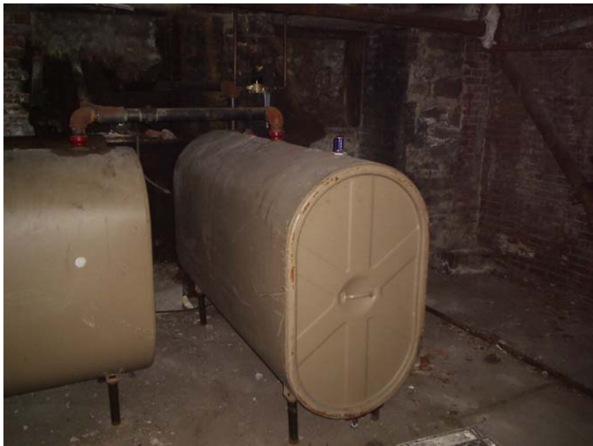
Photograph 6: Aboveground Fuel Oil Storage Tanks at 127-129 New Main Street
