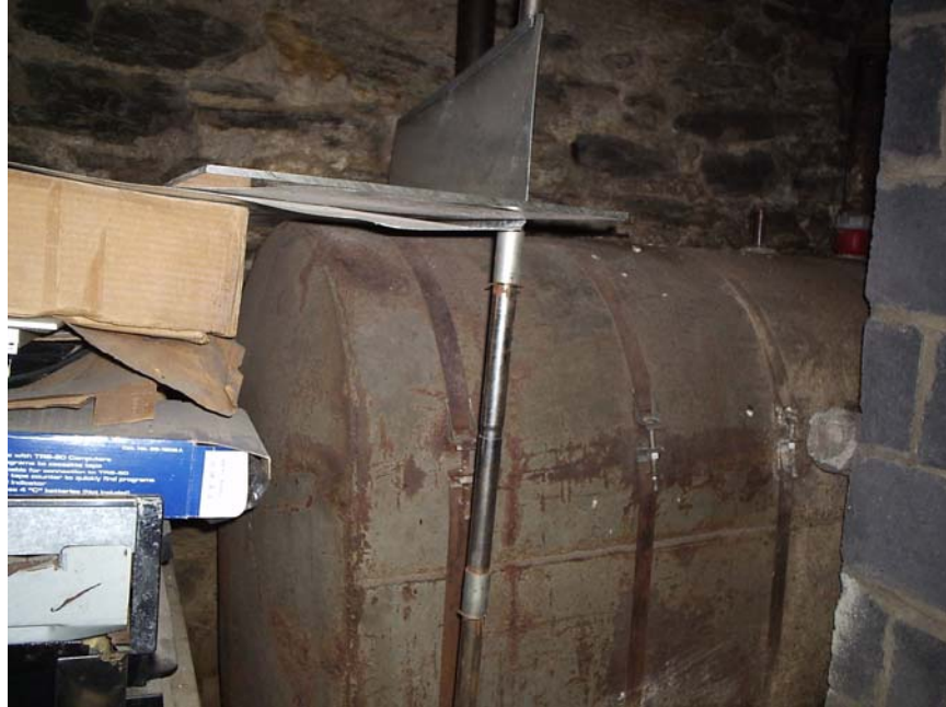
Photograph 7: Aboveground Fuel Oil Storage Tank at 131 New Main Street
