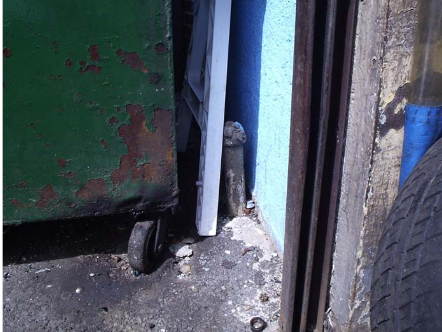
Photograph 11: Vent Pipe for Suspect Underground Storage Tank
