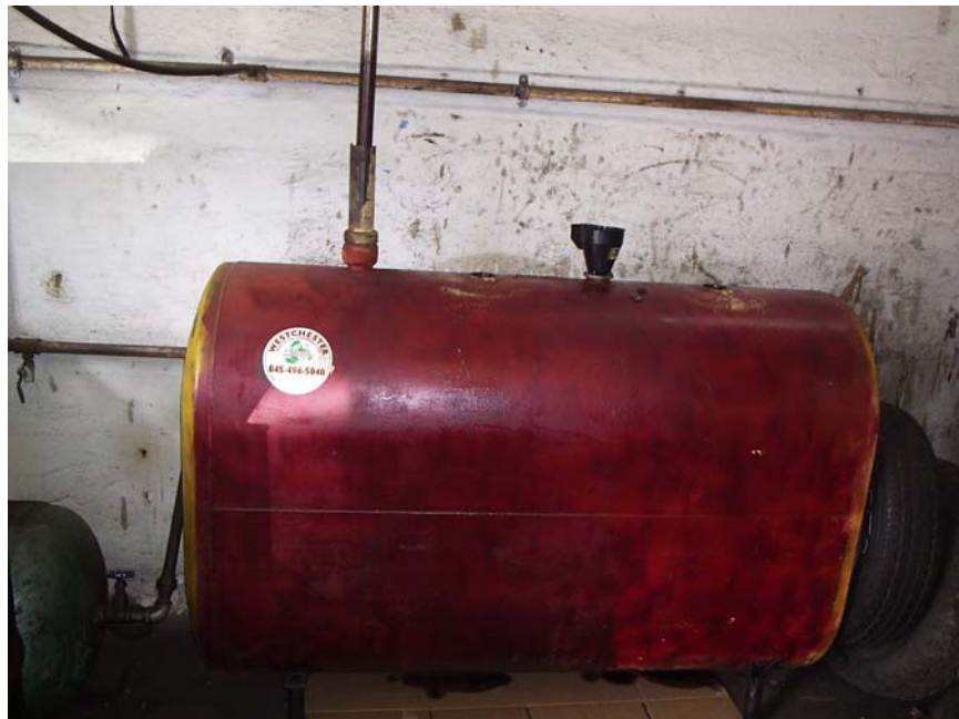
Photograph 10: Aboveground Waste Oil Storage Tank
