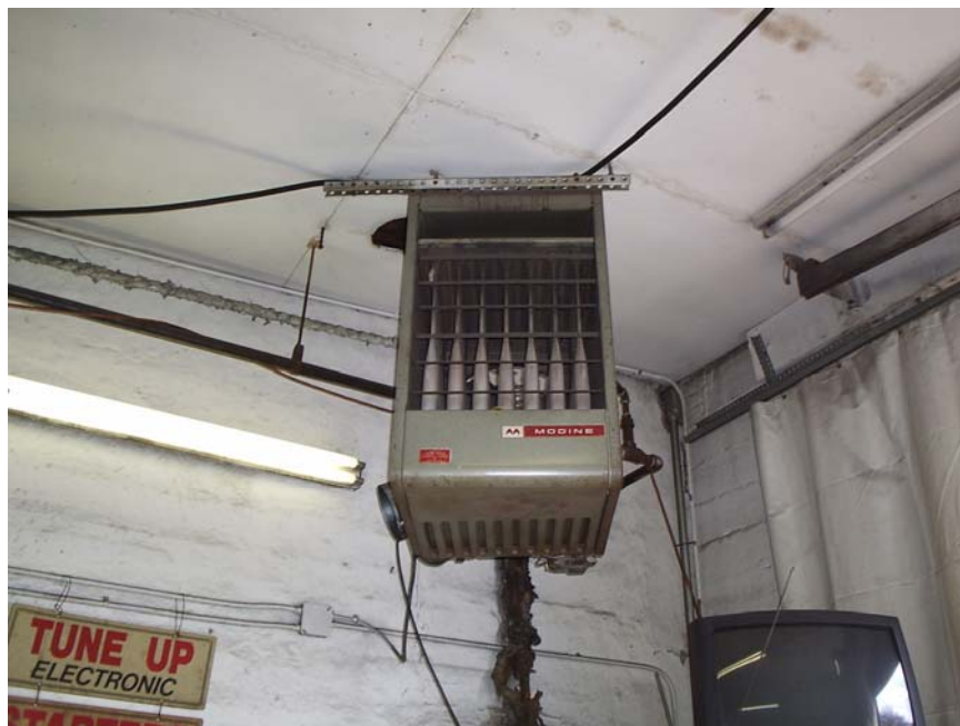
Photograph 2: Overhead Natural Gas Fired Heating Equipment, Typical
