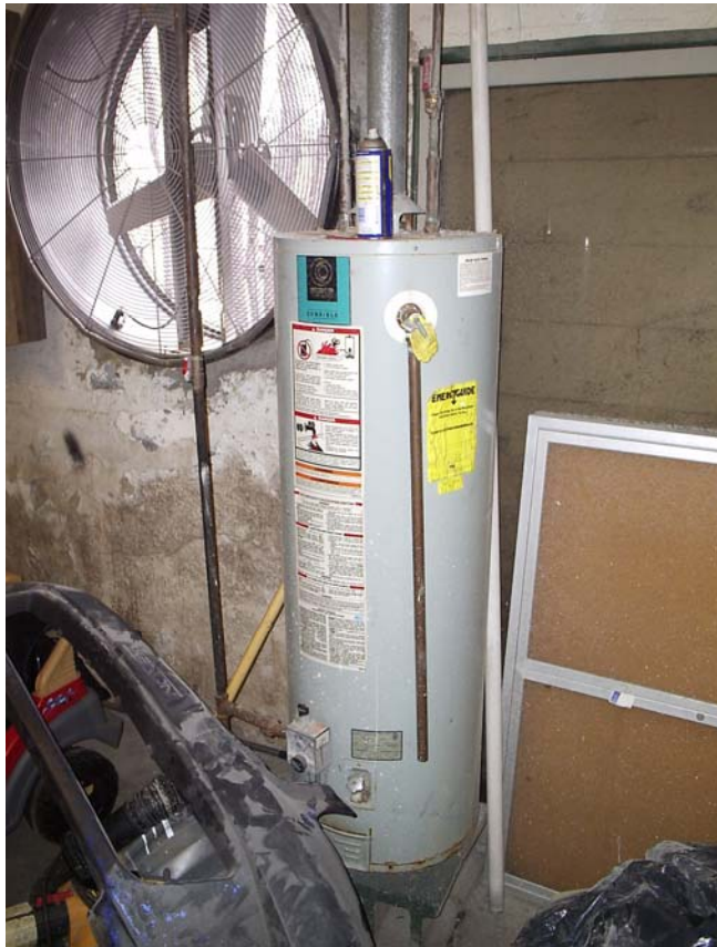
Photograph 3: Natural Gas Fired Hot Water Heating Equipment
