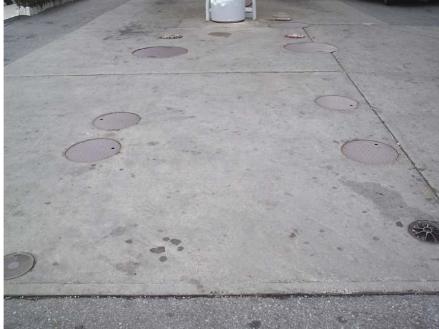
Photograph 9: Concrete Tank Pad for Underground Gasoline Storage Tanks
