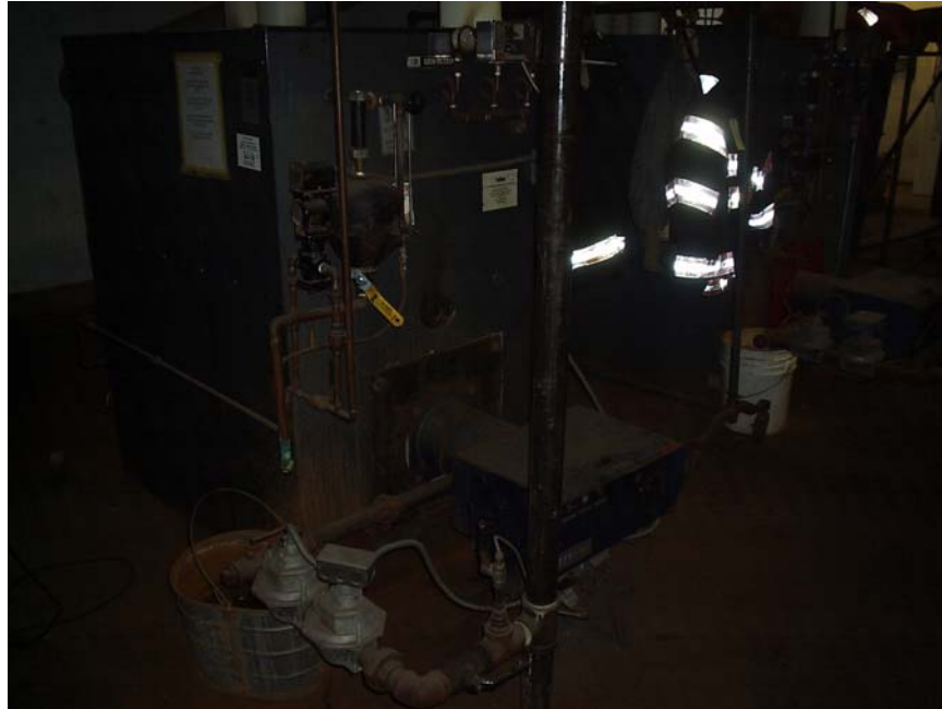
Photograph 6: Natural Gas Fired Heating Equipment
