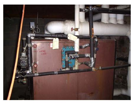
Photograph 4: Fuel Oil Fired Heating Equipment at 193 Nepperhan Avenue
