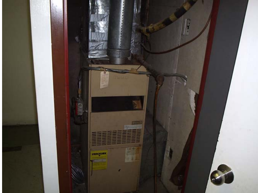
Photograph 5: Natural Gas Fired Heating Equipment
