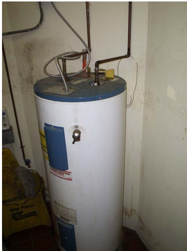
Photograph 6: Electrical Hot Water Heater
