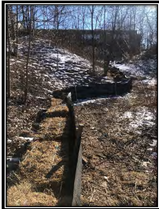
Photograph of silt fencing along Central/ Western and eastern Track 2 boundary (looking north)
