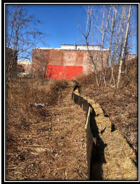
Photograph of silt fencing along Central/ Western and eastern Track 2 boundary (looking north)
