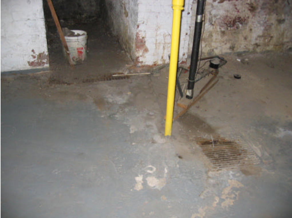
Photograph No. 8: Two floor drains within northeastern portion of the basement.
