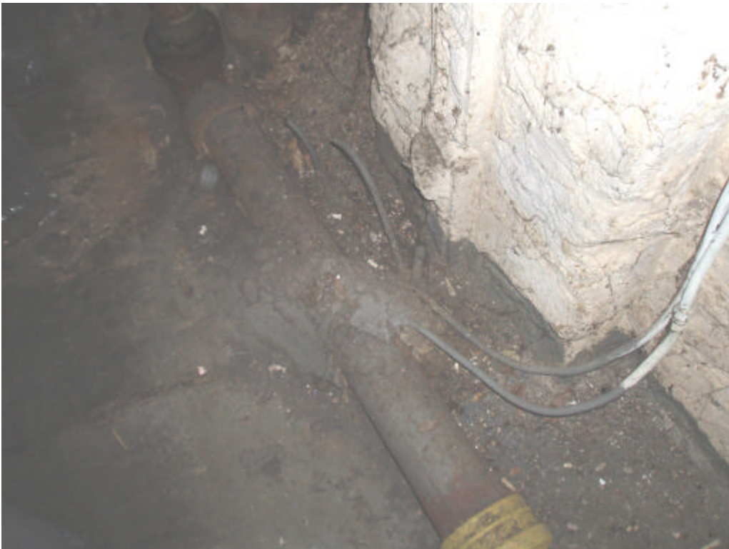
Photograph No. 5: Cut copper lines within basement.
