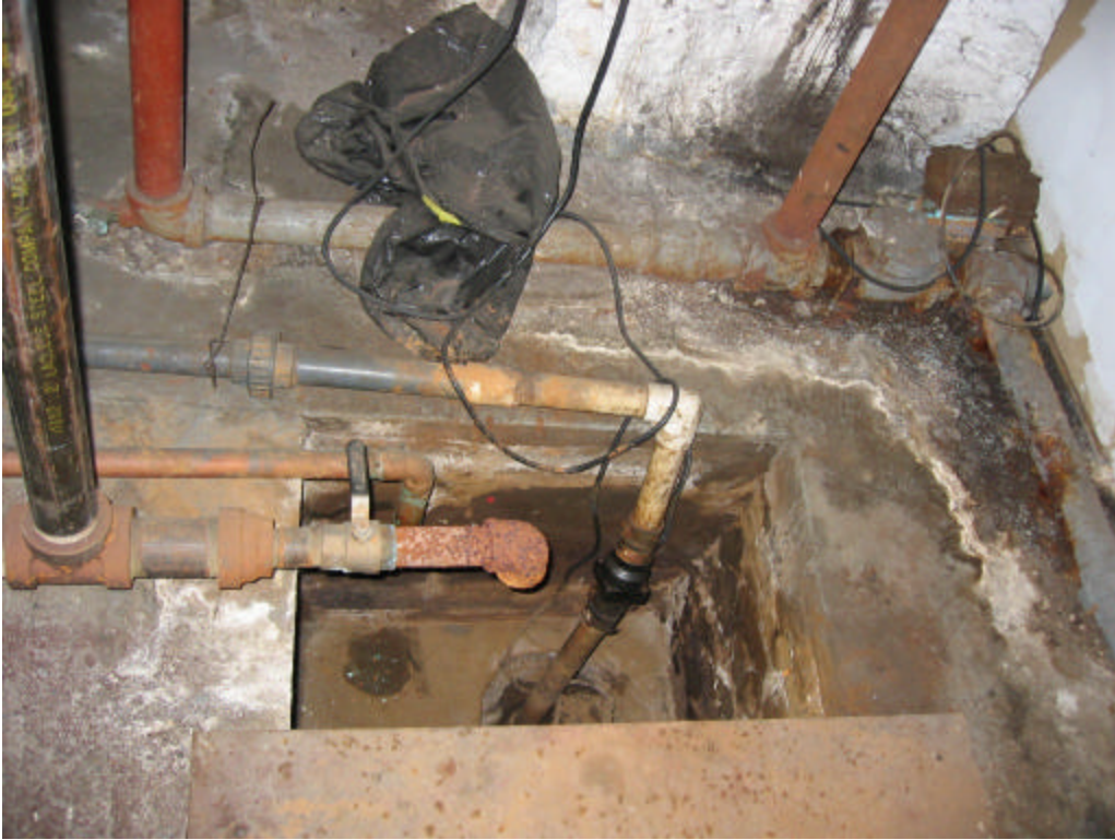
Photograph No. 6: Sump pit within boiler room.
