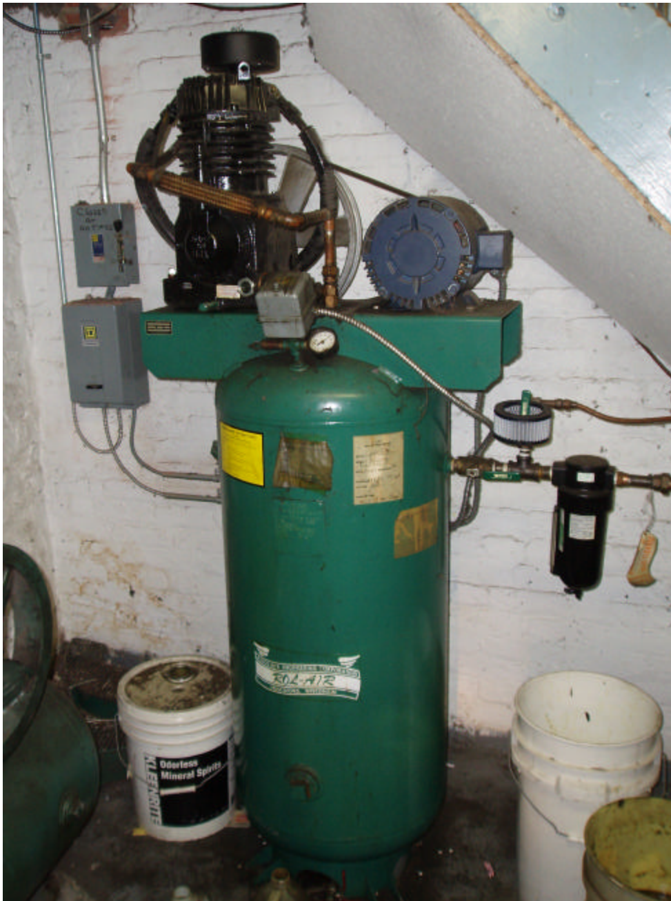
Photograph No. 3: Air compressor located within the basement.
