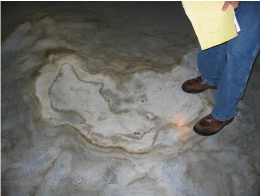
Photograph No. 7: Water staining and hole within slab floor of the basement.
