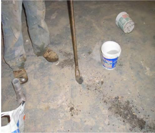
Hand installation of permanent vapor point
