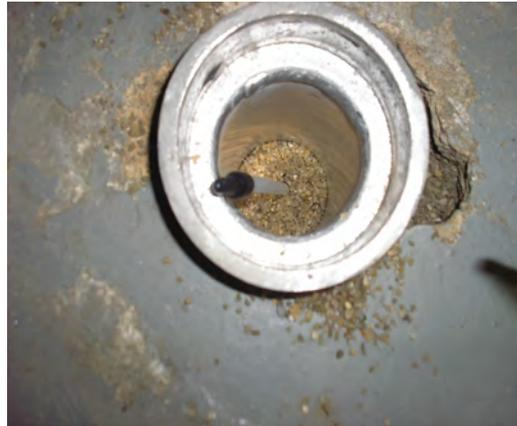
Installed permanent vapor point with gravel pack
