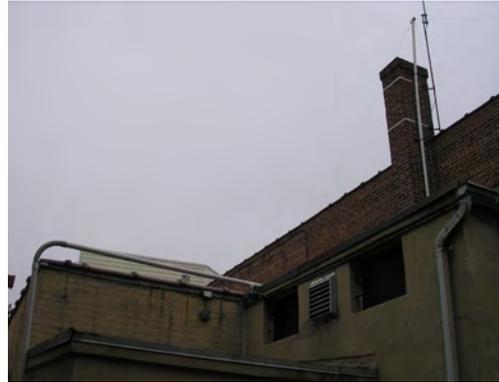
SVE/SSDS exhaust piping to 10' above roof line
