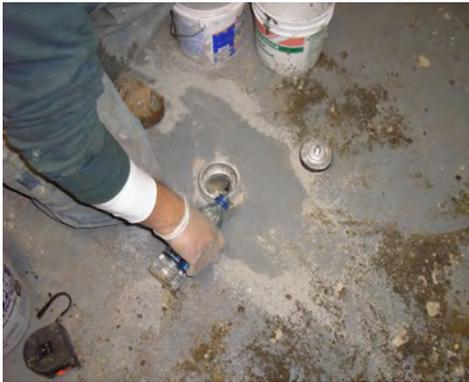
Hydrating bentonite to assure proper seal
