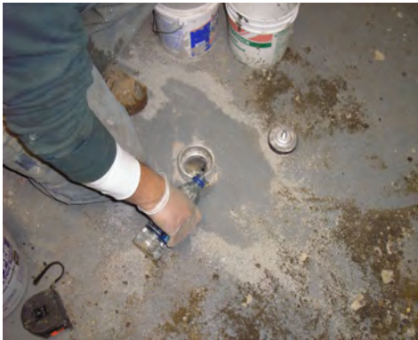
Hydrating bentonite to assure proper seal
