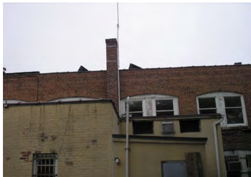
SVE/SSDS exhaust piping to 10' above roof line
