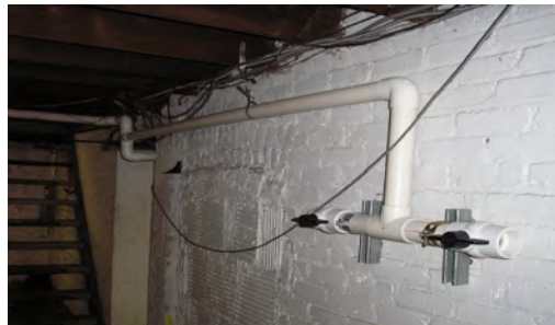
Basement piping manifold for each for North and South basement trenching
