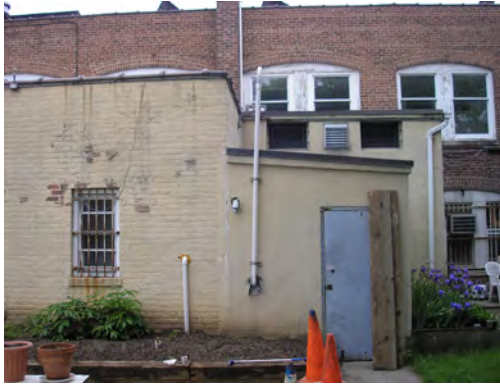
SVE/SSDS exhaust piping to 10' above roof line
