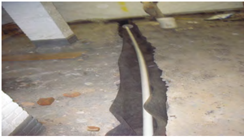
Trenching for SSDS in Basement of Schmukler's Cleaners
