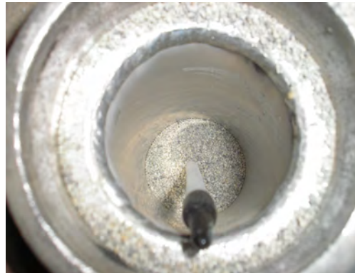
Hydrating bentonite to assure proper seal
