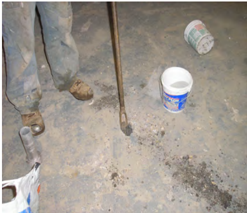
Hand installation of permanent vapor point
