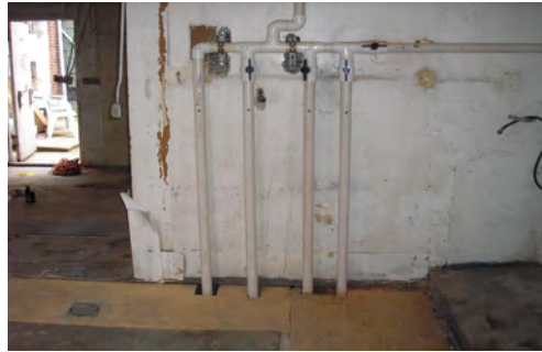
Installation of manifold for all SVE wells and SSDS
