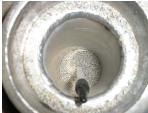
Hydrating bentonite to assure proper seal
