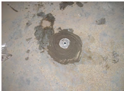
Finished permanent vapor point sealed to grade surface
