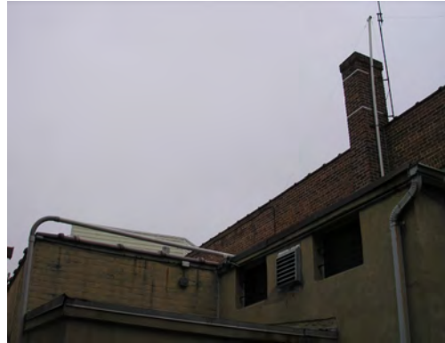
SVE/SSDS exhaust piping to 10' above roof line
