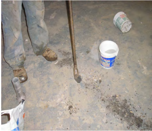
Hand installation of permanent vapor point
