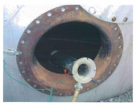
Photograph 2. Ventilation of Aboveground Storage Tank
