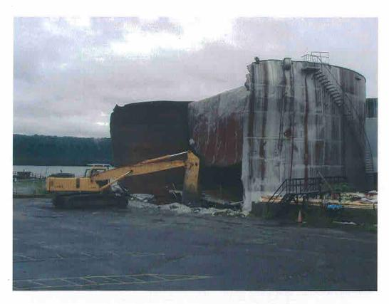
Photograph 5a. Partial Demolition of AST #2
