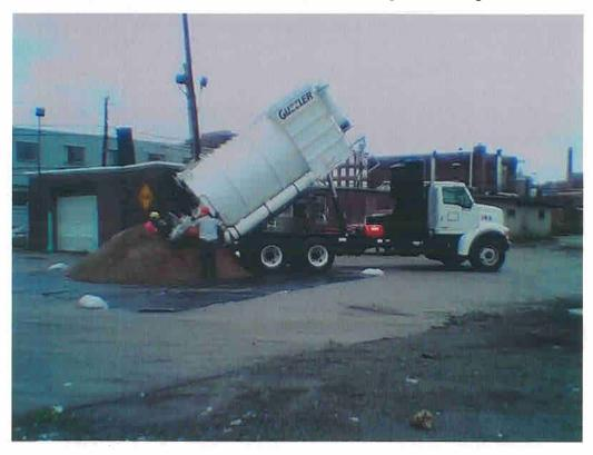
Photograph 14. Temporary Placement of Contaminated Sand in Northeast Property Corner from AST #1 False Bottom
