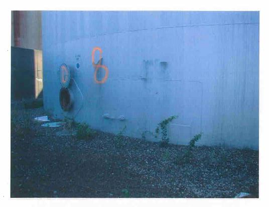
Photograph 3. Rectangular and Horizontal Welding Marks along AST #8
