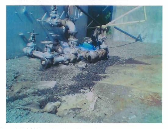
Photograph 10. Spill #2: Number 2 Oil Leak from Broken Piping Along Eastern Side of AST #4
