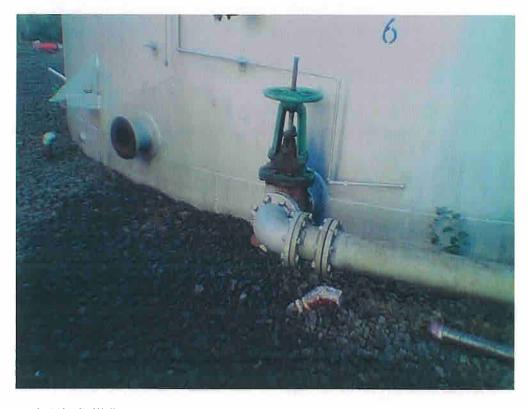
Photograph 11b. Spill #3: Number 2 Oil Leak from Broken Piping Along Western Side of AST #6
