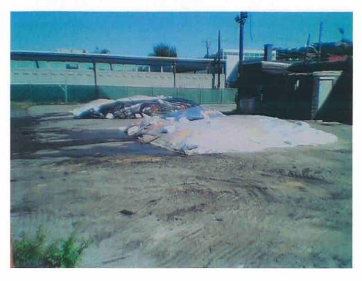
Photograph 16. Piles of All Unconsolidated Contaminated Material from ASTs #1, #4, #8 False Bottoms and from Vapor Recovery System
