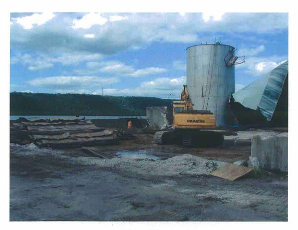
Photograph 6. Folded AST Sections Prepared for Removal and Disposal
