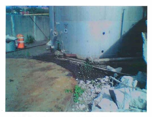
Photograph 11a. Spill #3: Number 2 Oil Leak from Broken Piping Along Western Side of AST #6
