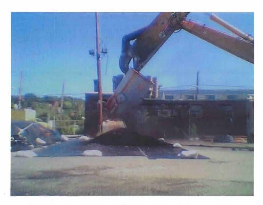
Photograph 15. Placement of Contaminated Charcoal in Northeast Property Corner from Vapor Recovery System
