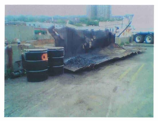
Photograph 13. Containment of Contaminated Gravel from Spill #1 in 55-gallon Metal Drums
