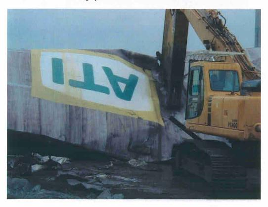
Photograph 5b. Folding and Shearing of AST #2 Sections
