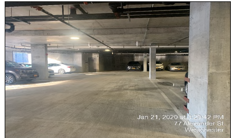
Photograph 12: The southeastern portion of the parking garage (looking north).
