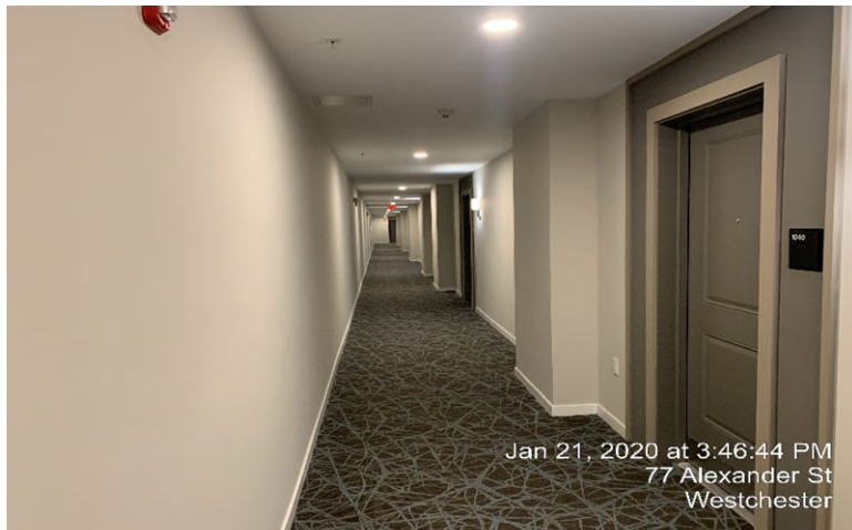
Photograph 19: View of the first floor hallway in the eastern portion of the Site.
