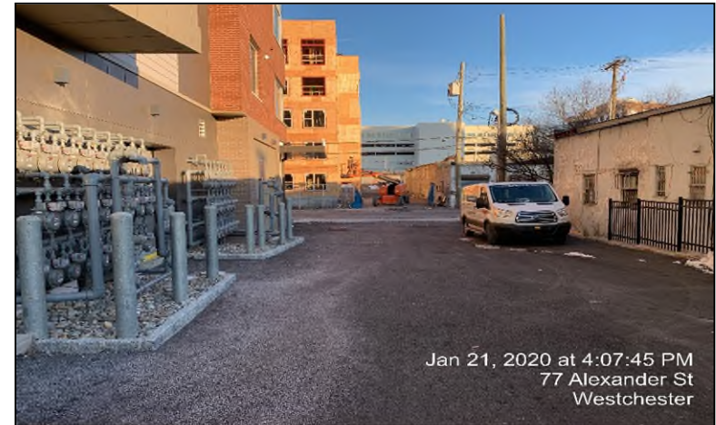
Photograph 10: Asphalt-paved area on the southeastern portion of the Site.
