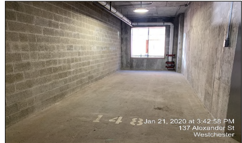
Photograph 14: Parking space in the northwestern portion of the parking garage.
