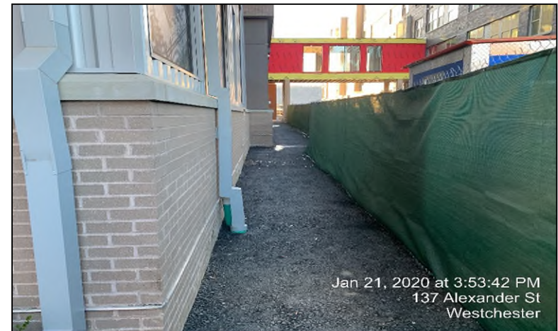
Photograph 4: The northern portion of the Site (looking west).
