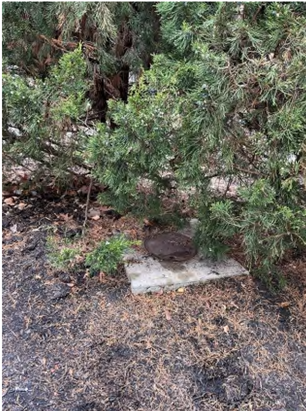
Recovery Well RW-C1
