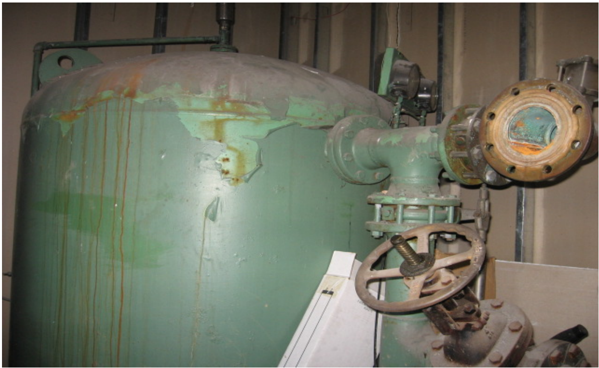
Photograph No. 15 View of an approximate 3,000 gallon boiler that is disconnected and located in the boiler room of the Stanlou Wholesale building.
