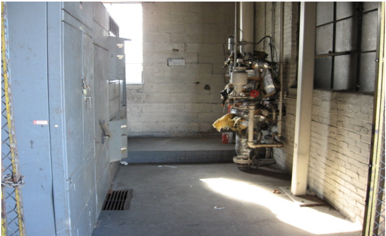
Photograph No. 21 View of air compressor, water main and floor drain located in the southwestern portion of the building located at 86 Alexander Street.
