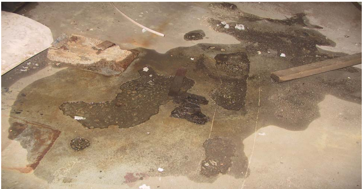
Photograph No. 12 View of water stains and cracks within the concrete floor of the northern room of the former Polychrome building located at 94 Alexander Street.
