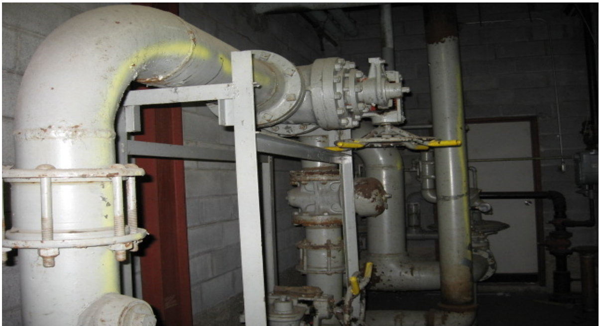
Photograph No. 16 View of rotary positive gas meter blower located in a mechanical room in the northwestern portion of the Stanlou Wholesale building.
