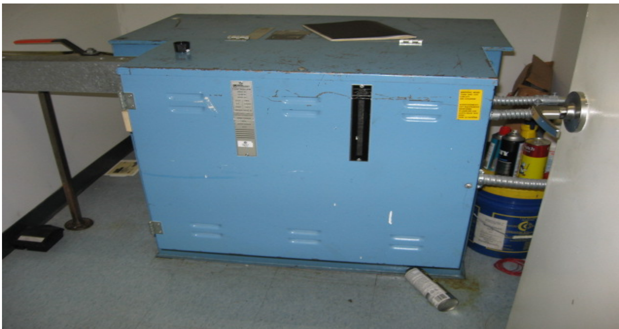
Photograph No. 6 View of elevator hydraulic motor and associated maintenance supplies contained in room adjacent to the elevator on the first floor of the WCDSS building.
