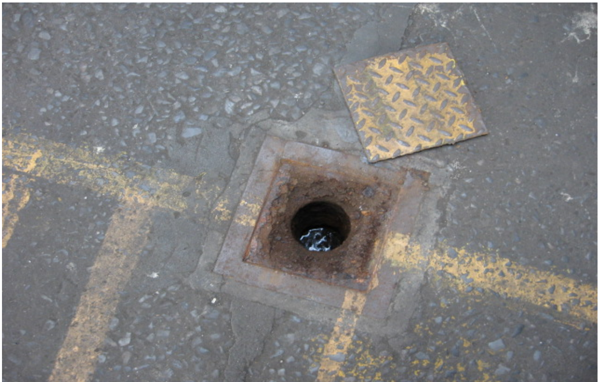
Photograph No. 23 View of a floor drain with standing water located in the central portion of the building located at 86 Alexander Street.
