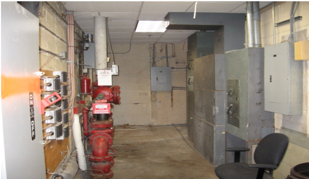
Photograph No. 9 View of a floor access area, water sprinkler main and electrical power switch panels in the mechanical room located in the southeastern portion of the WCDSS building. Apparent water stains are visible on the central portion of concrete floor.
