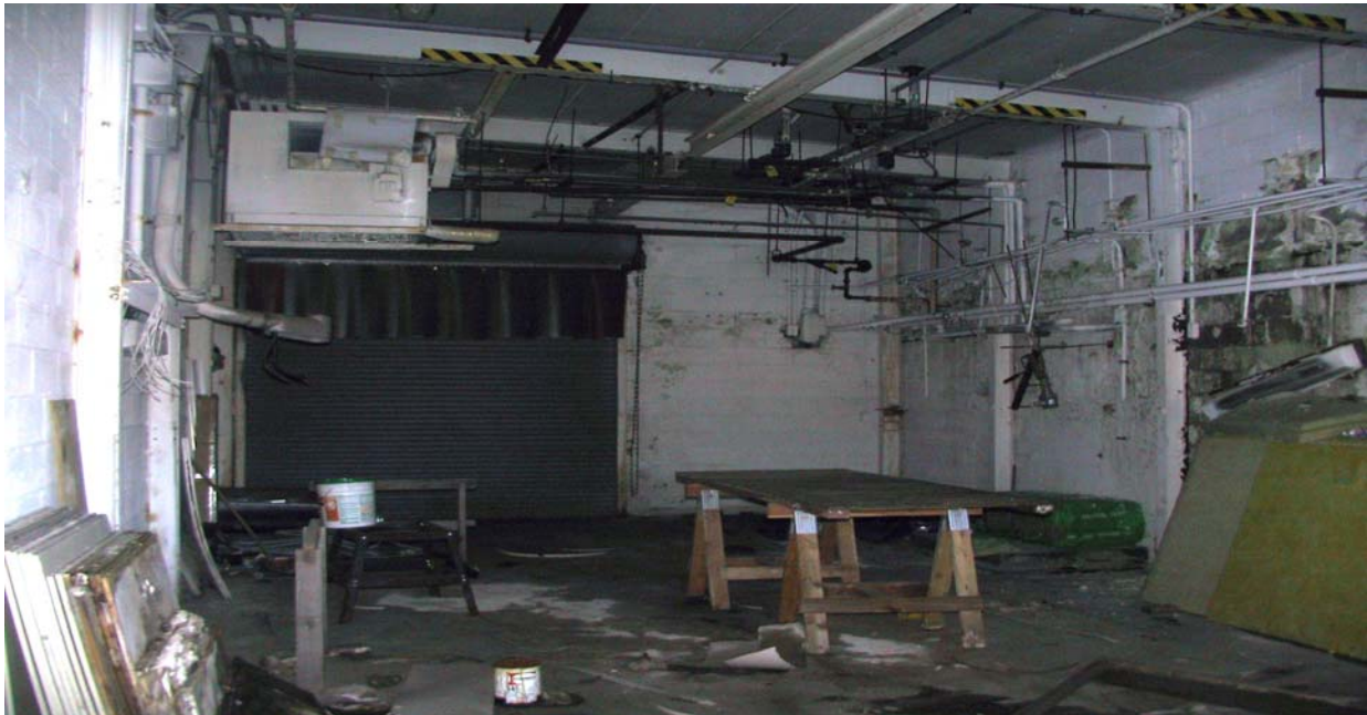
Photograph No. 11 View of northern room of the former Polychrome building located at 94 Alexander Street. Note water stains, peeling paint and mold visible on walls.
