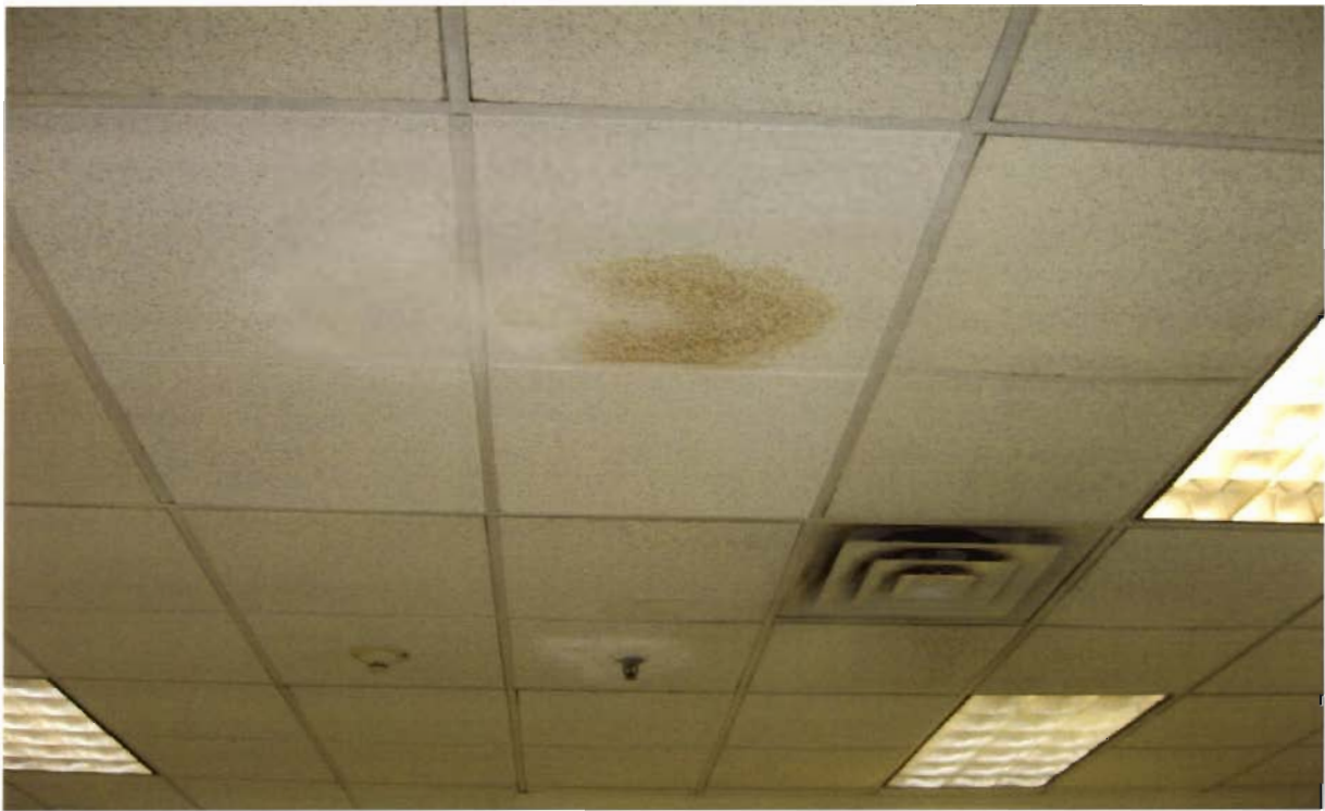
Photograph No. 7 View of water stain on ceiling tile of an office area located on the first floor of the WCDSS building.
