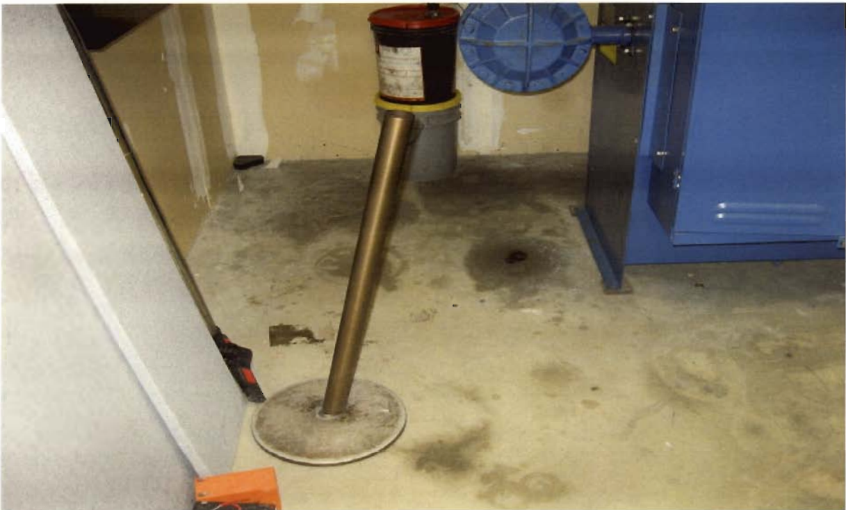
Photograph No. 8 View of oil stains on concrete floor of a mechanical room located in the northeastern portion of the WCDSS building.
