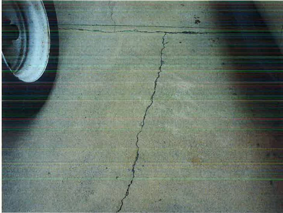
Photograph 7: More minor cracks observed in concrete surface of 441 Waverly Avenue.
