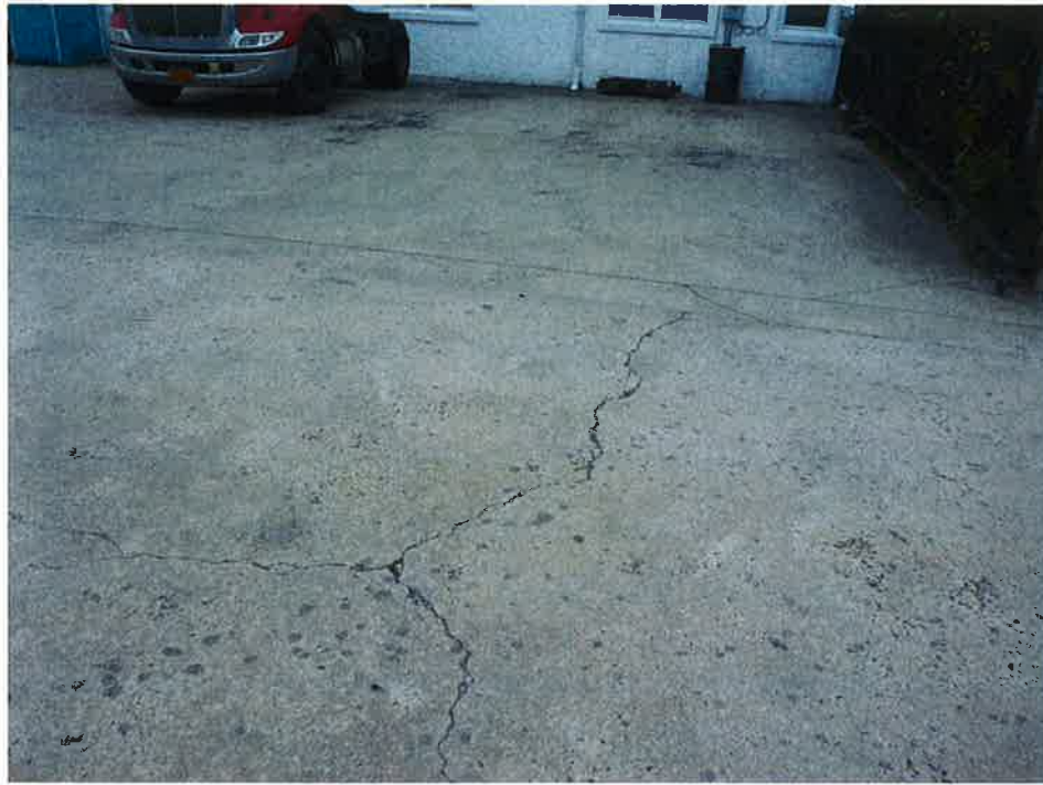
Photograph 9: Additional minor cracks observed in concrete surface of 441 Waverly Avenue.
