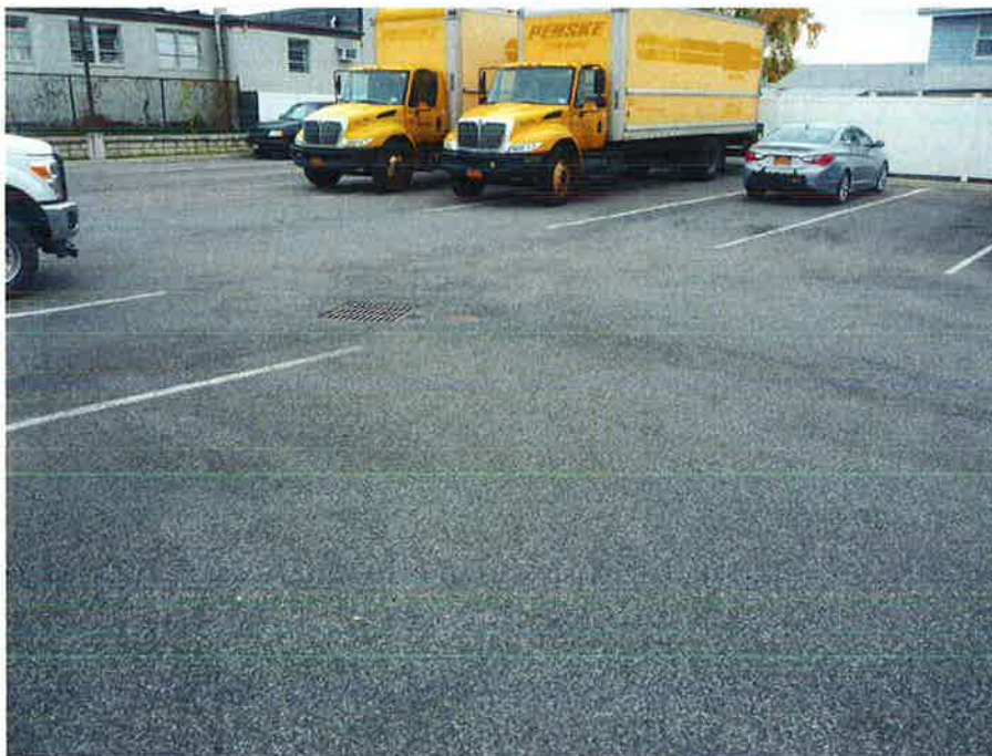
Photograph 12: Stormwater catch basin at 441 Waverly Avenue in excellent condition.
