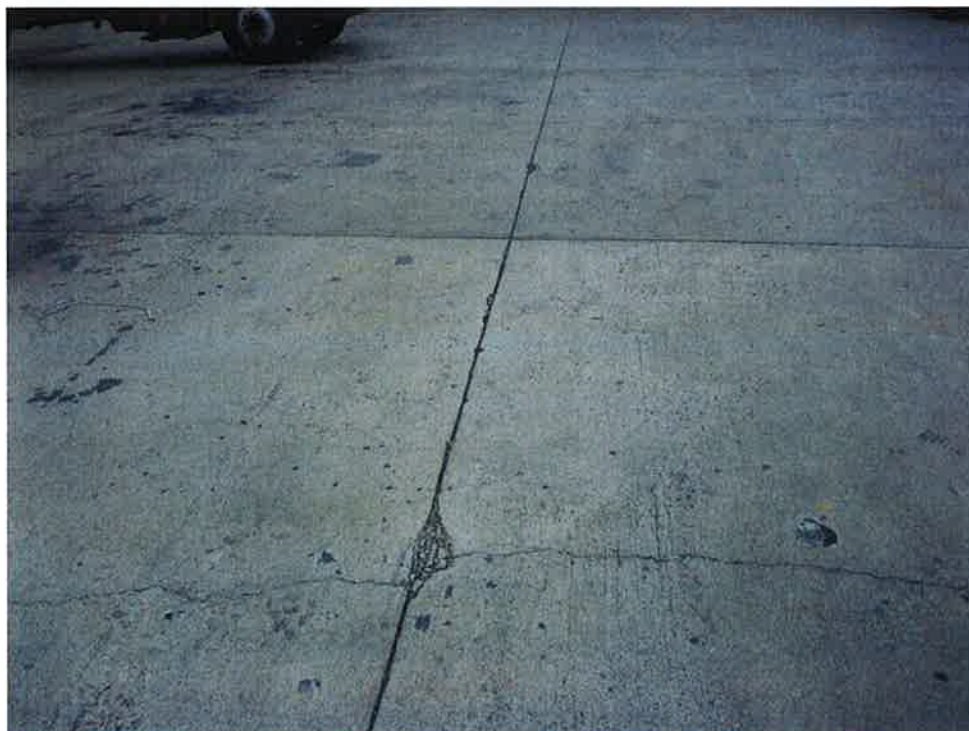
Photograph 6: Minor cracks observed in concrete on western portion of 441 Waverly Avenue.
