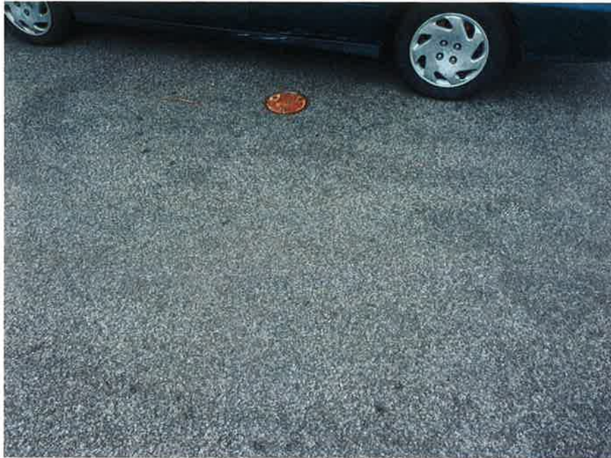
Photograph 1: Surrounding asphalt of GZ-21D in excellent condition.
