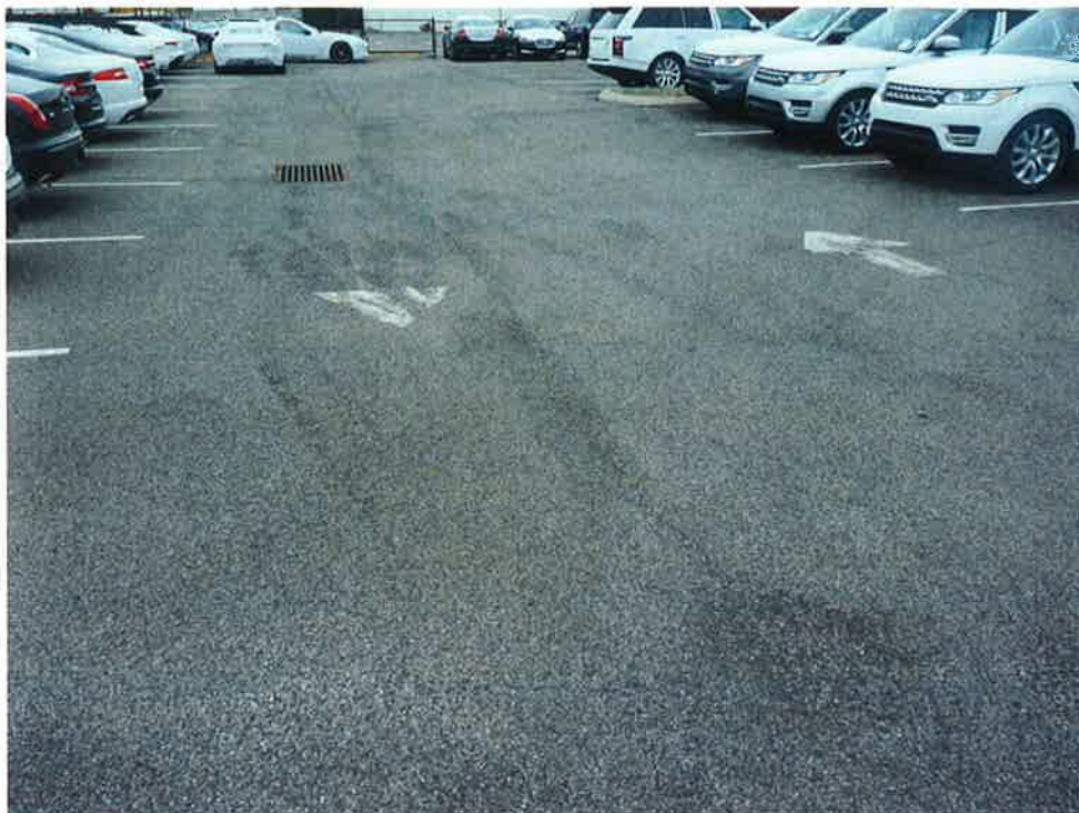
Photograph 5: Asphalt and stormwater catch basin in excellent condition at 524 Waverly Avenue.
