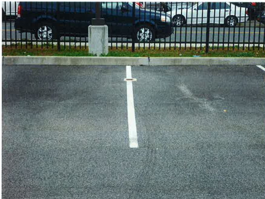
Photograph 2: Surrounding asphalt of OSMW-3 in excellent condition.
