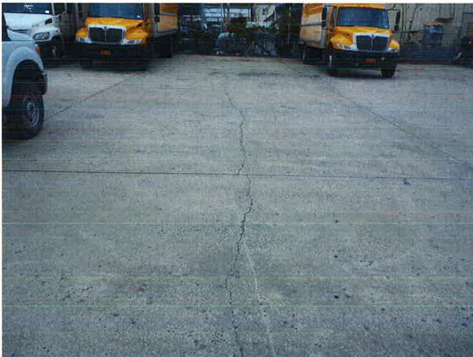
Photograph 8: Additional minor cracks observed in concrete surface of 441 Waverly Avenue.
