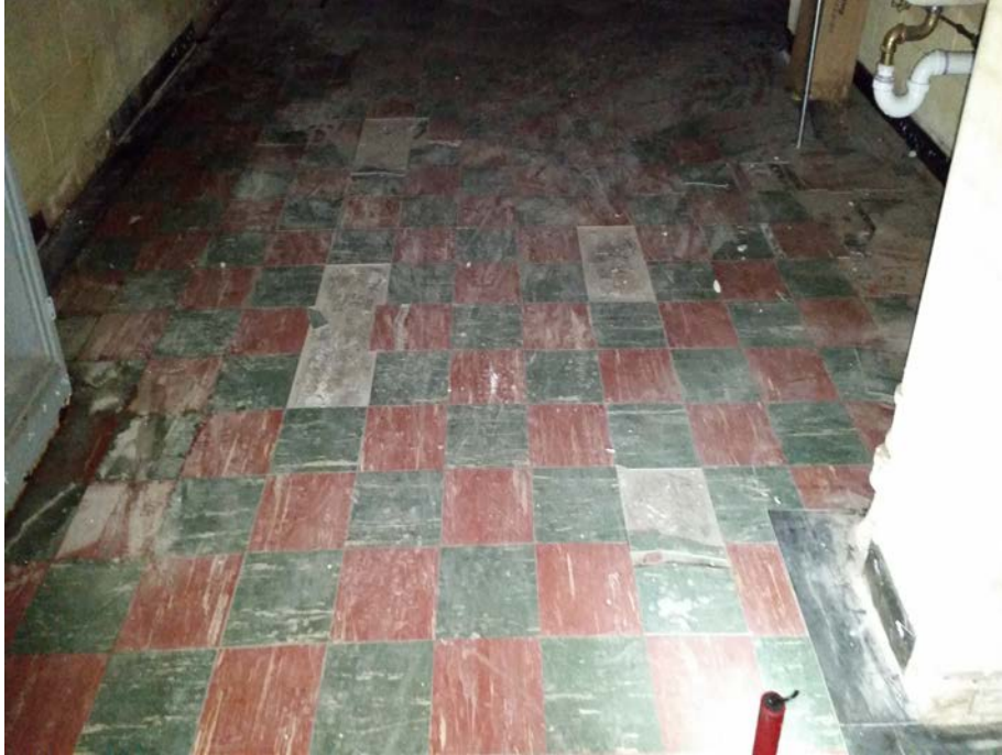
Photograph 9: Tile floor of 441 Waverly Avenue basement looking southeast towards Waverly Avenue from the stairwell. Some tiles are observed to be missing, but no penetrations observed in slab.
