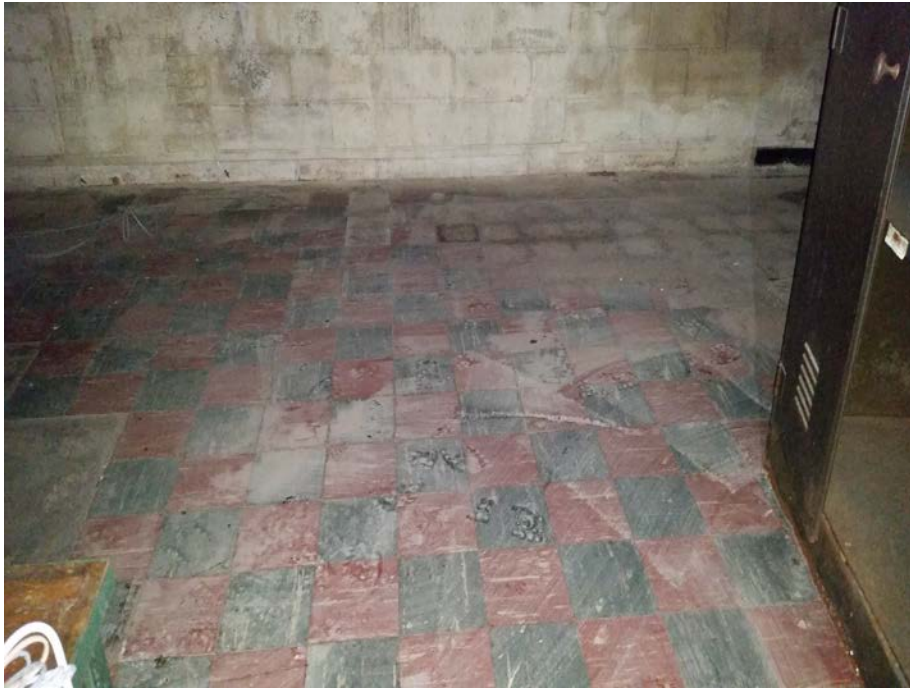
Photograph 11: Tile floor of 441 Waverly Avenue basement looking southeast towards Waverly Avenue from the stairwell. Some tiles are observed to be missing, but no penetrations observed in slab.
