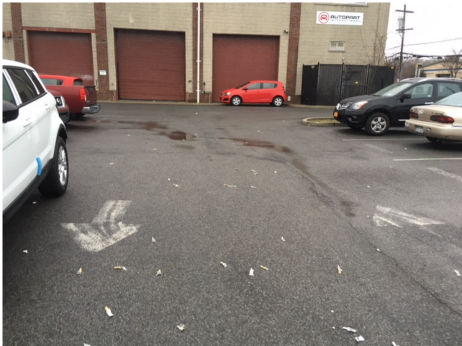
Photograph 2: Asphalt cover in parking lot of 524 Waverly Avenue is in good condition with no evidence of significant cracks, potholes, or other penetrations.
