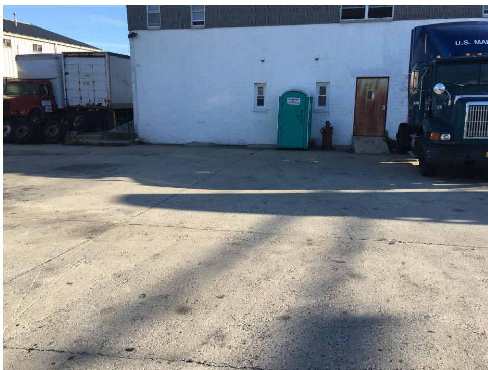
Photograph 8: Concrete surface of the western lot of 441 Waverly Avenue was observed to have minor cracks, but still acceptable (looking south to north).
