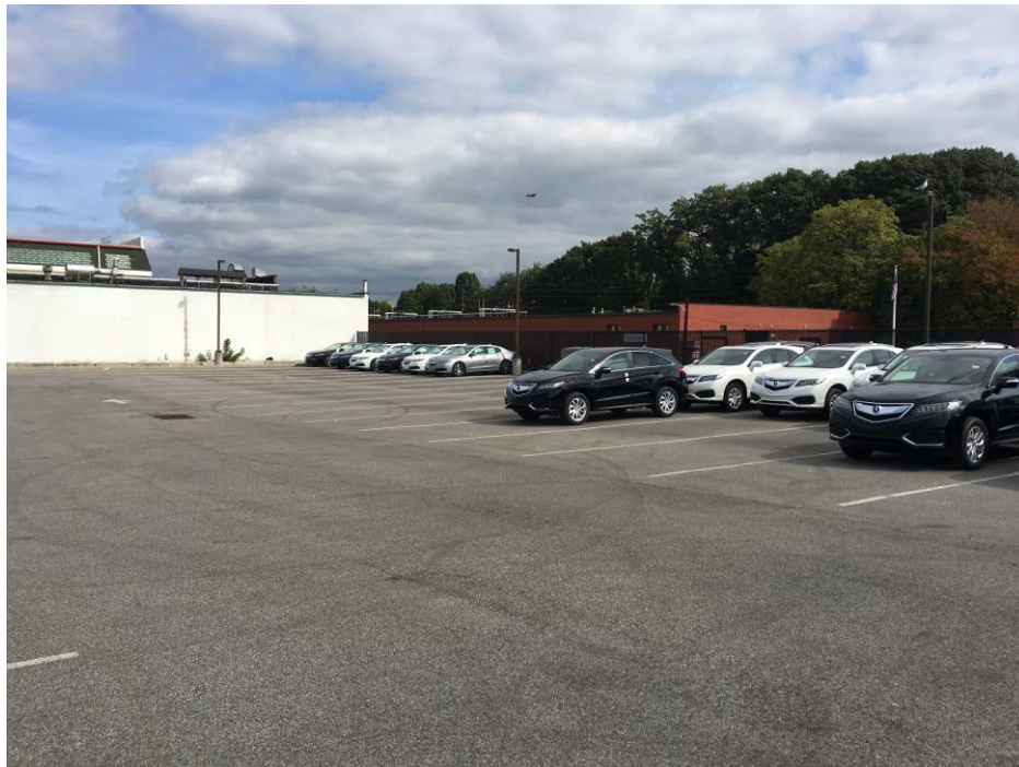
Photograph 4: Pavement across 442 Waverly Avenue is in great condition with no evidence of penetrations or cracks (looking west to east).
