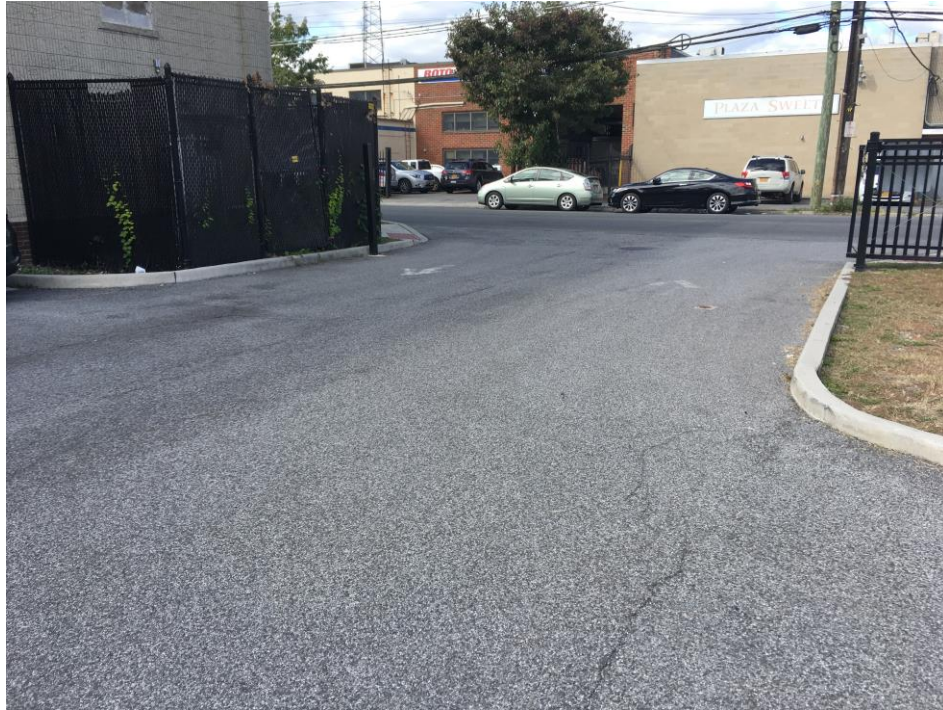
Photograph 1: Entrance/exit ramp of 524 Waverly Avenue is in great condition with no evidence of penetrations or major cracks (looking east to west).
