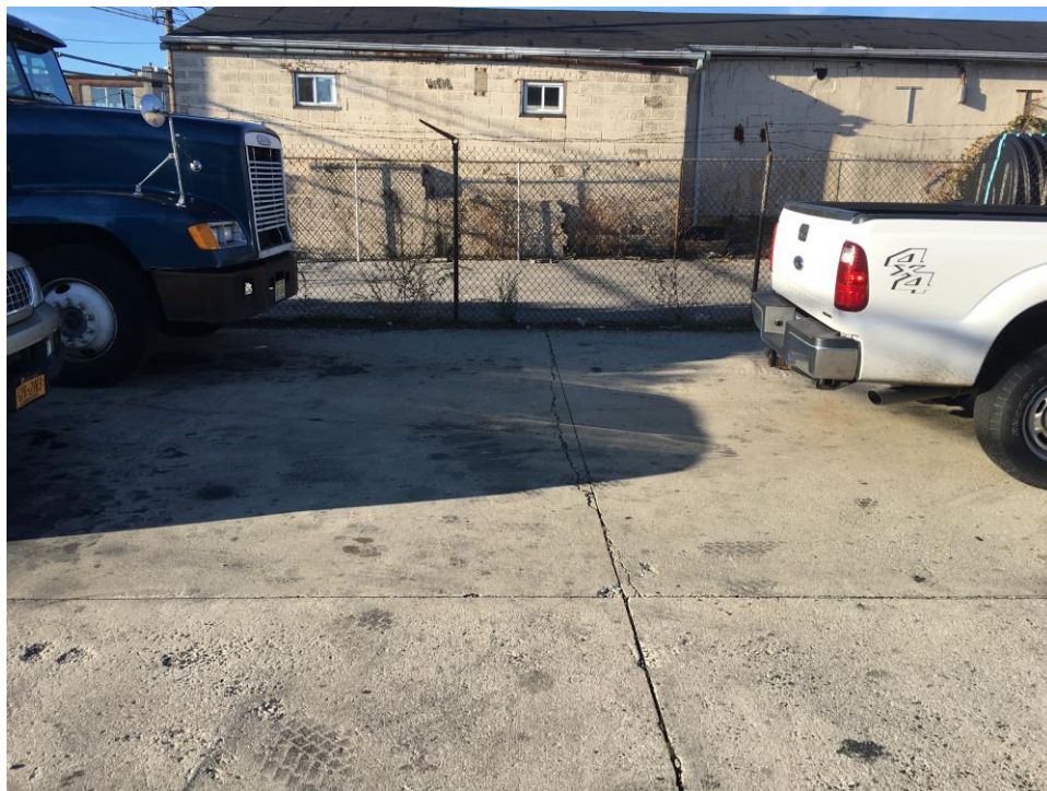
Photograph 7: Concrete surface of the western lot of 441 Waverly Avenue was observed to have minor cracks, but still acceptable (looking northeast to southwest).
