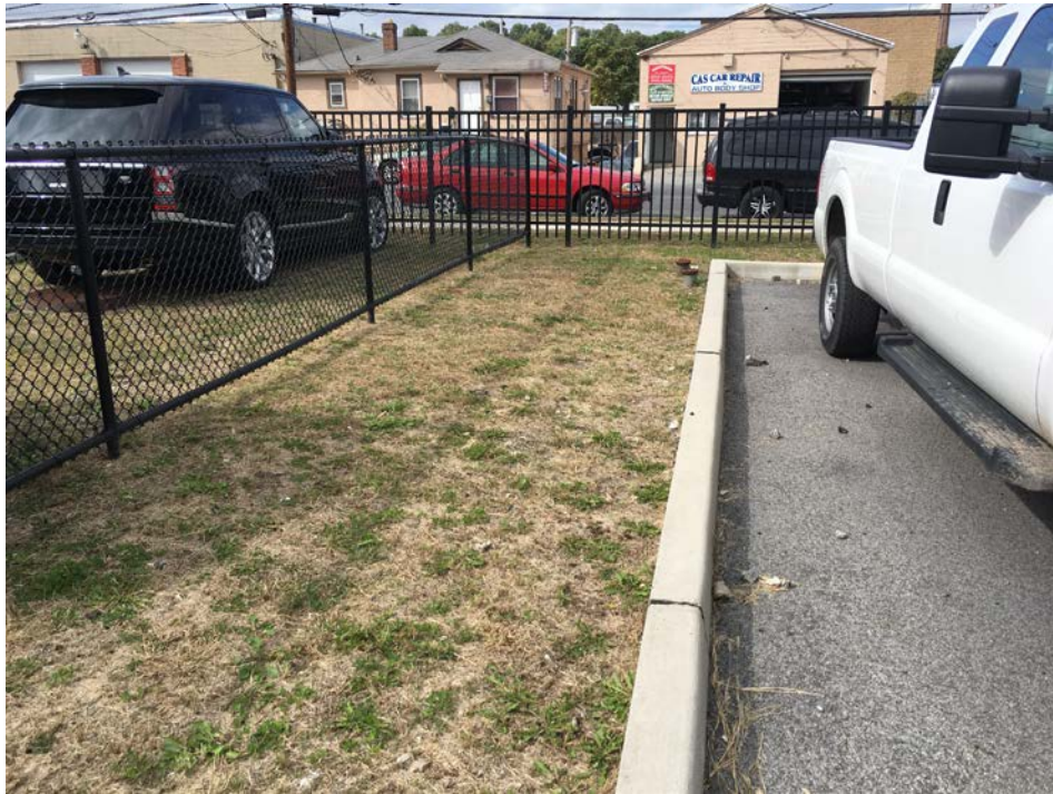
Photograph 3: Curbed lighting areas and retaining walls are in good condition with no evidence of erosion or cracks (Well GZ-23D, looking southeast to northwest).
