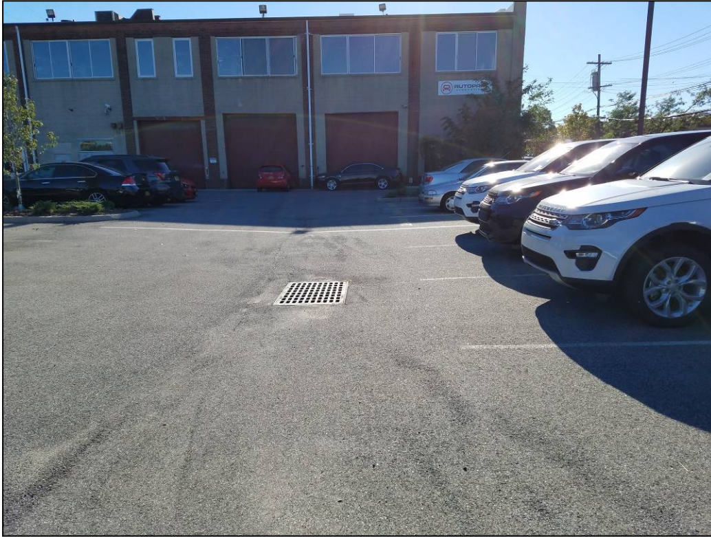
Photograph 5: Curbed areas and asphalt cover system are in good condition with no evidence of erosion or cracks.
