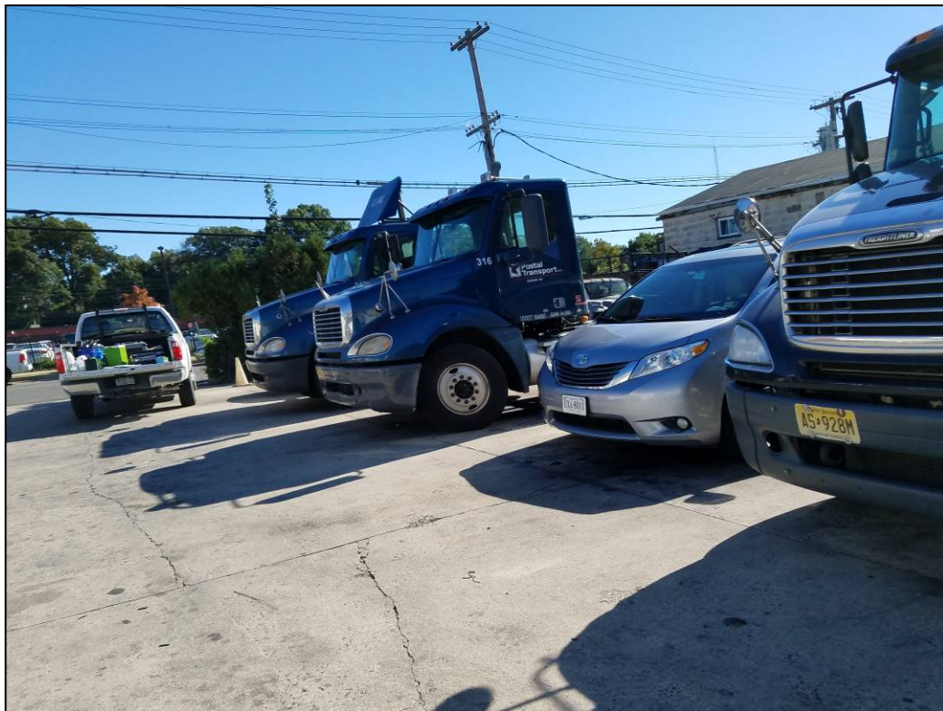
Photograph 2: Onsite pavement is in fair condition with no evidence of penetrations or major cracks. Some minor cracks in pavement observed.
