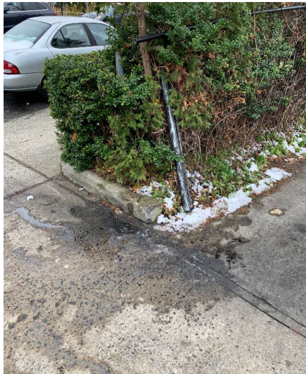
Photograph 5: Minor damage to the perimeter fence at 441 Waverly Avenue. Curbs and concrete cover are in acceptable condition with no observed damage or large cracks, looking south.
