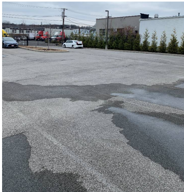
Photograph 4: Onsite asphalt at 442 Waverly Avenue is in good condition with no evidence of penetrations or large cracks, looking north-northwest.
