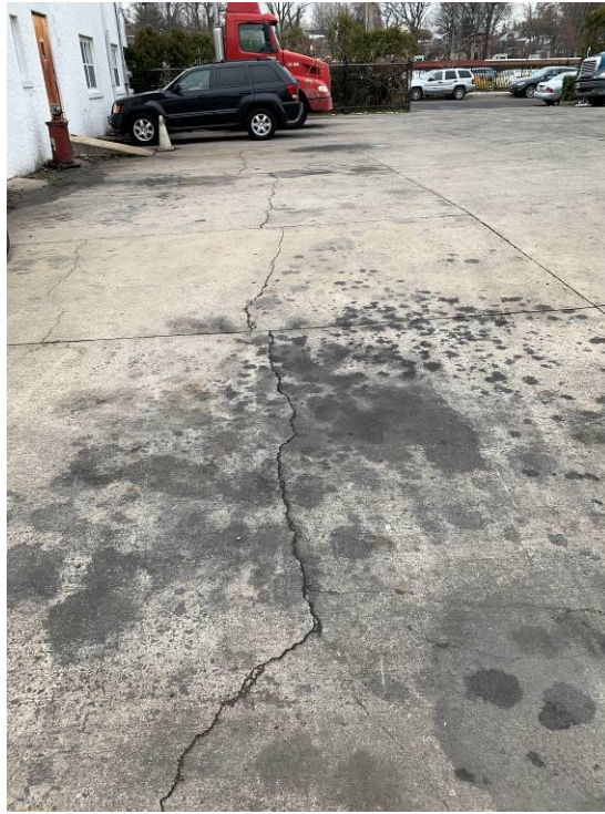
Photograph 1: View of concrete cover system at 441 Waverly Avenue in good condition with some cracks wider than 1/4-inch that should be monitored, looking southwest.
