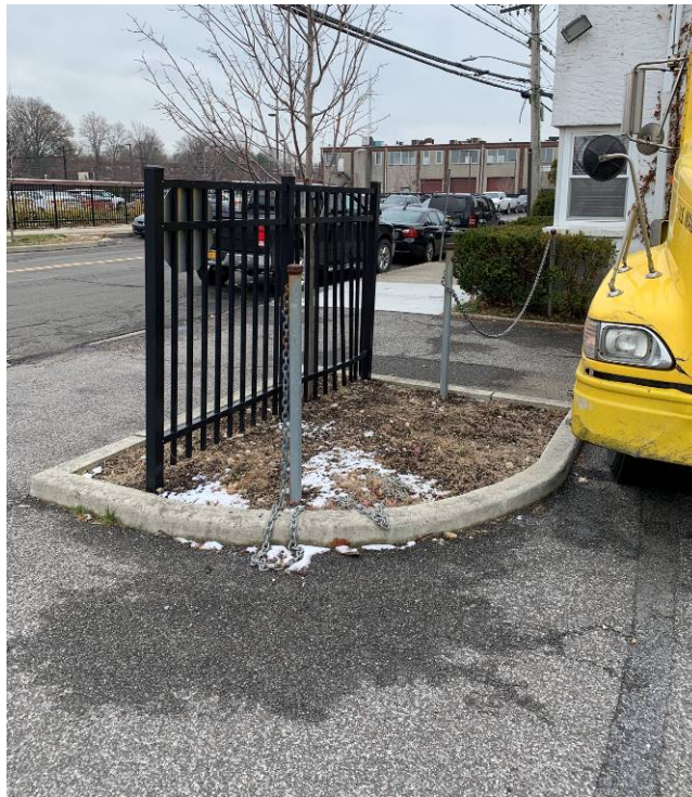
Photograph 3: Curbed areas and asphalt cover system at 441 Waverly Avenue in good condition with no evidence of damage or large cracks, looking south.
